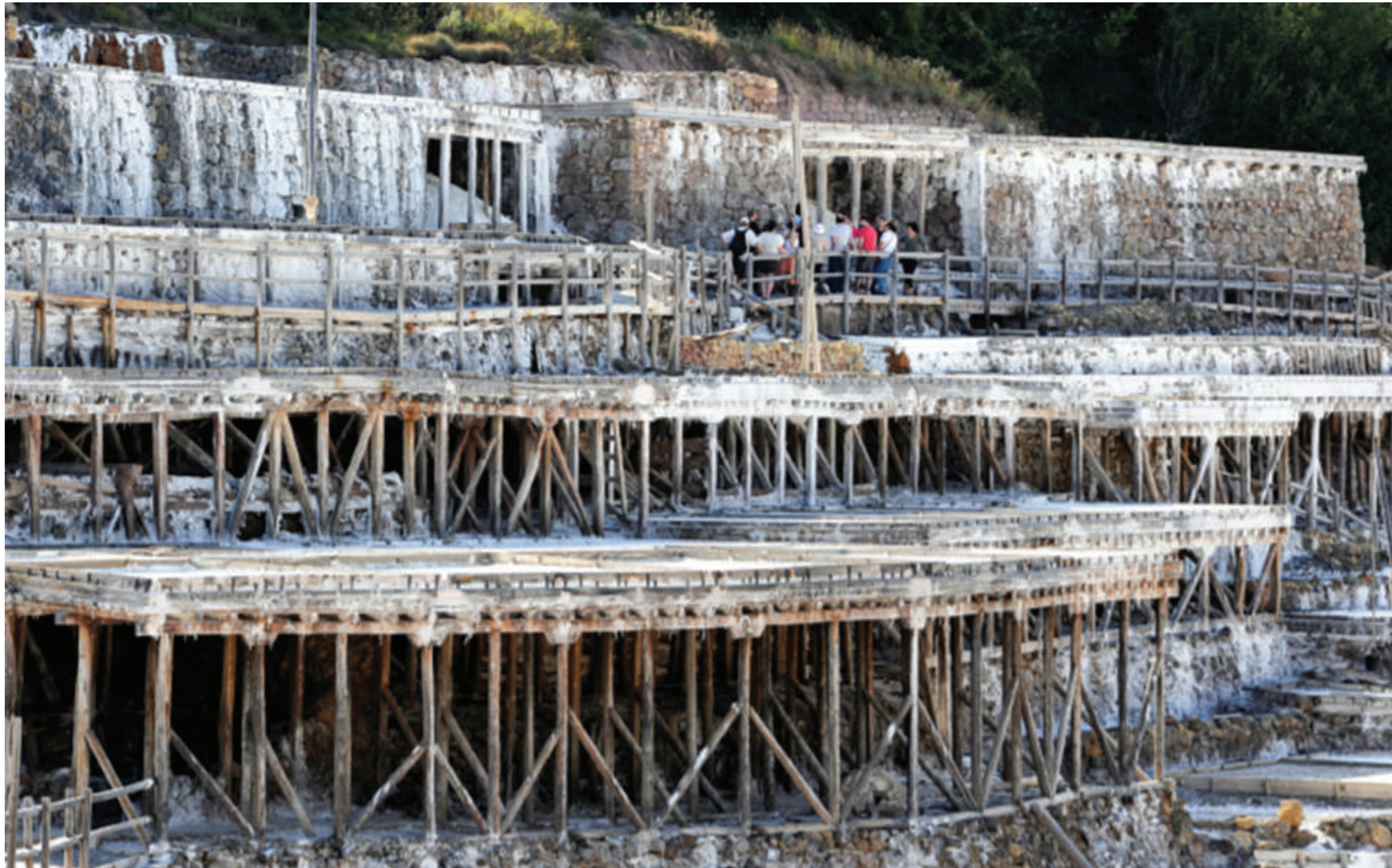
Fig.3: View of the different levels of threshing floors, wooden construction, and stone retaining walls.
