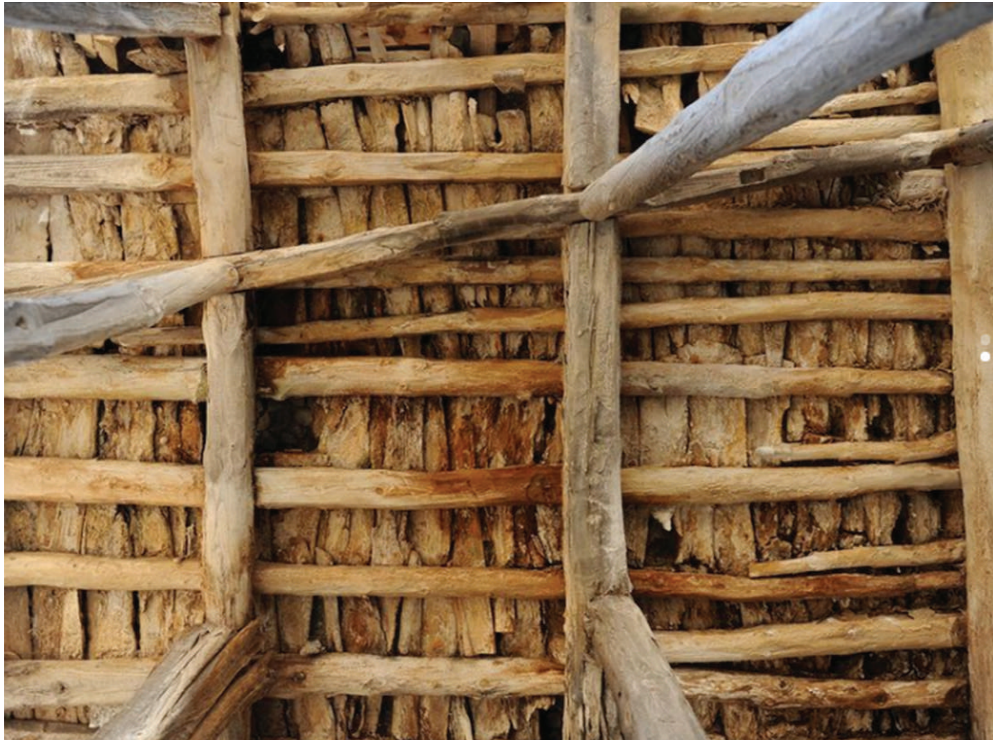
Fig.4: View of the wooden under structure that supports the threshing floors.
