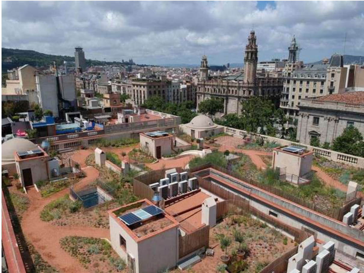
Fig.3: View of the recently finished rooftop. © MataAlta Studio
