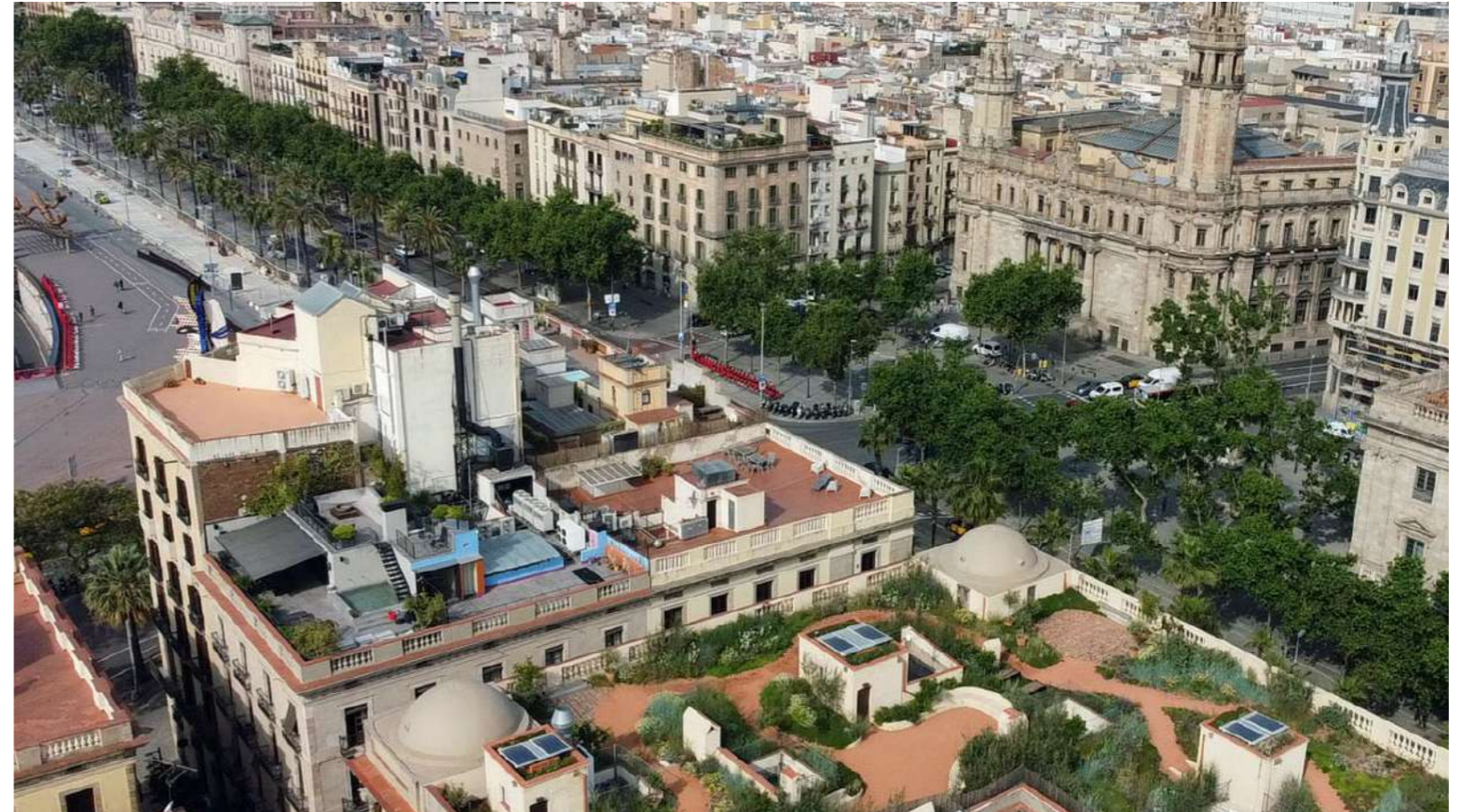
Fig.4: Aerial view of the recently terrace and its surroundings. © MataAlta Studio
