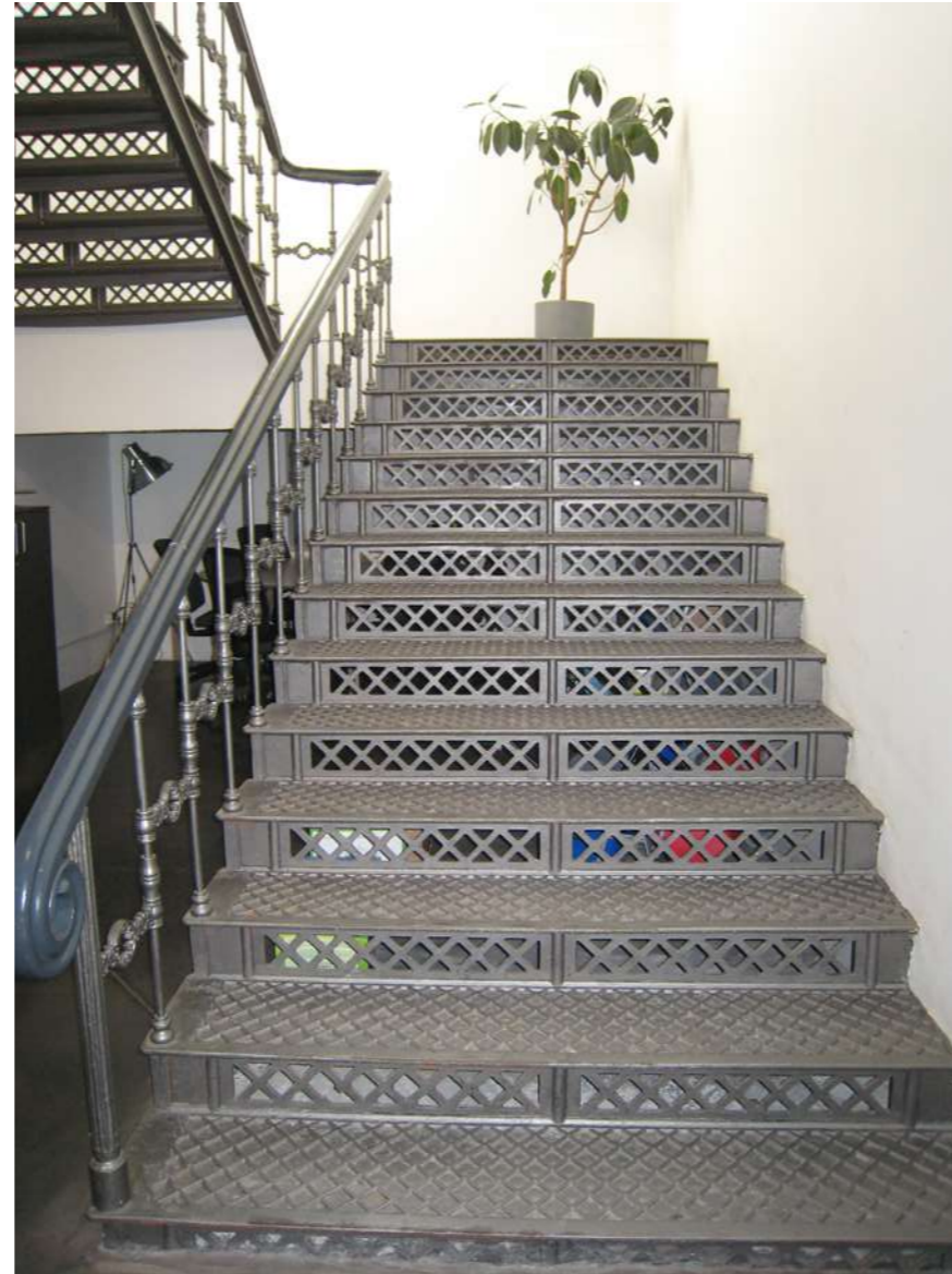
Fig.25: Restored old stairs.
