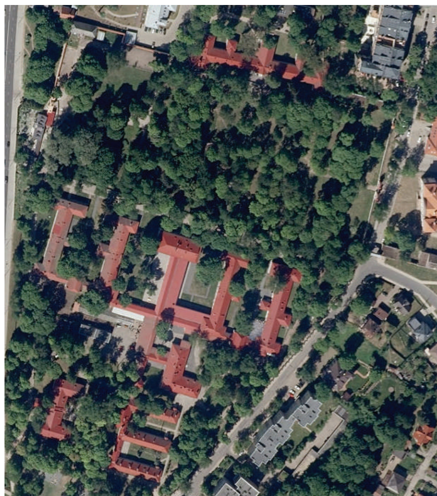
Fig.2: Bird's eye view of the complex.
