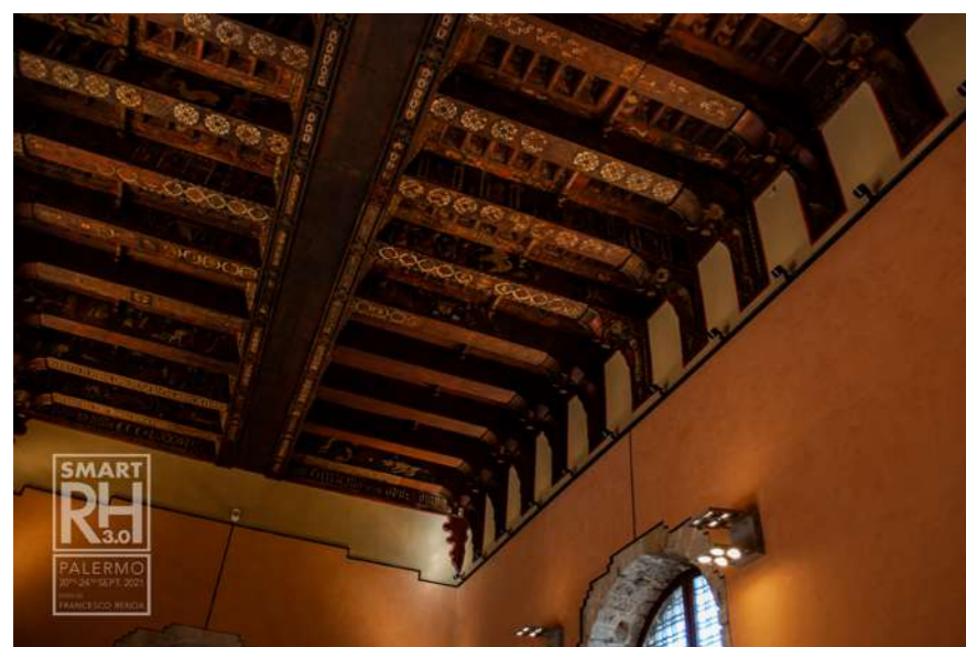
Fig.6: General view of the wooden ceiling, from below. ©Francesco Renda
