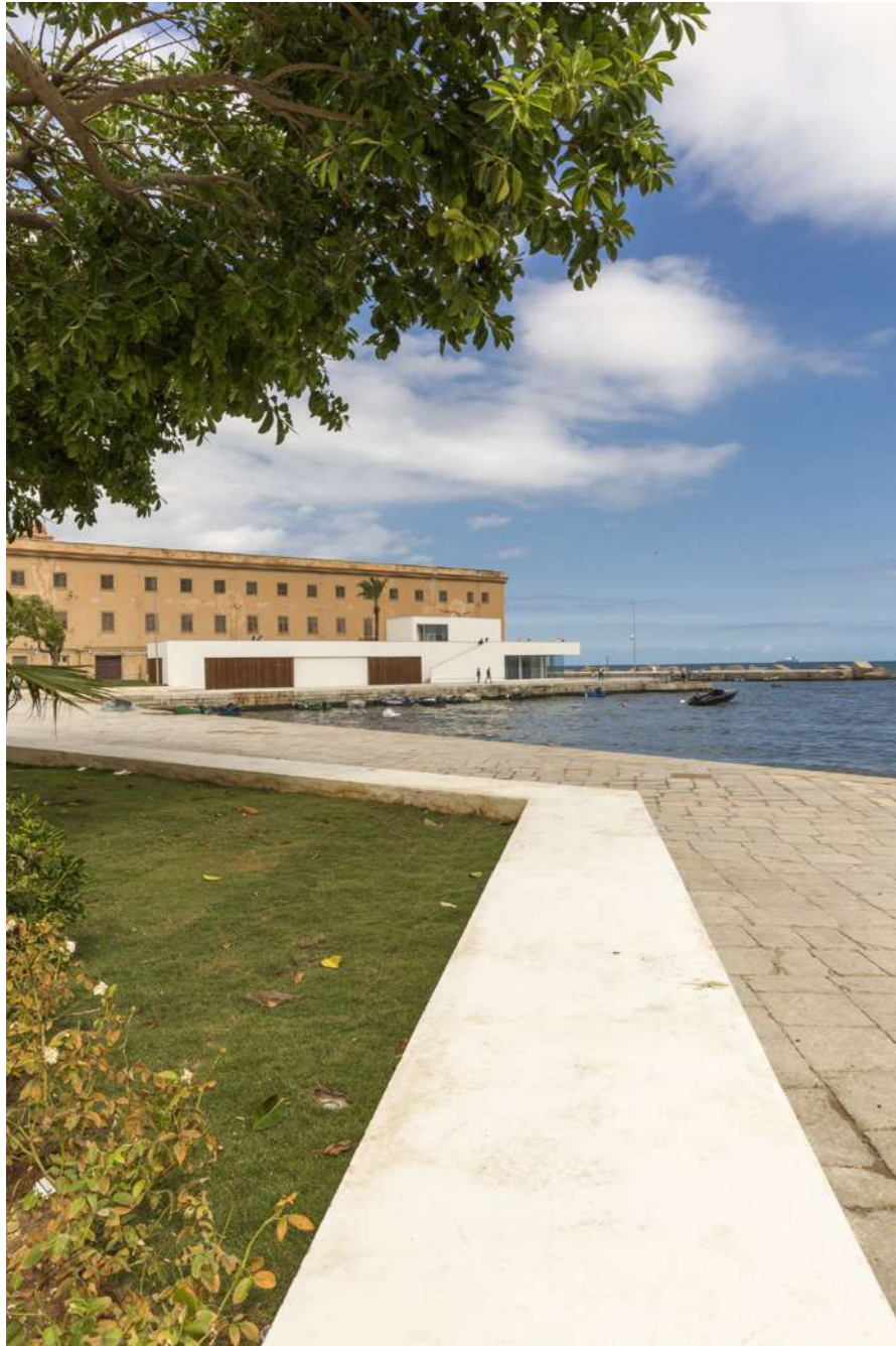
Fig.5-6: The pier after the intervention. © Provenzano Architects
