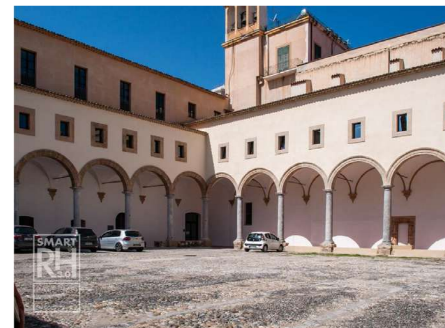
Fig.3: View of the internal courtyard and portico. ©Francesco Renda
