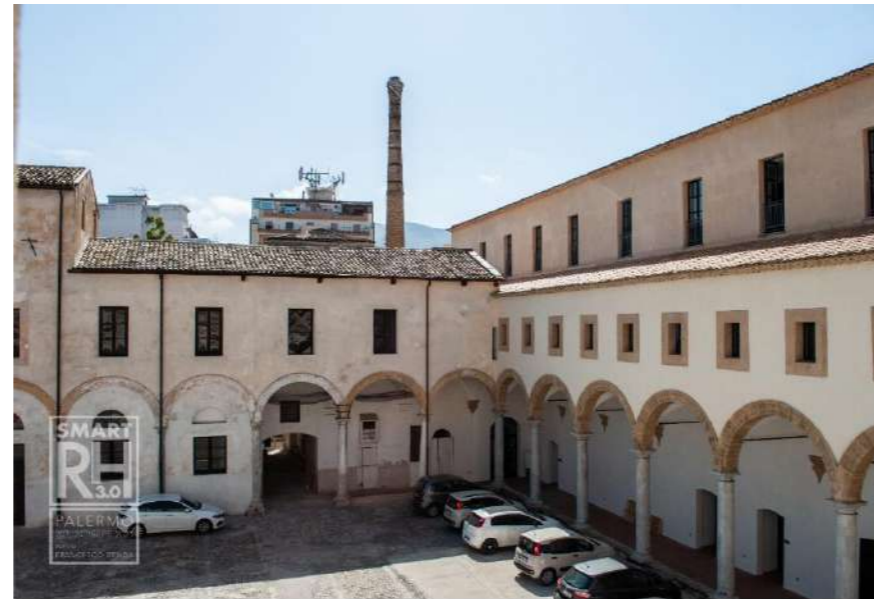
Fig.22: View of the chimney of the Military Mill. ©Francesco Renda
