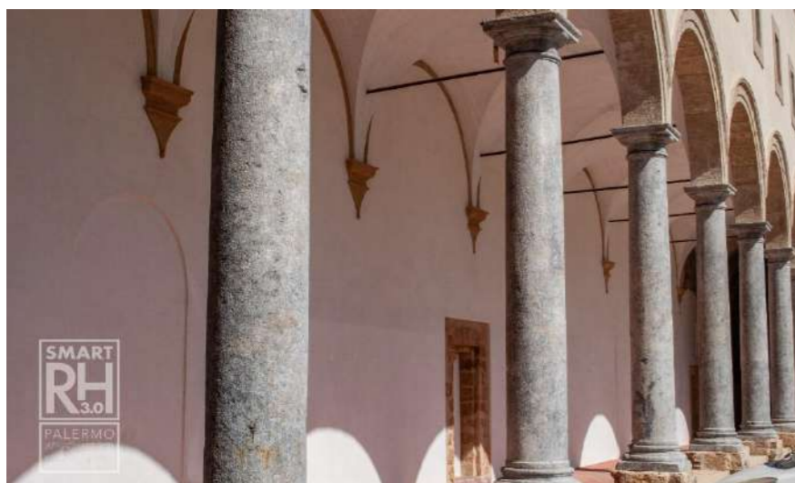
Fig.5: Detail view of one of the arms of the inner portico with columns of compact grey limestone and shell limestone arches. ©Francesco Renda
