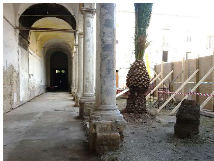
Fig.6a: Detail view of one of the arms of the inner portico with stone cross vaults, set on corbels and metal chains to eliminate horizontal actions, before the interventions. © University of Palermo, Technical Area
