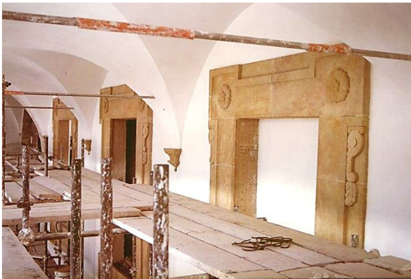
Fig.14: Restoration of the openings in on sight stone of the convent portico. © Municipality of Palermo, Historical Center Technical Area
