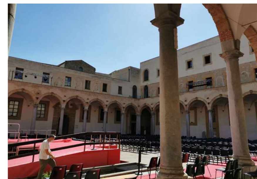
Fig.33: The courtyard itself, with a detail of the stage intended for concrete, equipped with ramps. The restoration project took care of in detail all aspects relating to extended accessibility. © Luisa Lombardo
