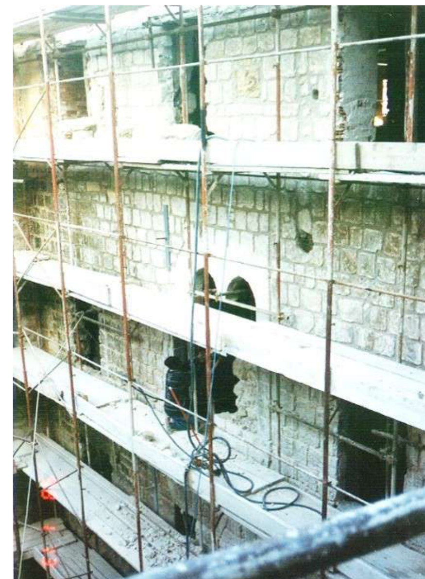
Fig.3a-b: Pre-consolidation and cleaning works, as well as freeing up closed openings. © Municipality of Palermo, Historical Center Technical Area
