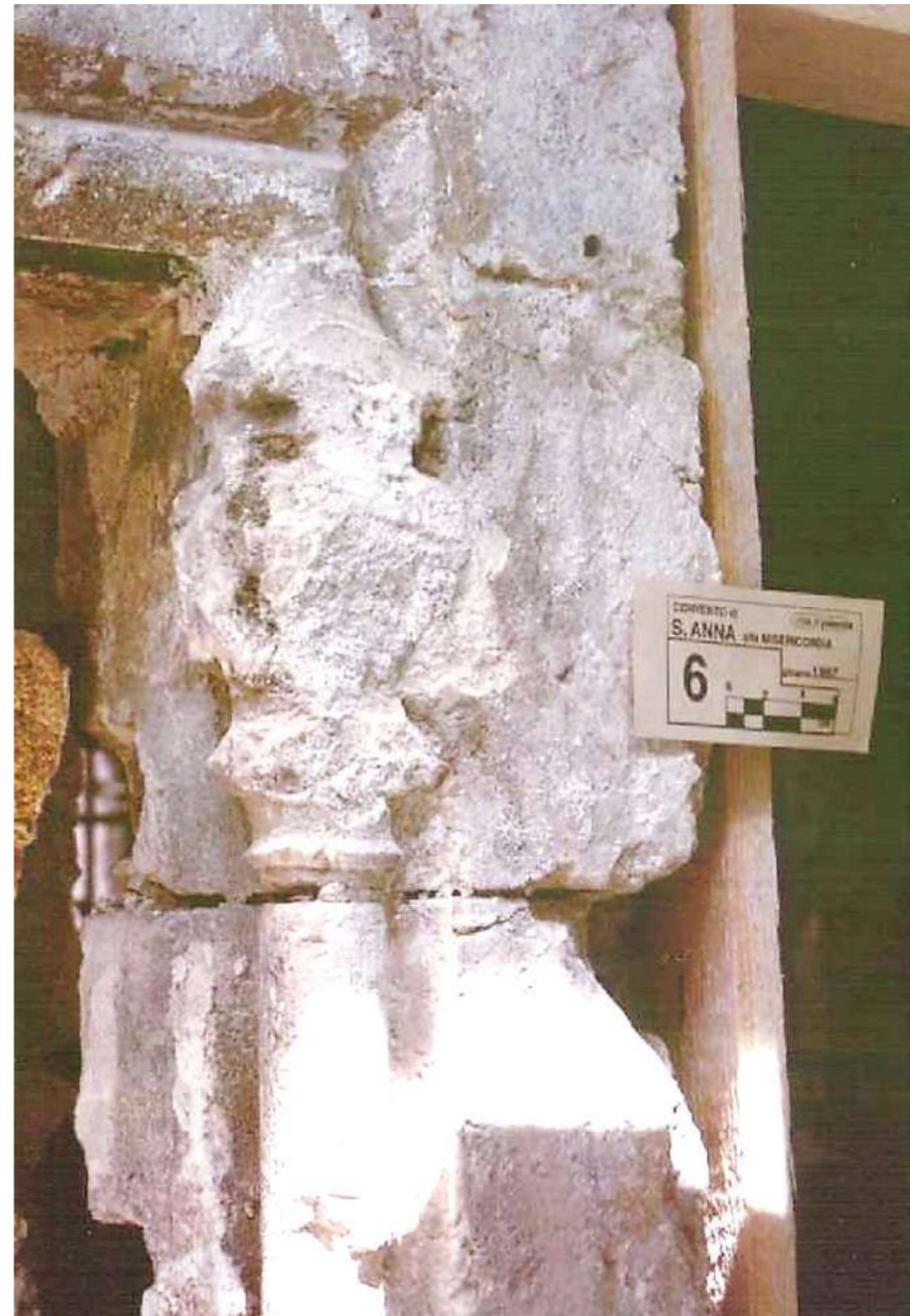
Fig.6a-b: Securing work on a reopened mullioned window and appearance of the "Catalan-style" cornices that have been chipped to hide them over time. © Municipality of Palermo, Historical Center Technical Area
