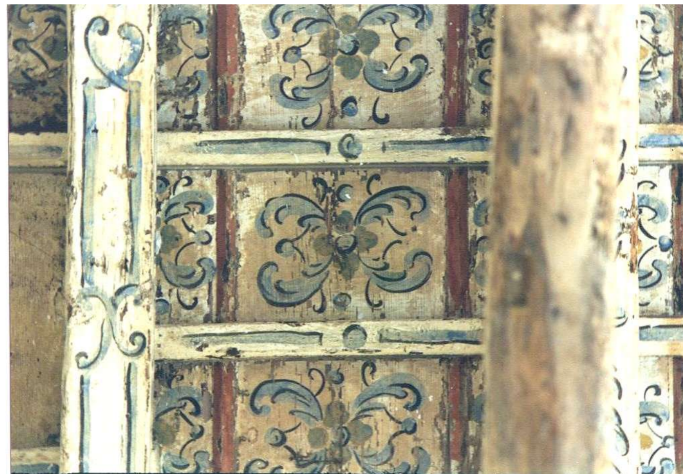
Fig.15: Tempera painted wooden floor, before restoration works. © Municipality of Palermo, Historical Center Technical Area
