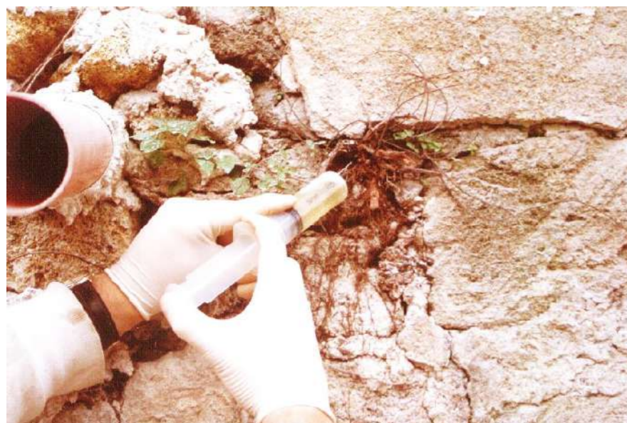
Fig.4: Disinfestation intervention through the application of herbicide. © Municipality of Palermo, Historical Center Technical Area
