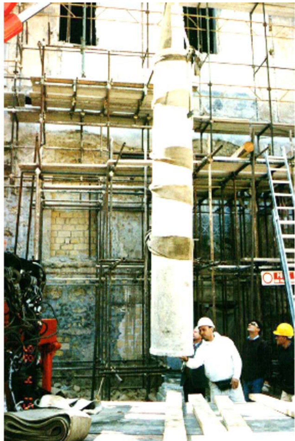
Fig.18: Relocation of old and new columns and capitals of compact limestone. © Municipality of Palermo, Historical Center Technical Area
