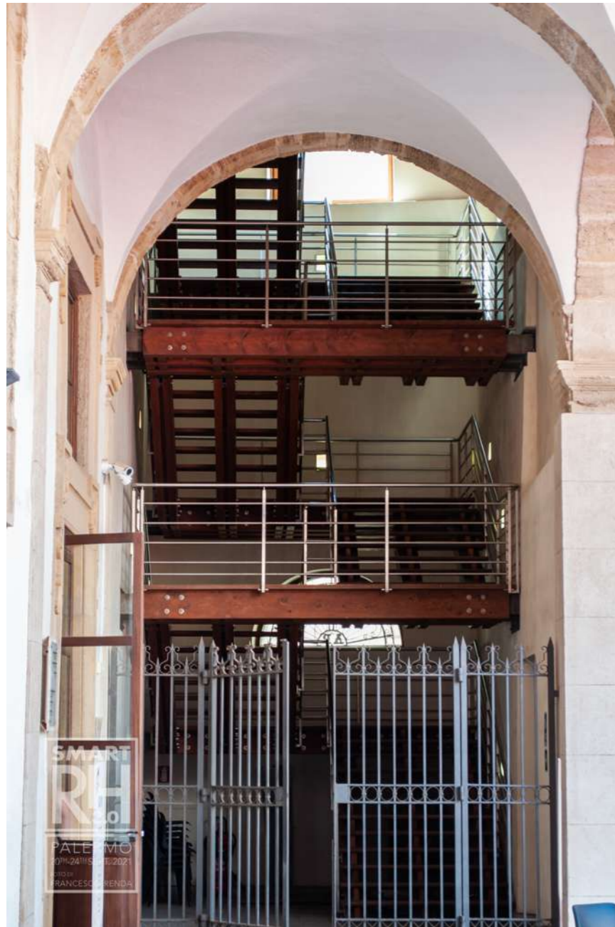
Fig.30a-b: Creation of a new security staircase and integrated services (lightning and air conditioning systems) in correspondence of wooden trusses. © Francesco Renda & Luisa Lombardo
