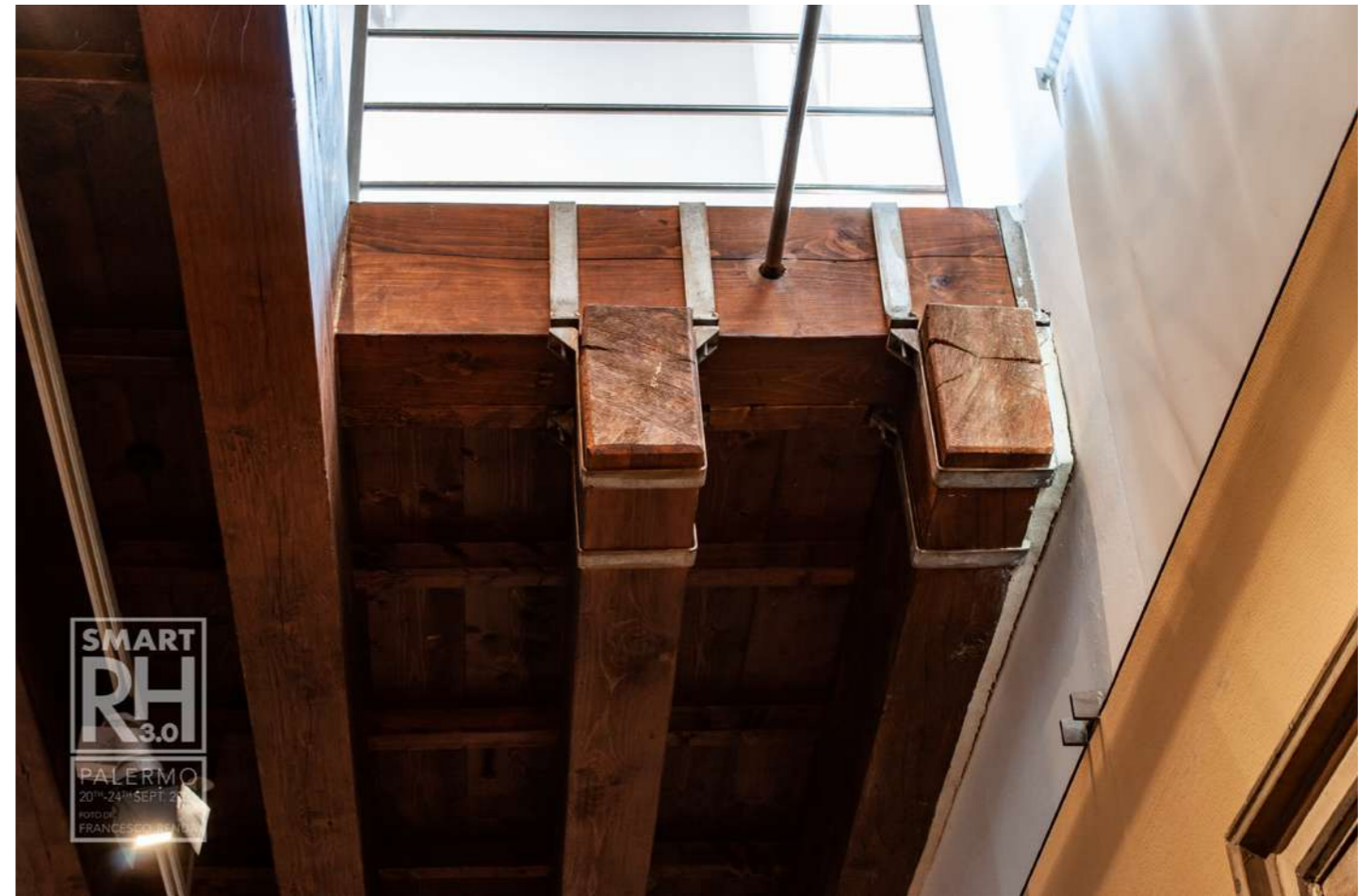
Fig.27: Consolidation intervention on a wooden floor, useful to the creation of an inside hollow space. © Francesco Renda
