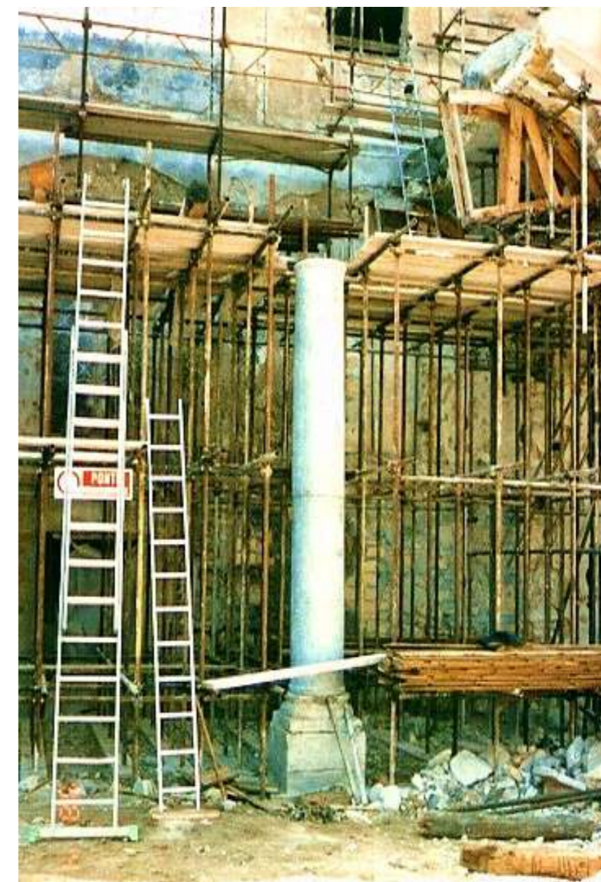
Fig.17a-b: Collapse of an arm of the porch of the convent, following a mafia attack and start of the reconstruction and restoration works: relocation of old and new columns of compact limestone. © Municipality of Palermo, Historical Center Technical Area
