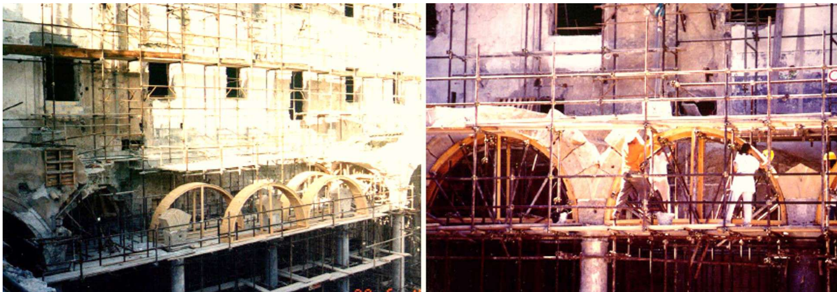
Fig.19: Collapse of an arm of the porch of the convent, following a mafia attack and start of the reconstruction and restoration works: reconstruction of stony arches. © Municipality of Palermo, Historical Center Technical Area
