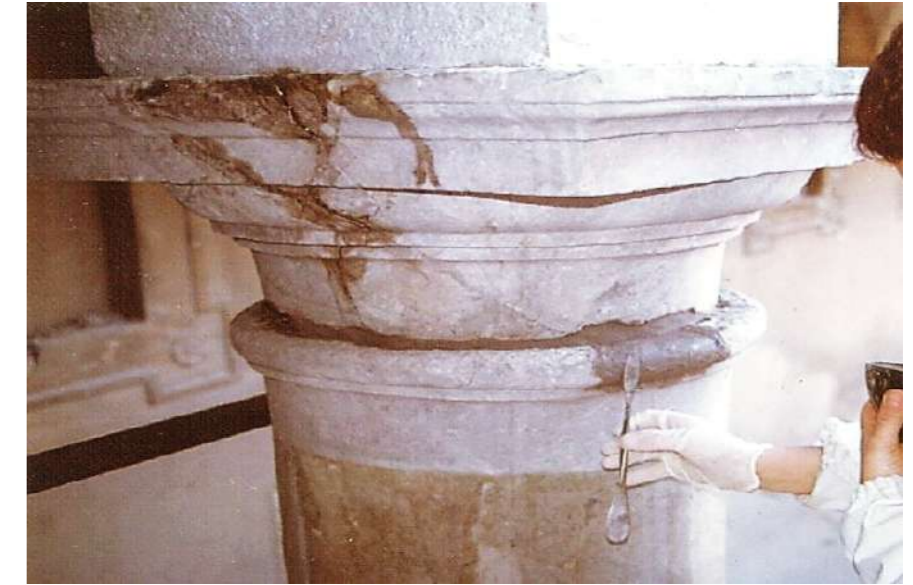
Fig.12: Cleaning and plastering work on one of the columns of the portico, in compact gray limestone. © Municipality of Palermo, Historical Center Technical Area
