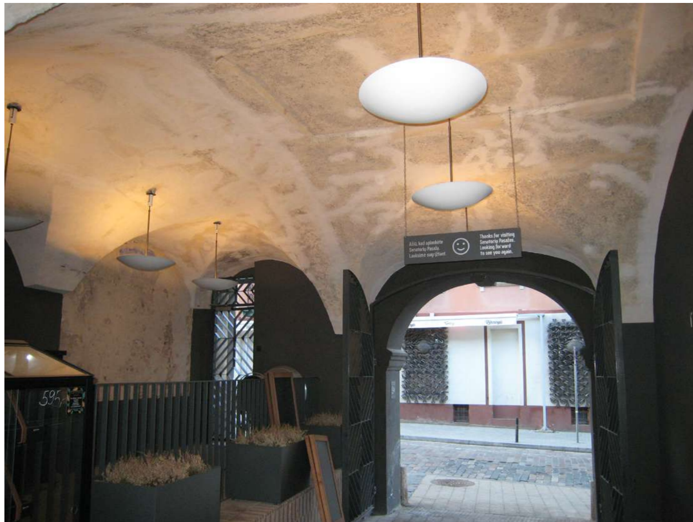
Fig.19: Passage to the yard.
