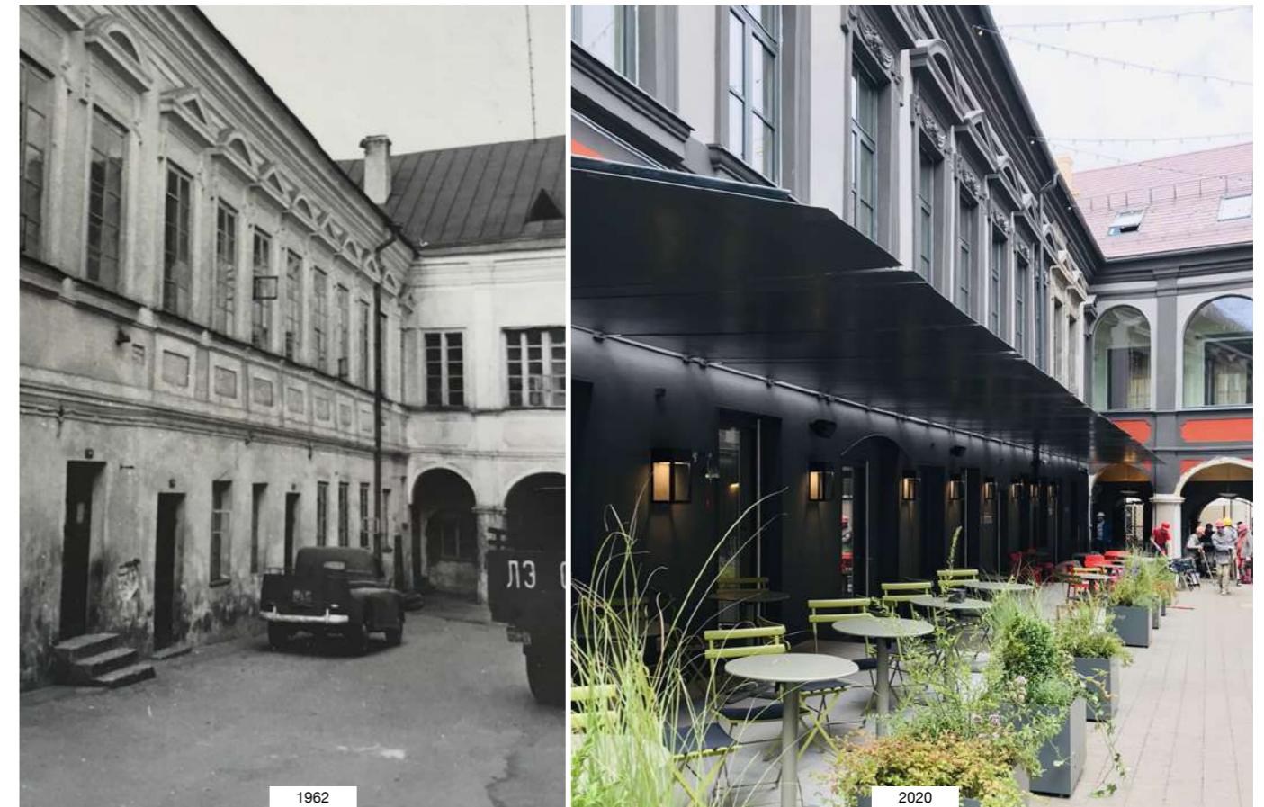
Fig.15: Courtyard facade before and after reconstruction.
