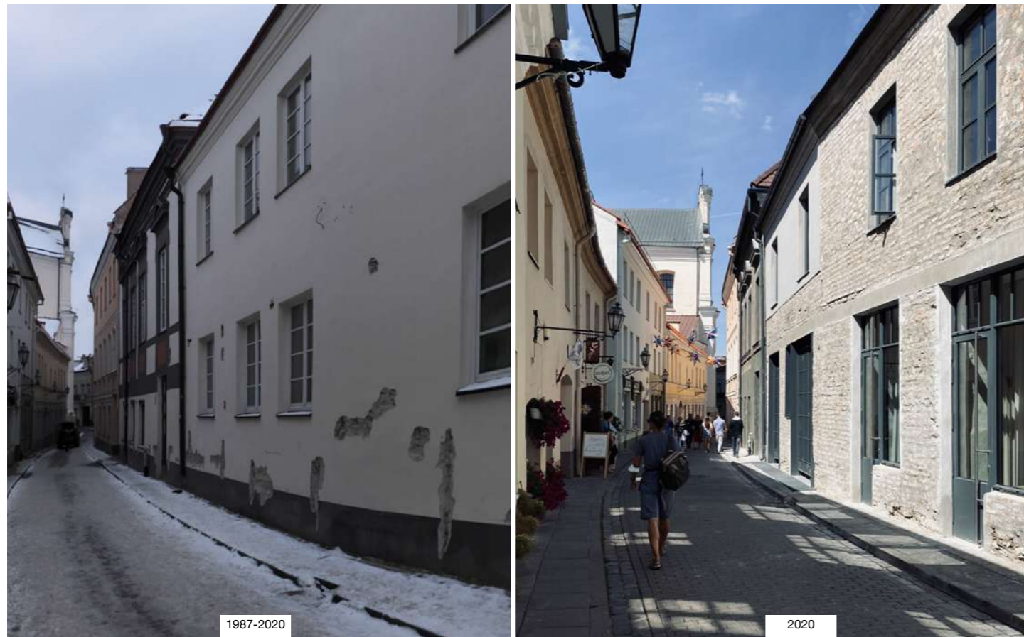
Fig.14: Street facade before and after reconstruction.
