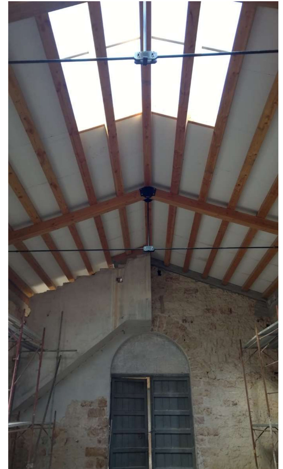
Fig.15: The tavern during the construction phase. © Arch.Chiera Mazarella
