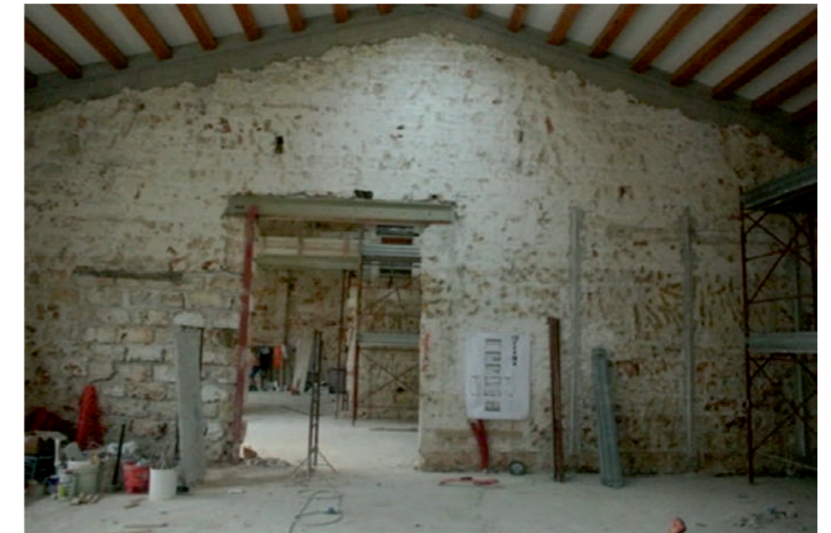
Fig.20: The furnace during the construction phase. © Arch.Chiara Mazzarella
