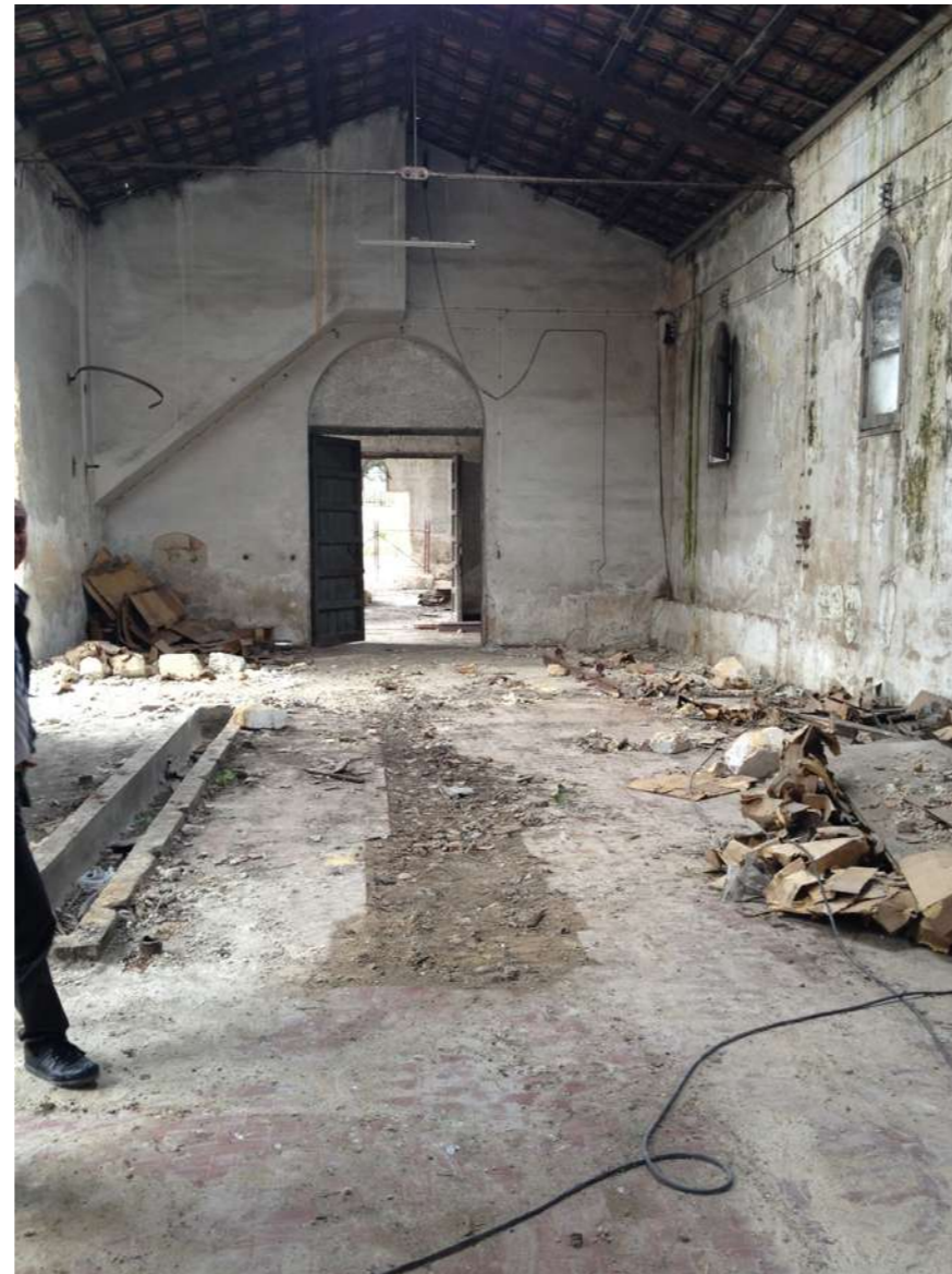
Fig.22: The Vinery during the construction phase. © Arch.Chiara Mazzarella
