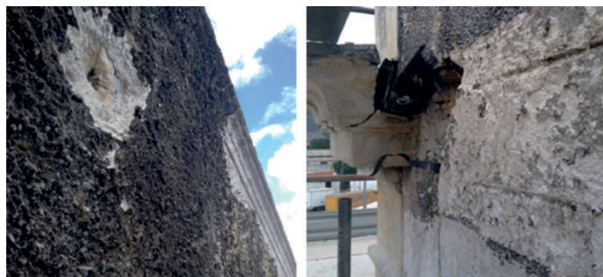
Fig.9a-b: Detail of the rustic cement-based plaster and sting course before cleaning and reinforcement intervention. © Arch.Chiara Mazzarella
