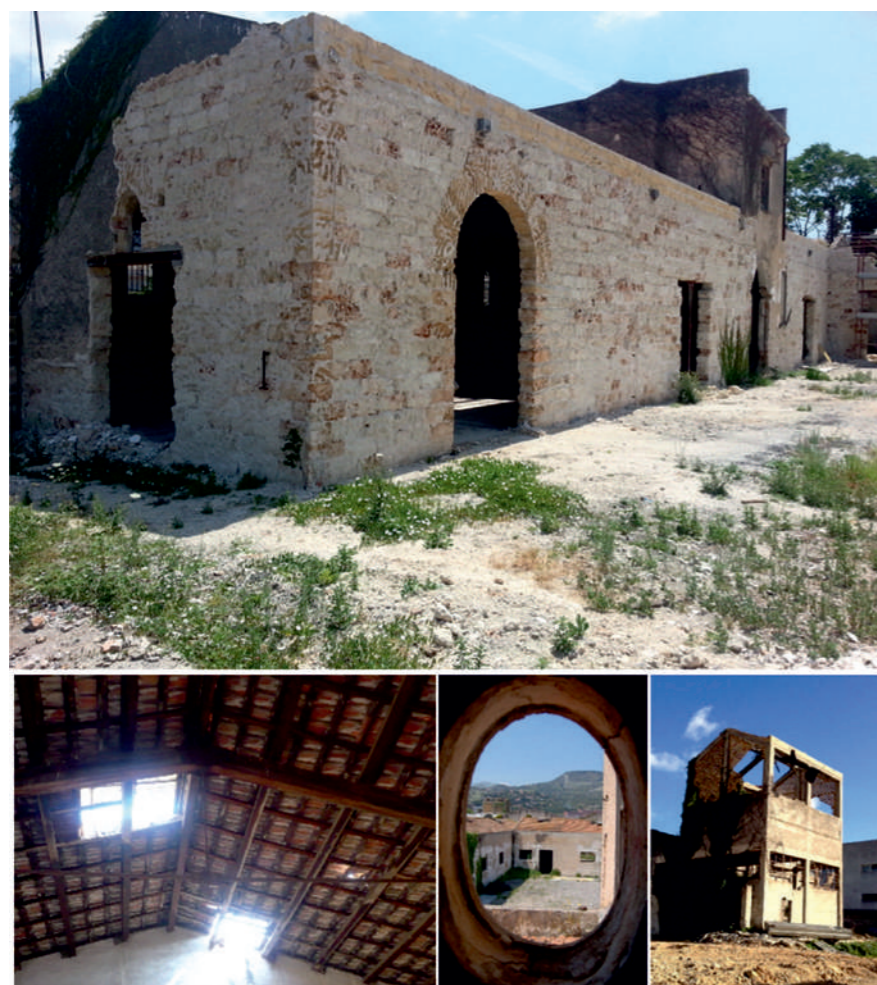
Fig.3: Views of the original state. © Arch. Chiara Mazzarella
