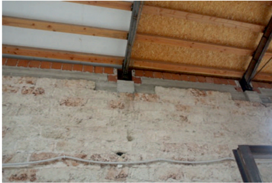
Fig.16: The tavern. Covers consolidation. © Arch.Chiara Mazzarella
