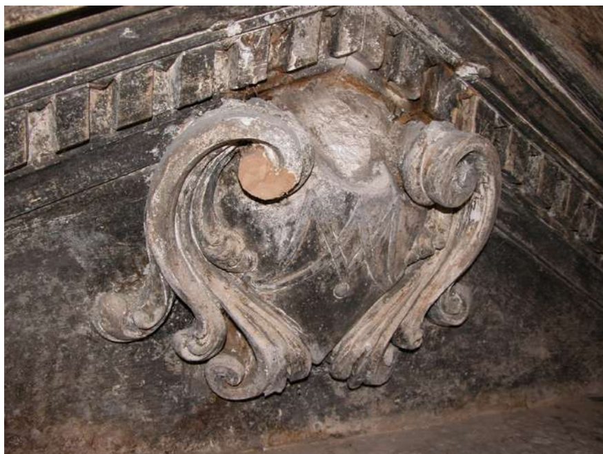
Fig.12: State of maintenance of the inner plaster and the stucco decoration of the spaces, in the picture the friezes of the chapel before the restoration works. @ Eng. Marinella Fiore
