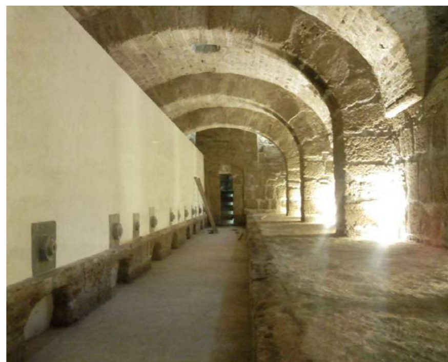
Fig.4: View of the underground level under the right nave, with masonry wine containers, after the restoration works - @ Eng. Marinella Fiore
