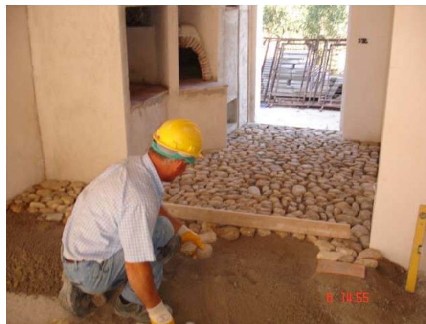
Fig.22: Reconstruction of the traditional cobblestone paving, during the restoration works. @ Eng. Marinella Fiore
