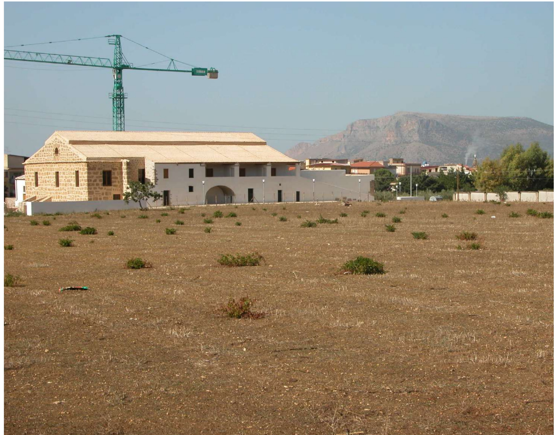
Fig.24: View of the complex during the restoration works. @ Eng. Marinella Fiore
