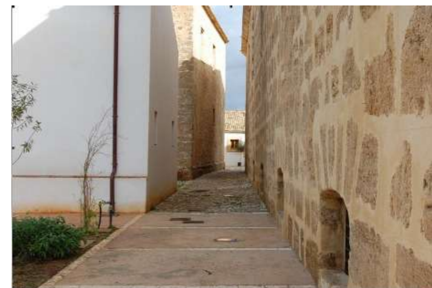
Fig.6: View of the inner spaces (passage between the cellar, the tower and the stable) and external treatment, after the restoration works. @ Eng. Marinella Fiore
