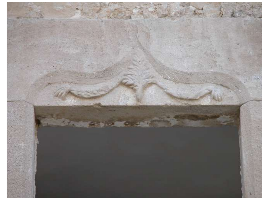
Fig.7: Architrave is adorned in Catalan style with two volutes connected in a central point. An interesting element in an industrial building, after the restoration works. @ Eng. Marinella Fiore
