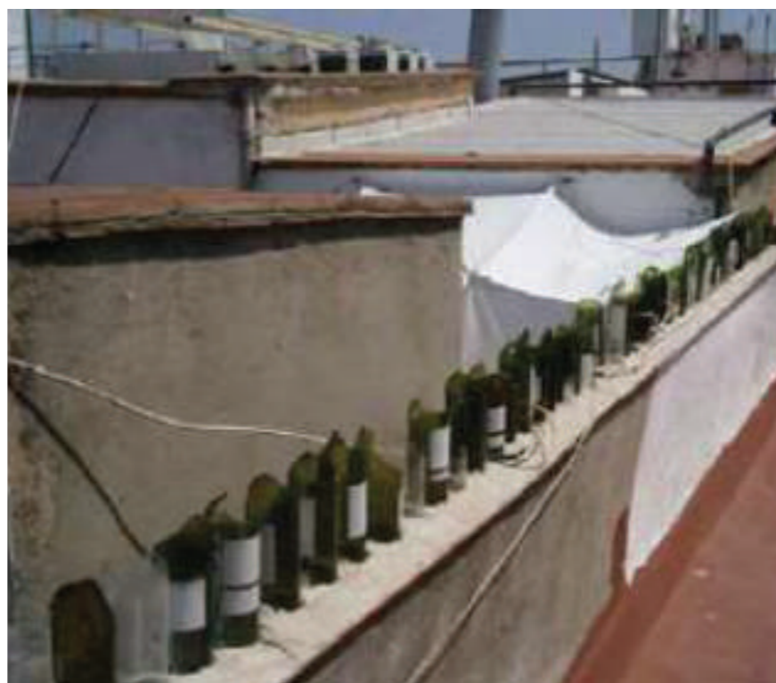
Fig.7-8: Conditions of the patio and rooftop prior to the intervention.
