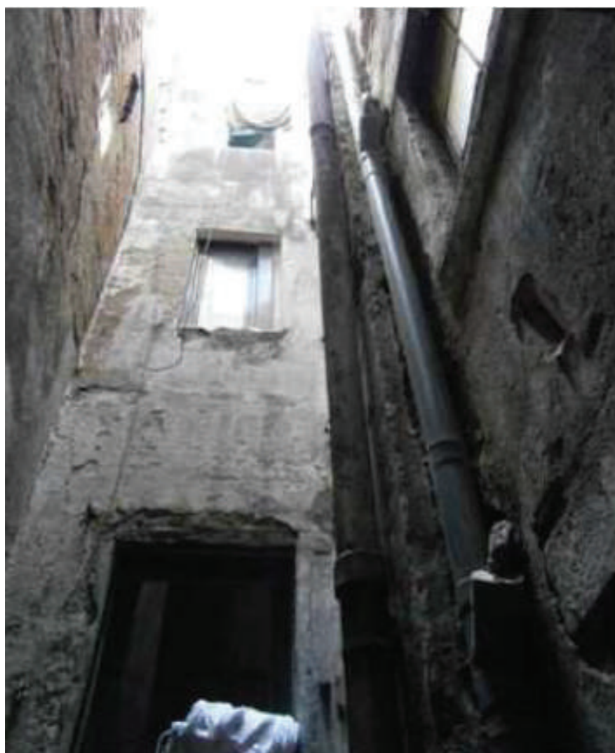
Fig.6: Condition of the inner patio prior to the intervention.
