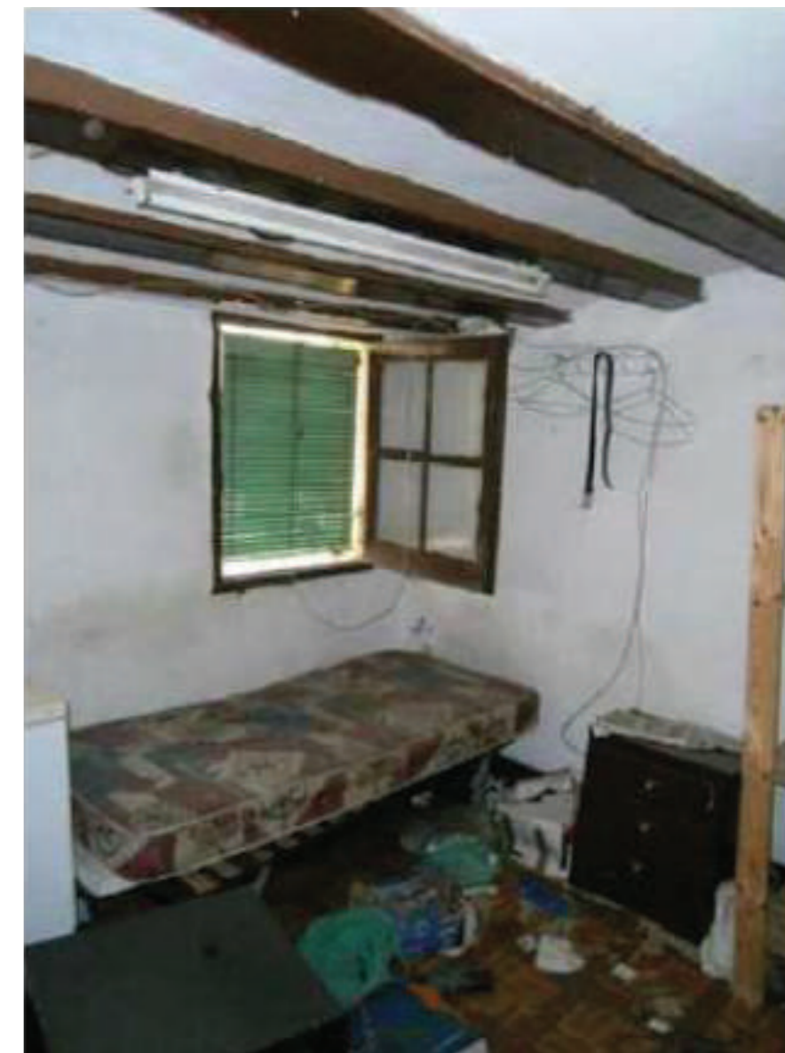
Fig.9: Conditions of the interior of dwellings prior to the intervention.
