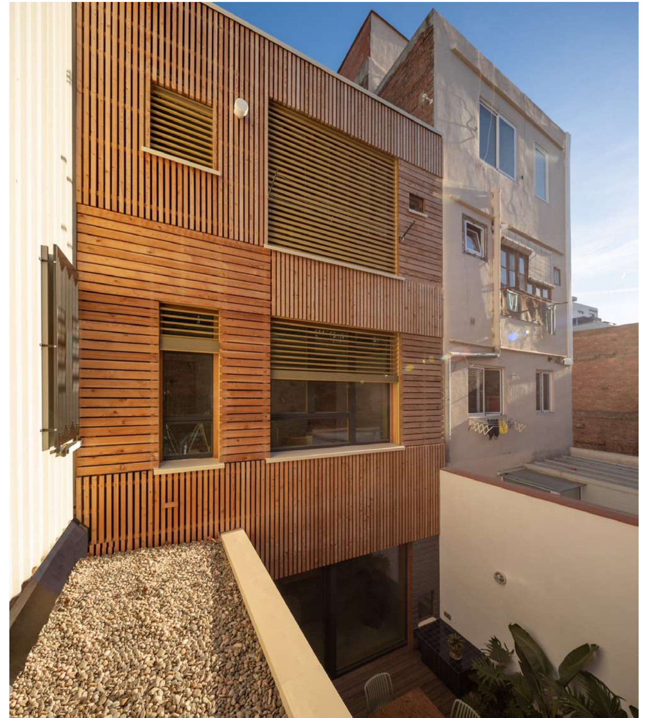
Fig.15: Courtyard's façade after the intervention.
