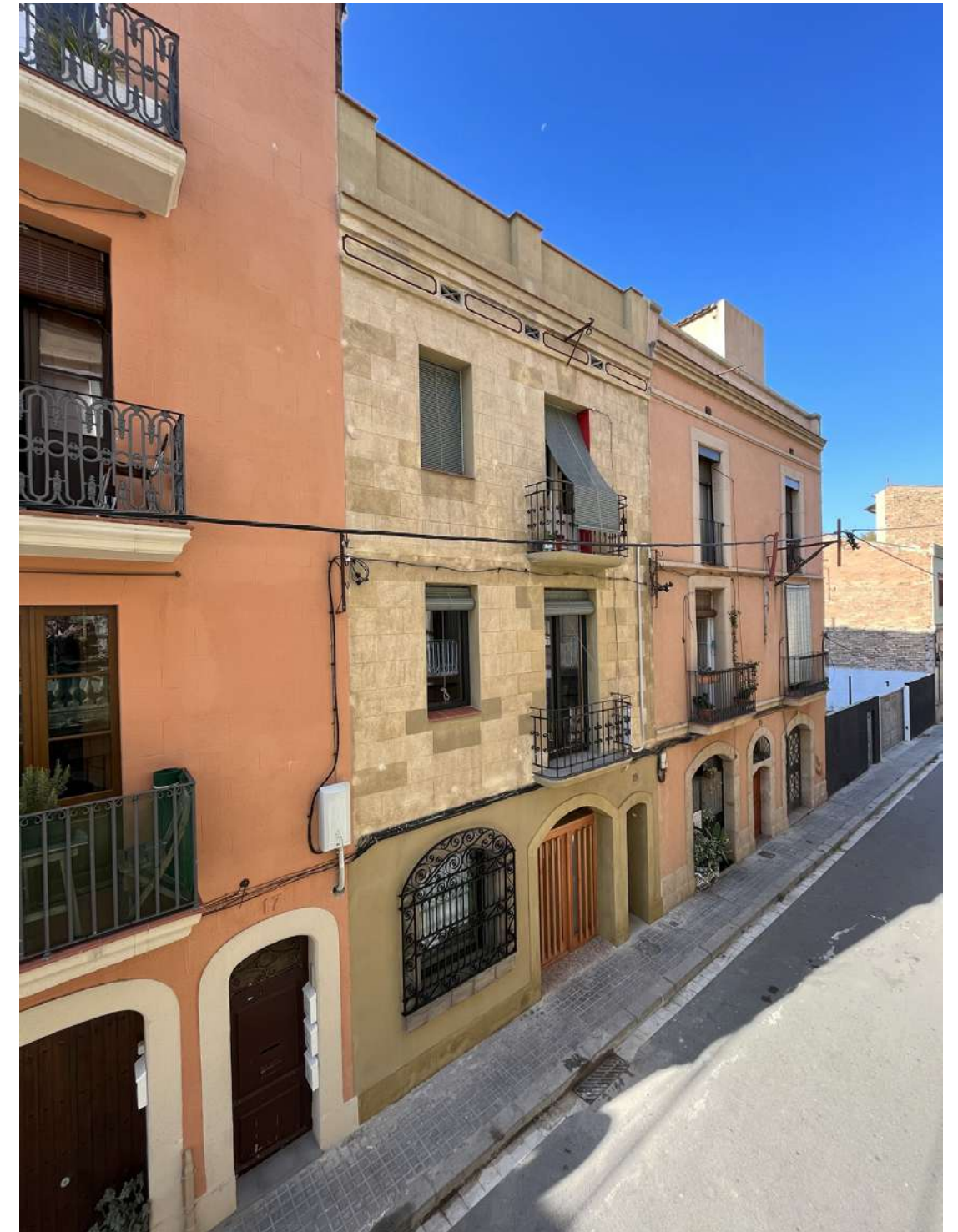
Fig.13: View of the restored main façade, and neighboring buildings.
