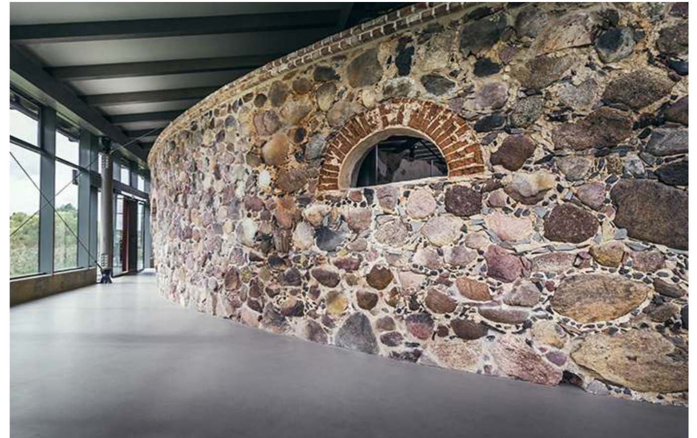
Fig.16: Interior fragment of cattle barn.
