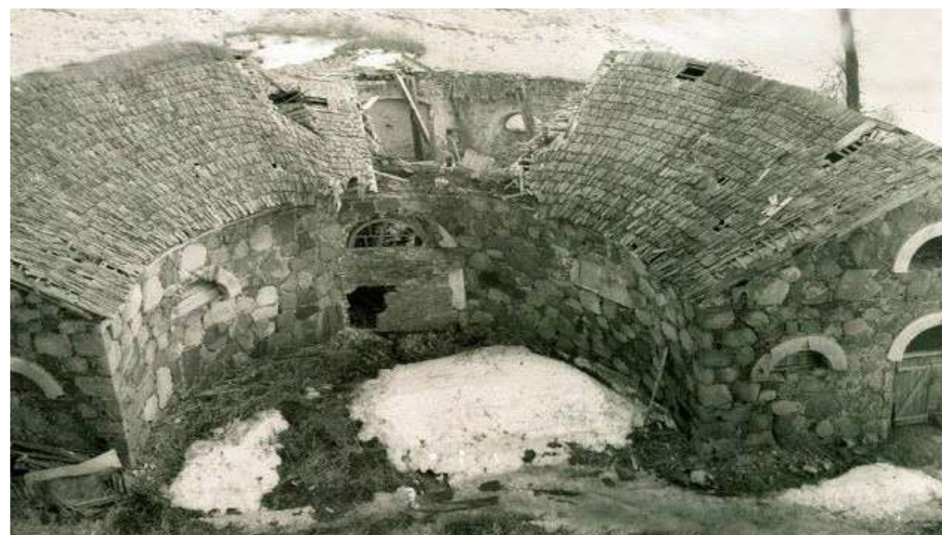
Fig.5: Cattle barn before restoration.
