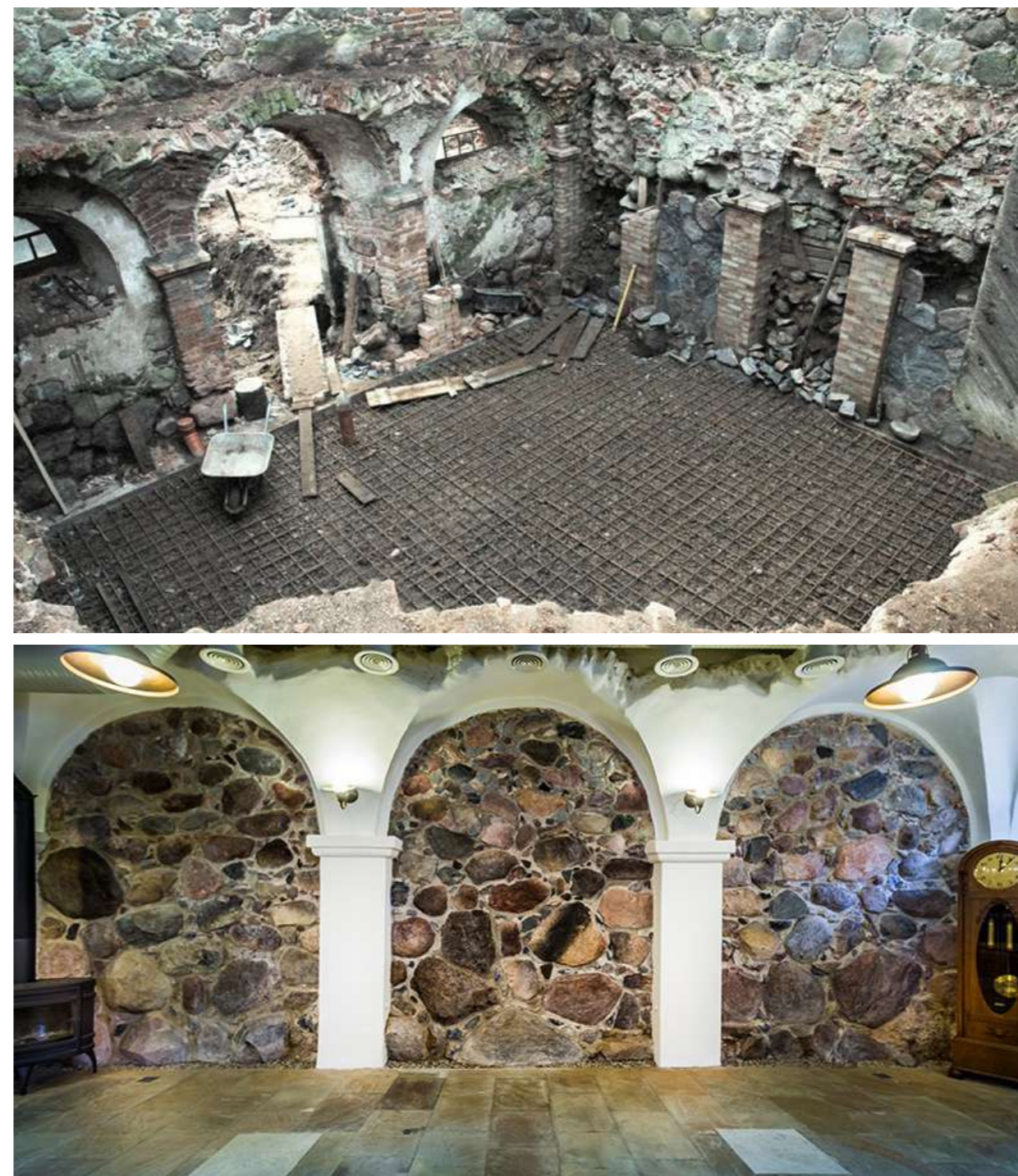
Fig.6: Interior of supervisor's house before and after renovation.
