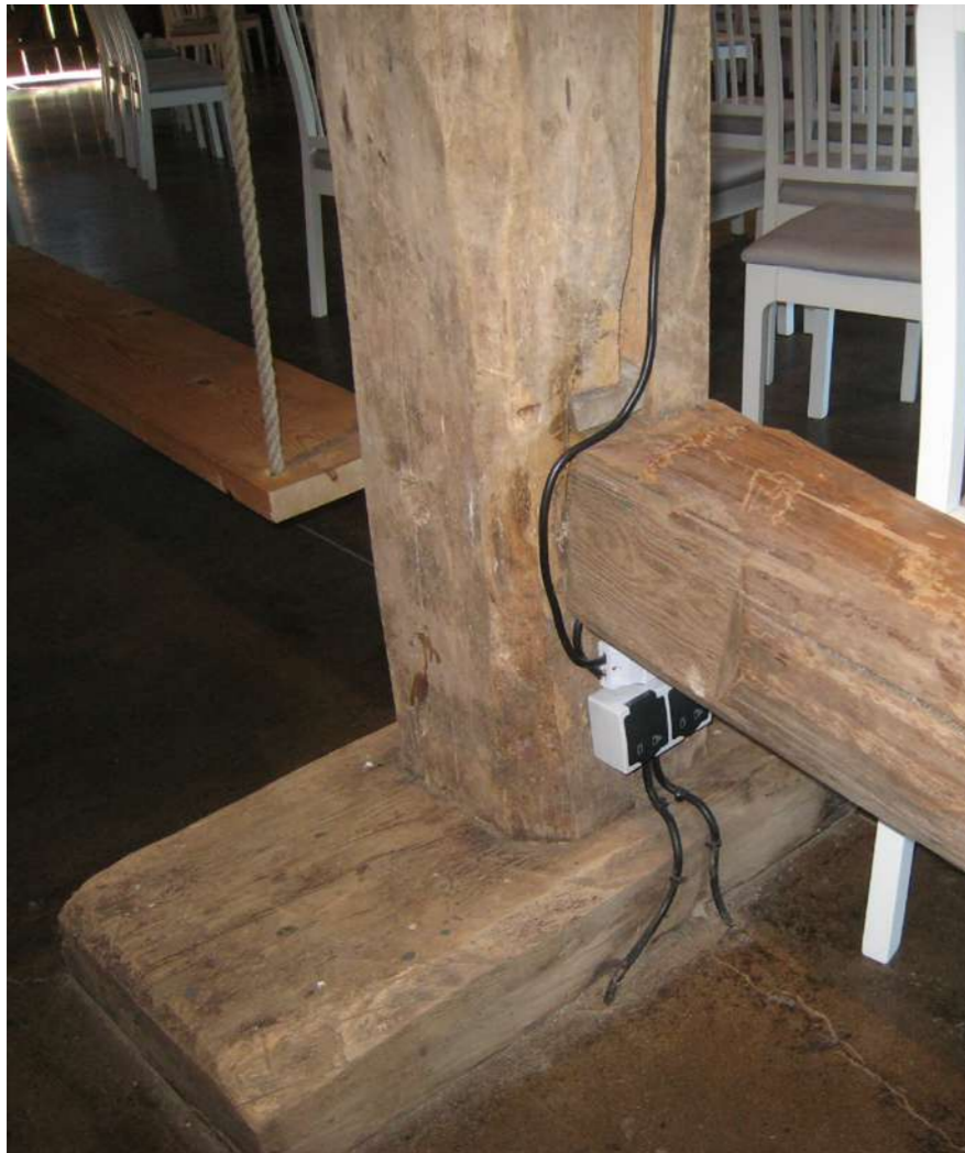
Fig.27-28: Connections of old and new parts.
