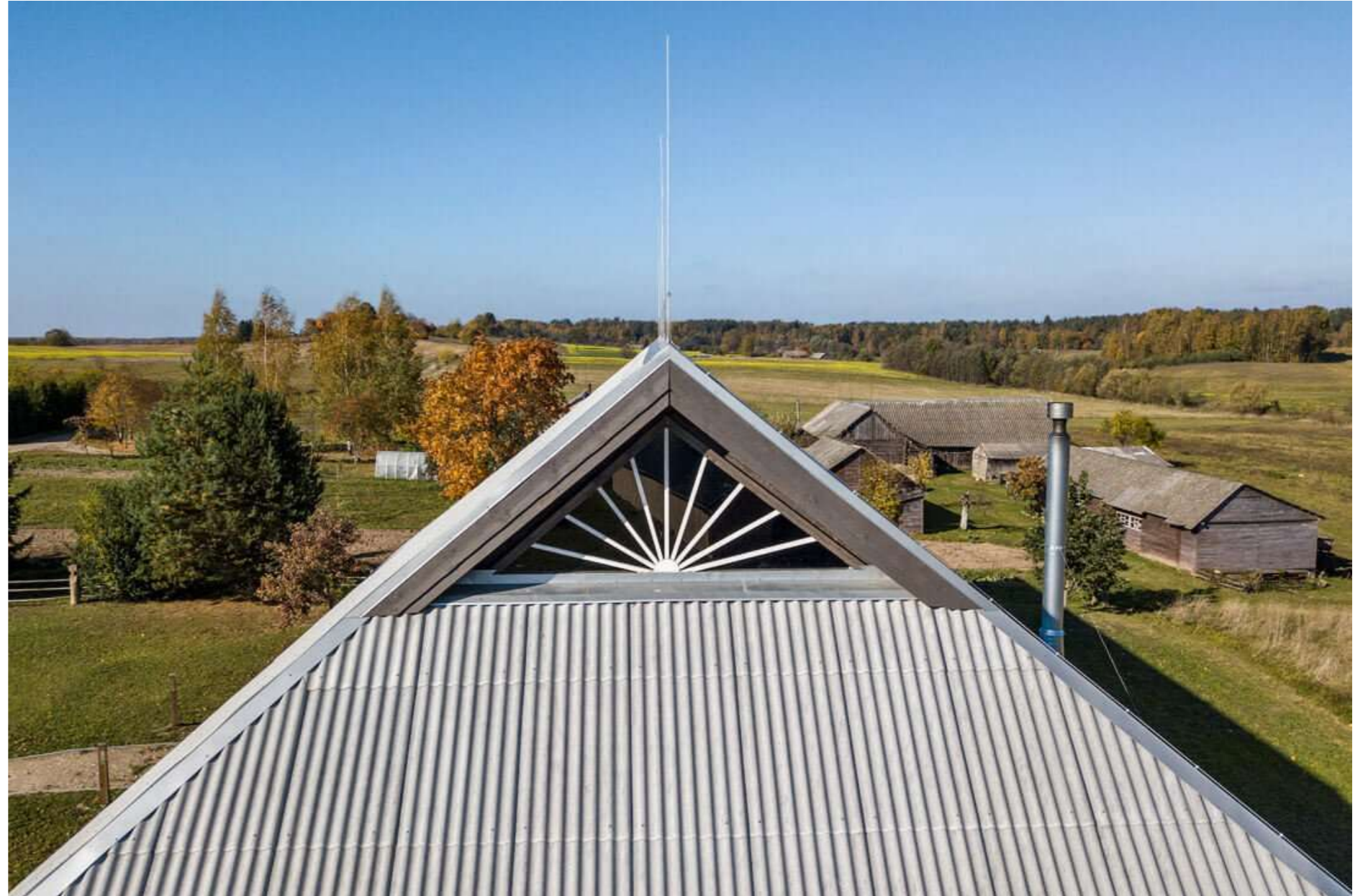
Fig.36: Opening at the ridge of the roof.
