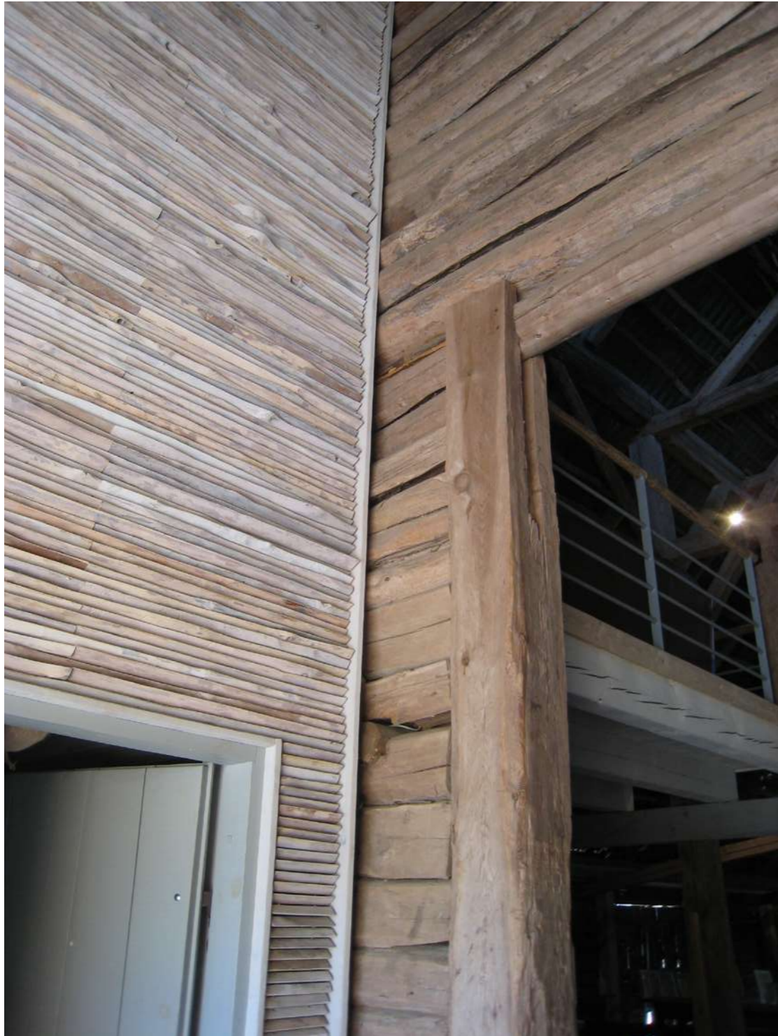
Fig.23: Connections of old and new parts.
