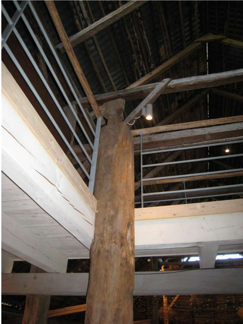
Fig.35: Connections of old and new parts.
