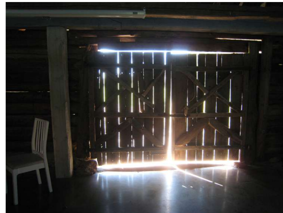
Fig.13: Threshing barn gate from the inside.
