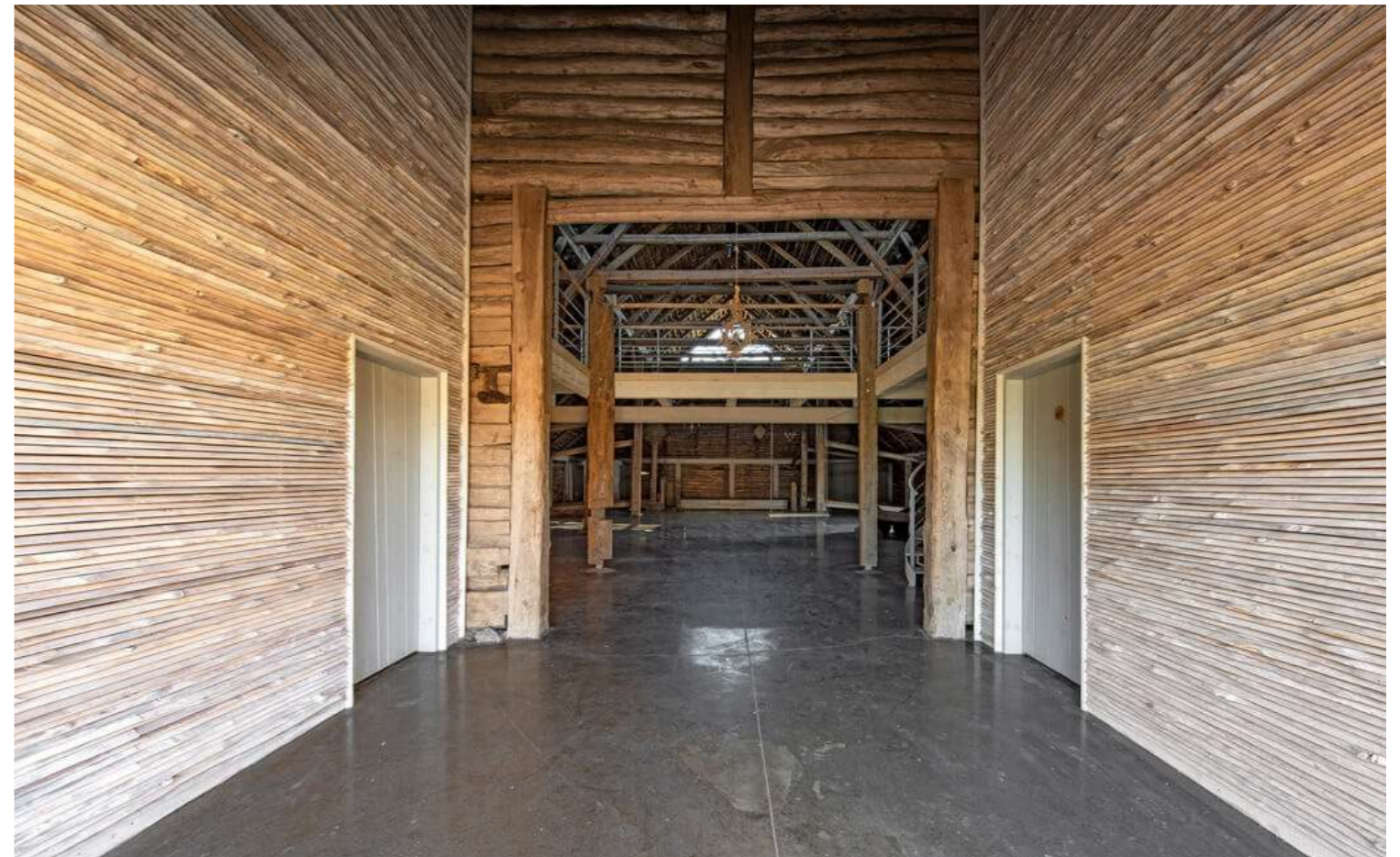
Fig.20: Hallway of threshing barn.
