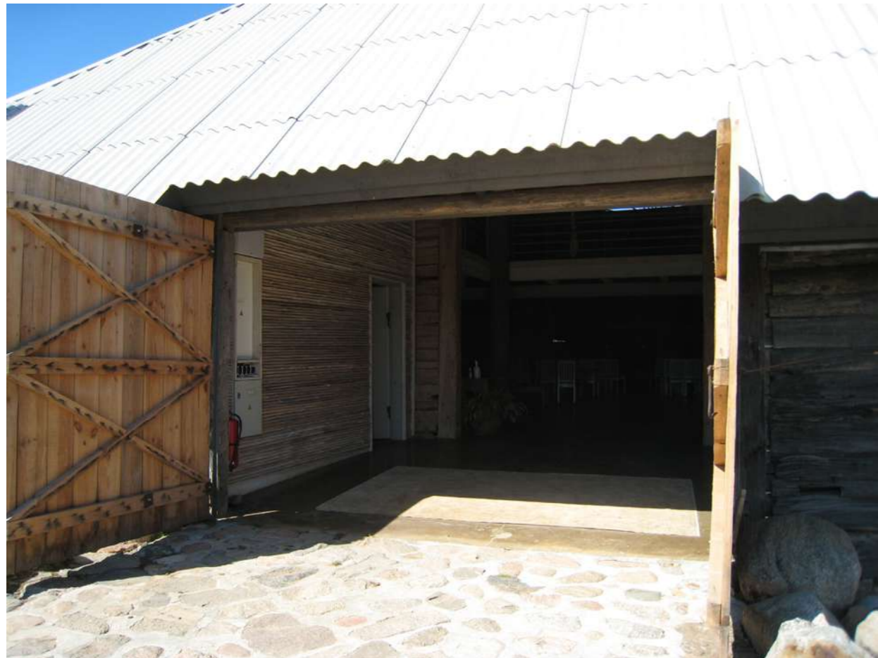
Fig.19: Entrance to the reconstructed threshing barn.
