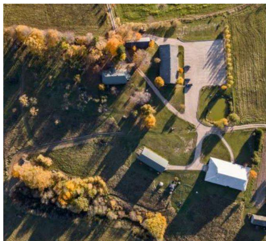
Fig.5: View of the homestead from a bird's eye view before reconstruction.
