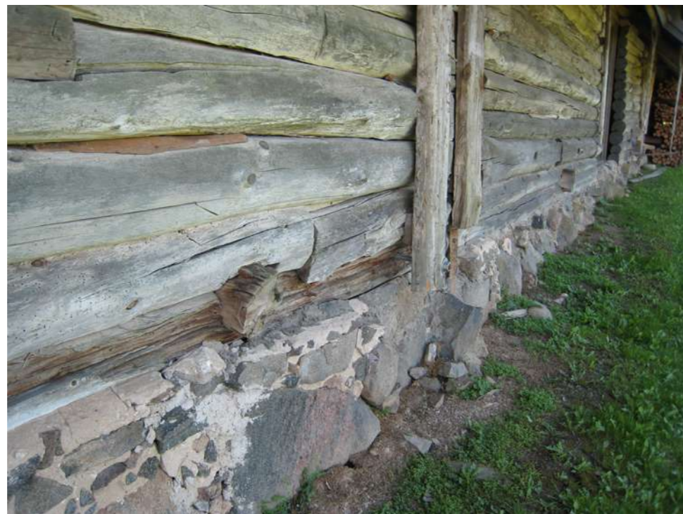
Fig.12: Threshing barn wall.
