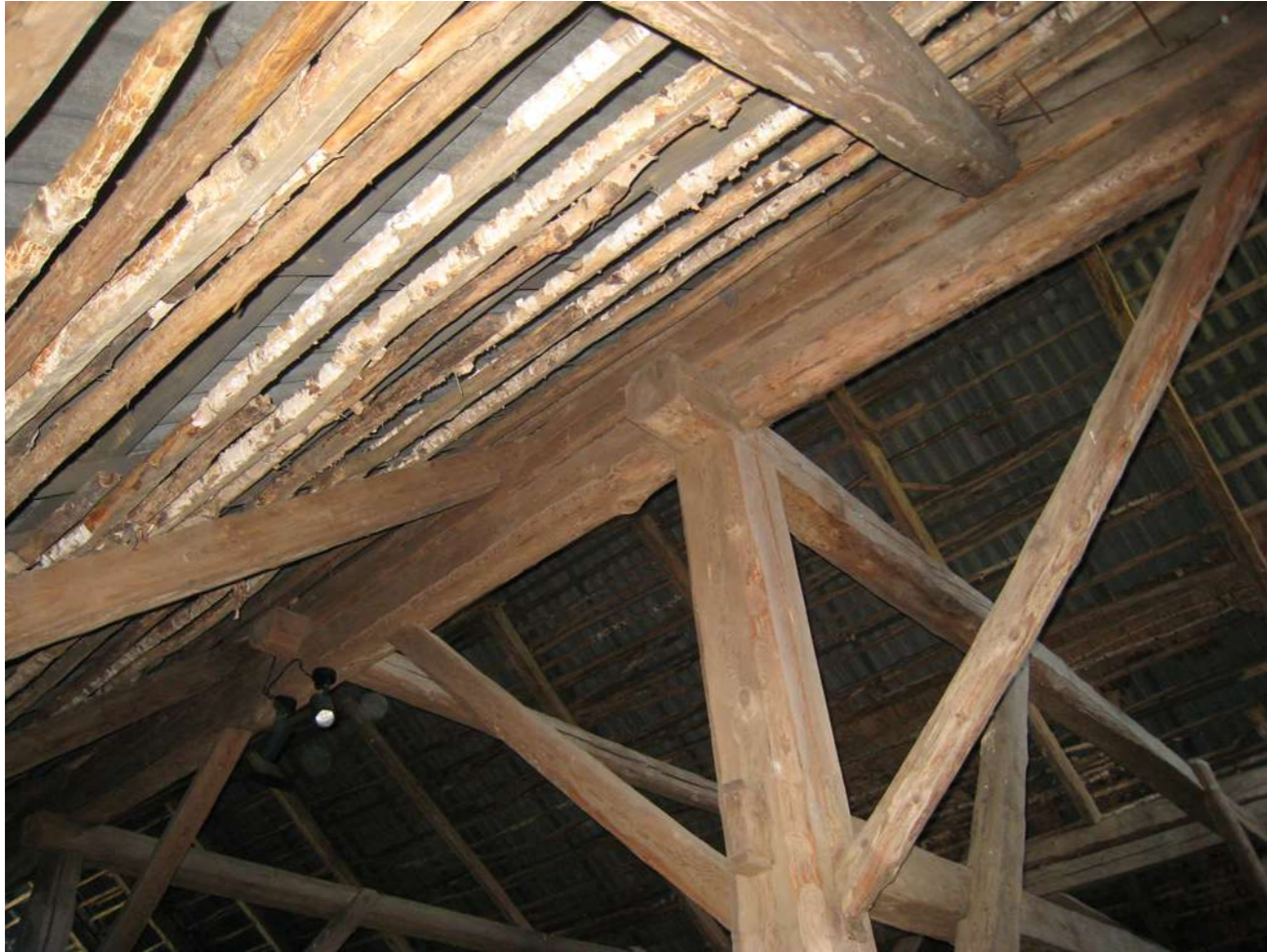
Fig.33: Old roof construction.
