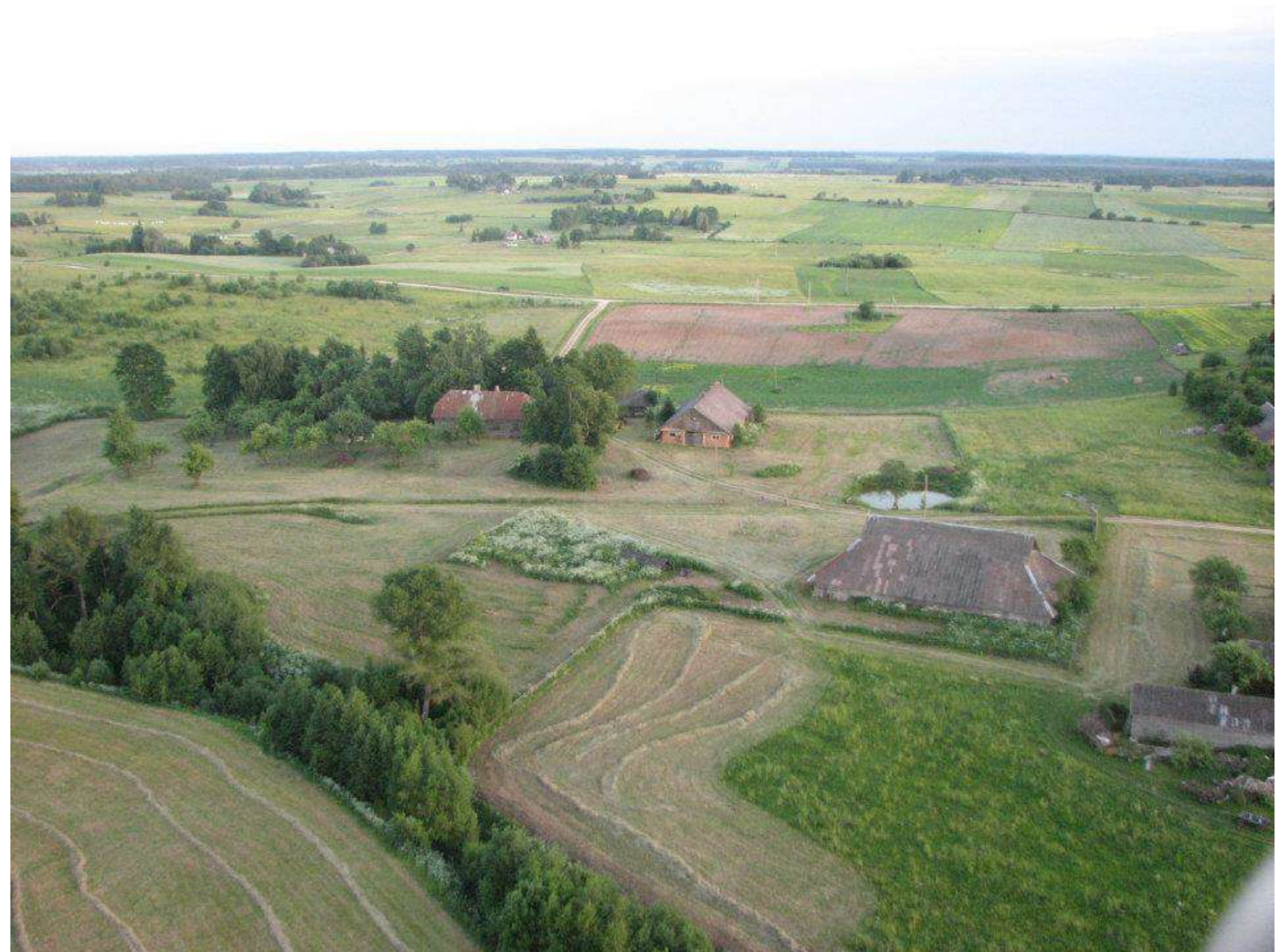
Fig.3: View of the homestead from a bird's eye view before reconstruction.
