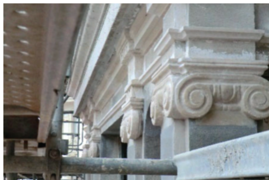
Fig.24-25: Restoration and rehabilitation of the ornamental elements of the tribunes.
