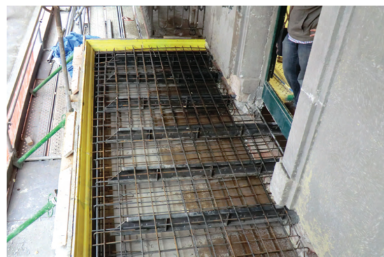
Fig.20-22: Substitution profiles in overhangs of tribunes; Fig.23: Detailed drawing of substitution profiles in overhangs.
