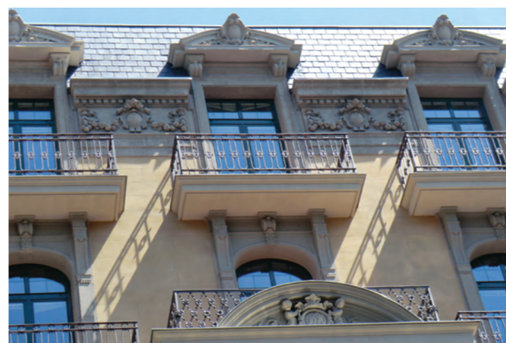
Fig.1: Detail of mansard windows and Agullers Street's façade.
