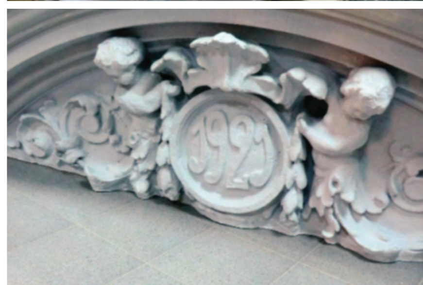
Fig.26-27: Restoration and rehabilitation of the ornamental elements of the mansard windows.
