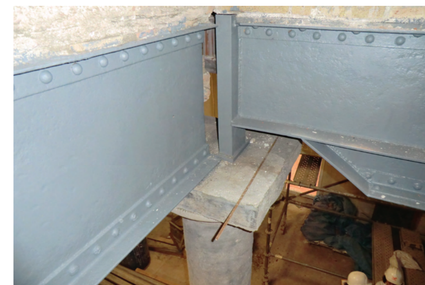
Fig.11-12: Rehabilitation of the capitel and head of the composite profile beam.
