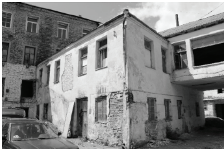
Fig.5: Views of the complex before reconstruction.
