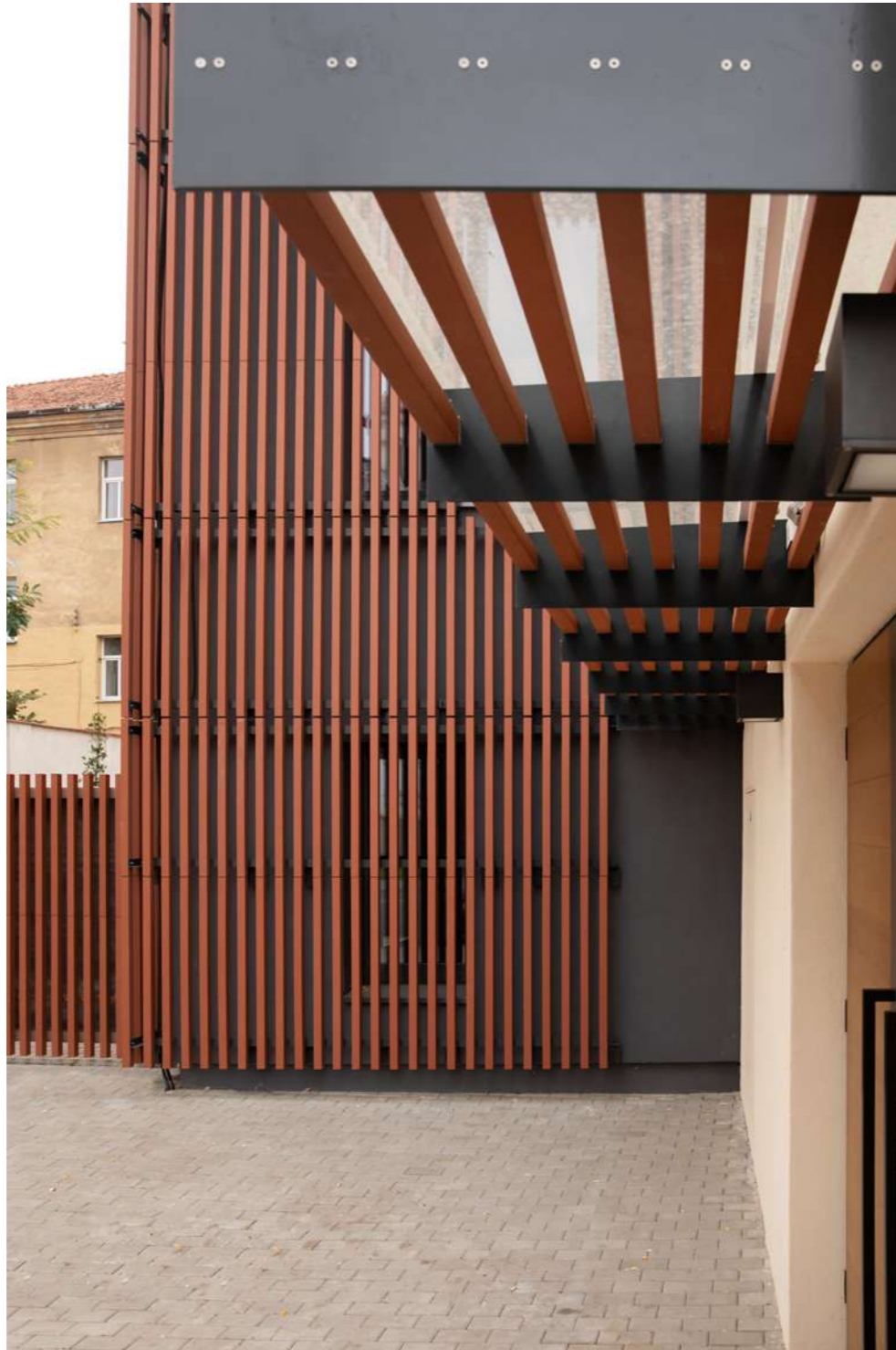
Fig.14: New elements in the exterior of the building.
