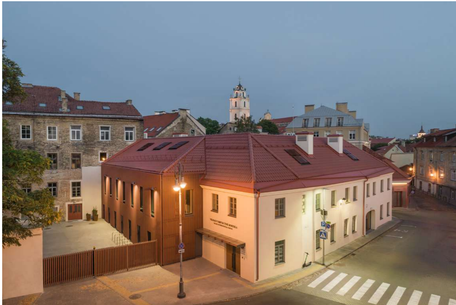
Fig.7: View of the restored building.
