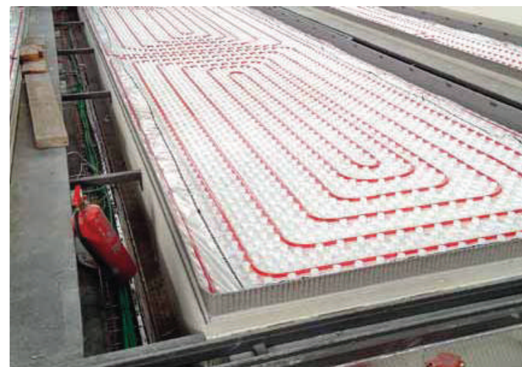
Fig.4-5: Installation of the new elevator, and radiant floor systems.
