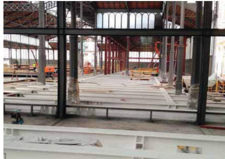
Fig.6: Construction of the new steel and glass enclosures.
