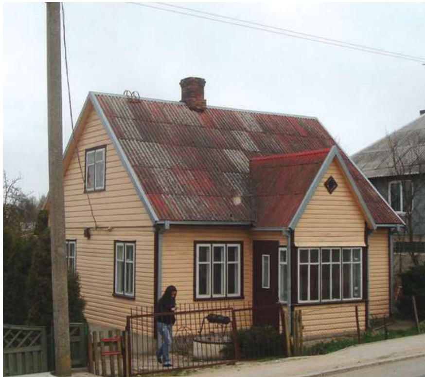
Fig.5: Building before renovation.
