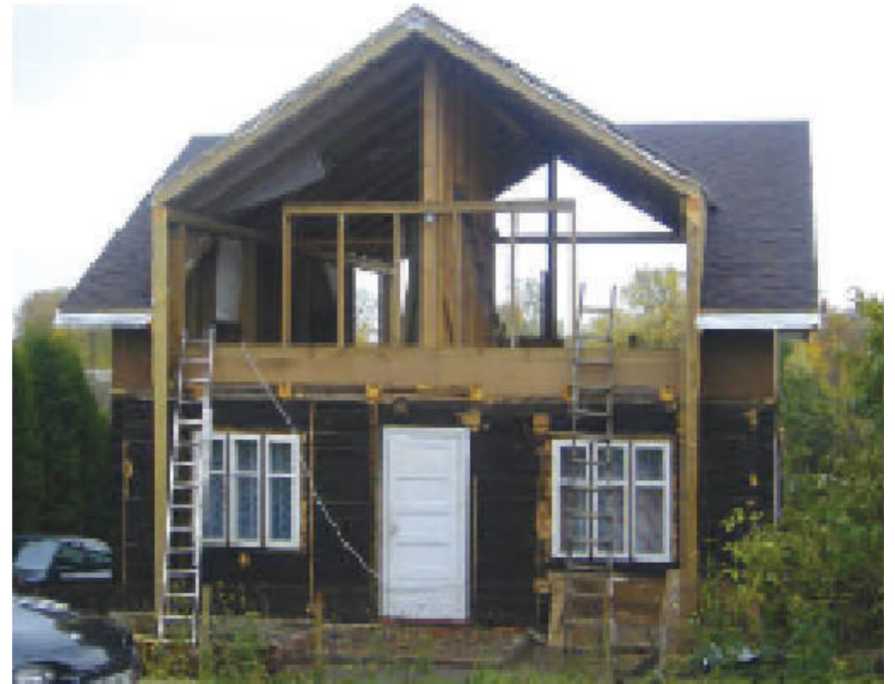
Fig.12: Building during renovation works.
