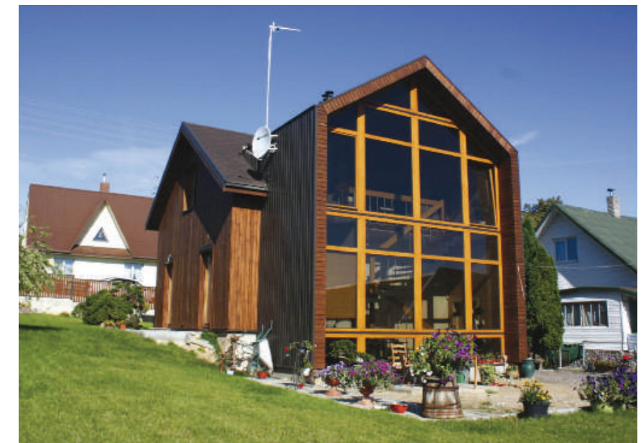
Fig.4: View of the renovated building from the courtyard.
