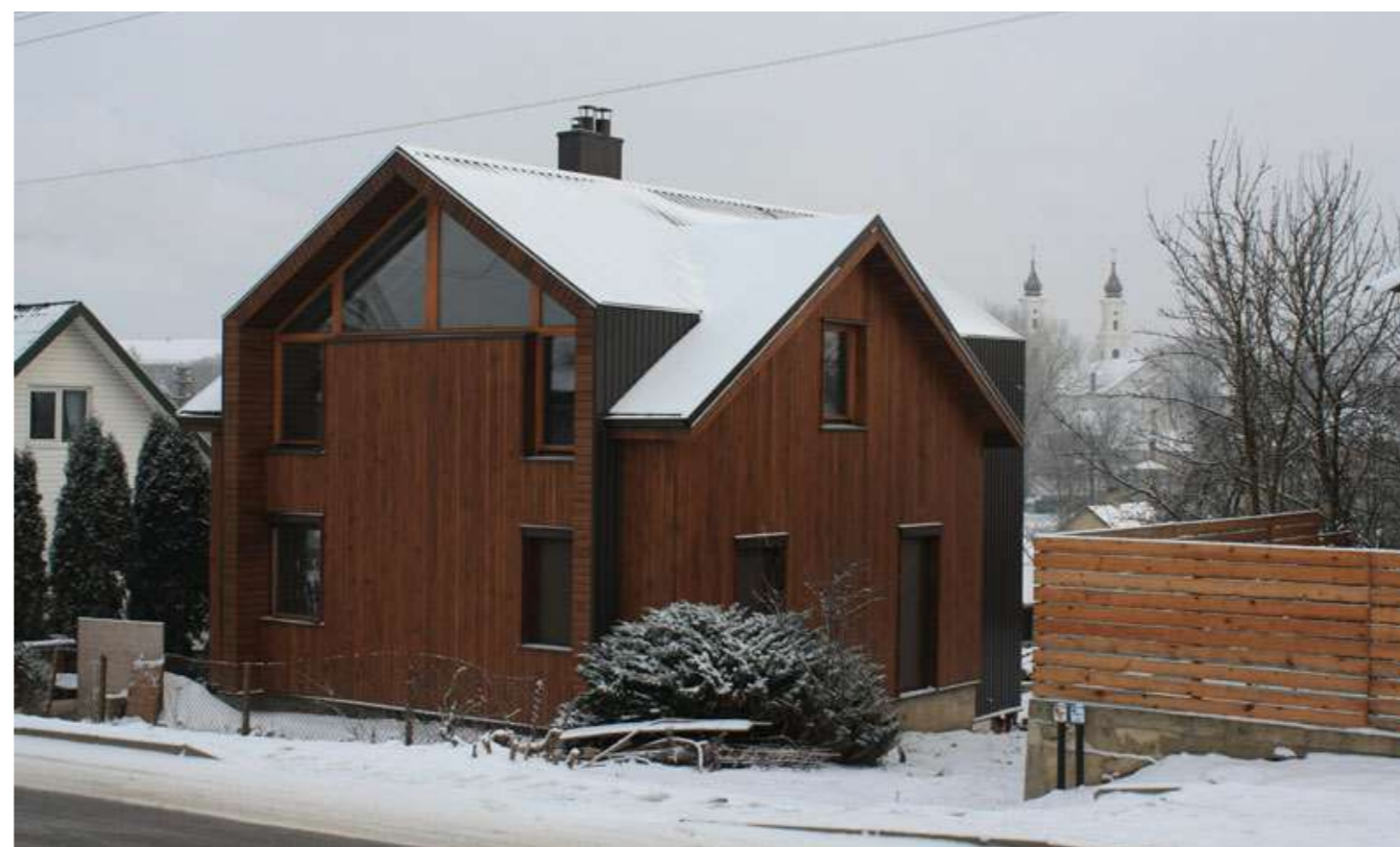
Fig.8: View of the renovated building.
