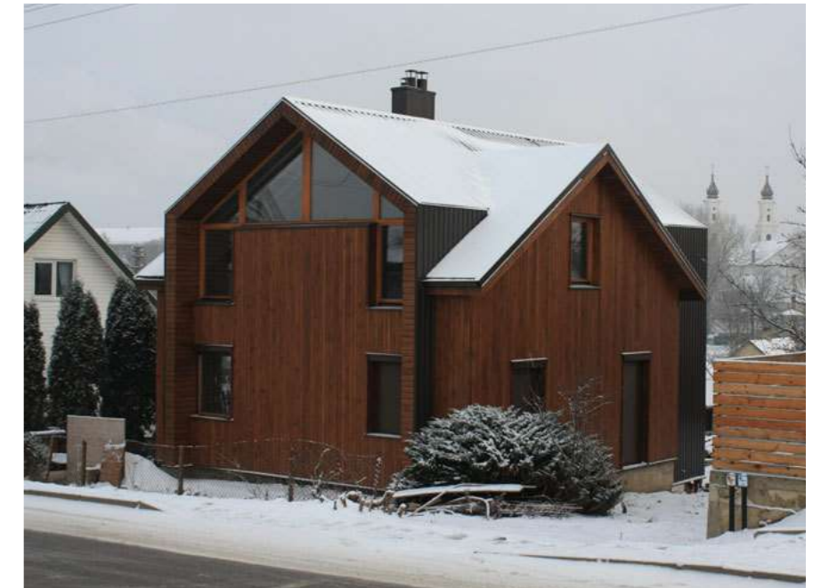
Fig.3: View of the renovated building from the street.
