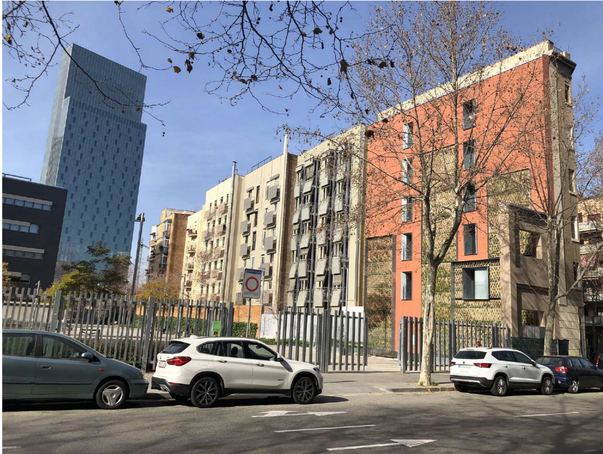
Fig.7: View of the urban renovation.
