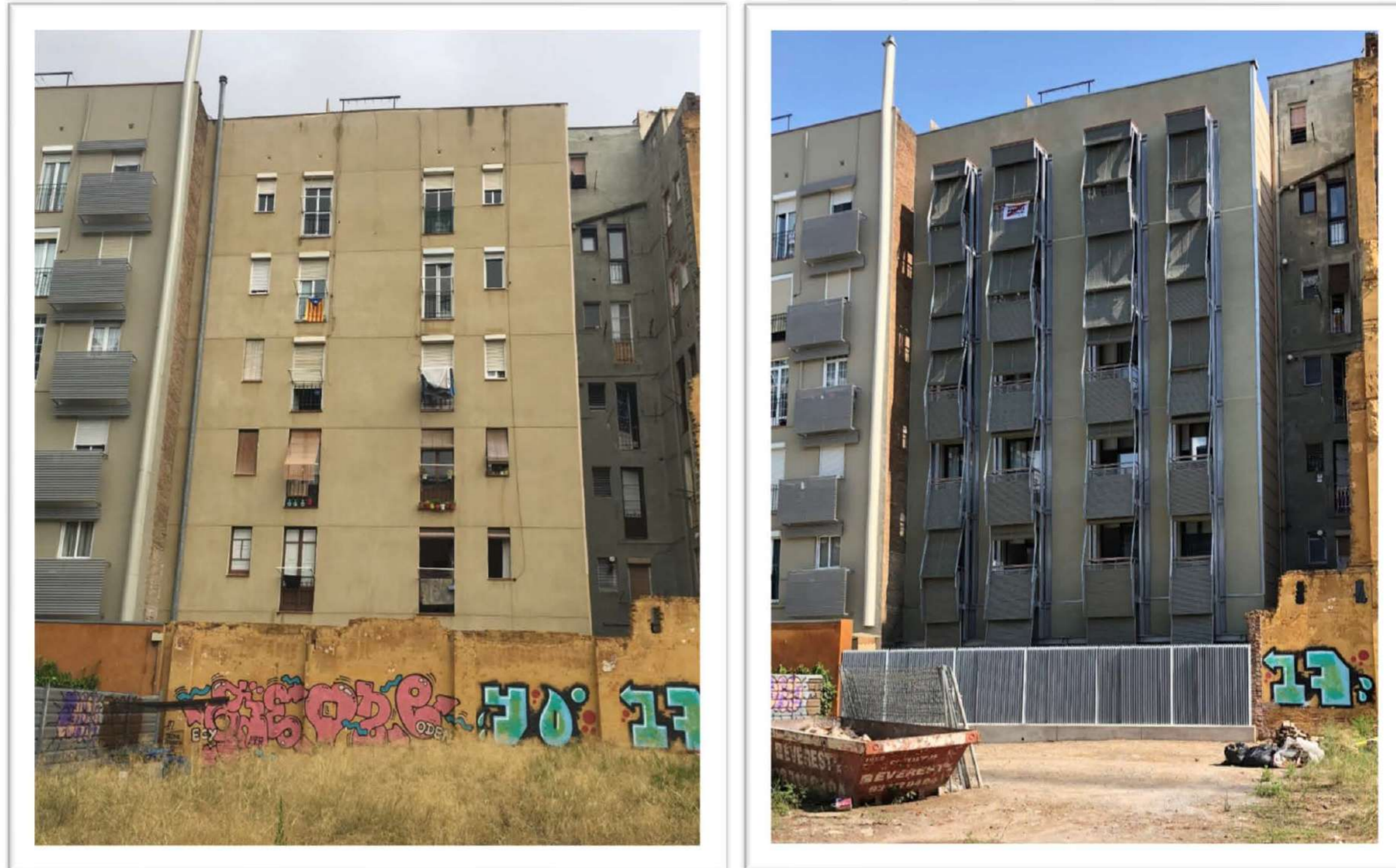
Fig.6: Before and after of the intervention.
