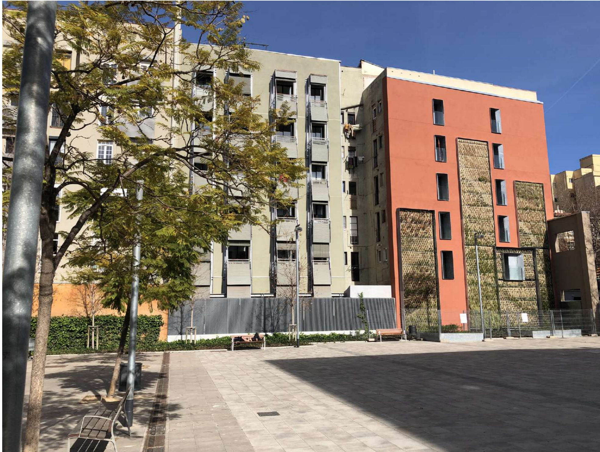
Fig.8: View of the urban renovation.
