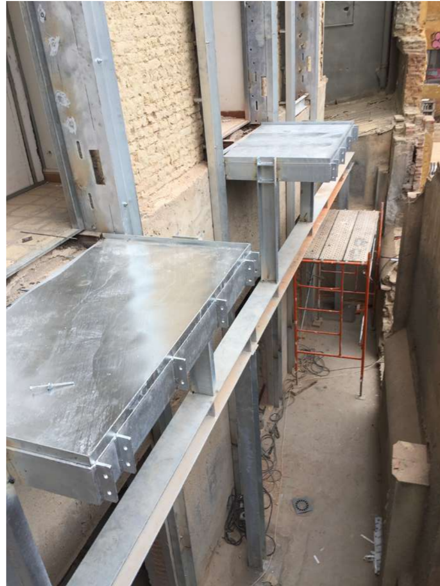
Fig.16: installation of the balconies.
