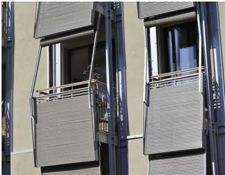
Fig.10: Detail of the finished balconies.
