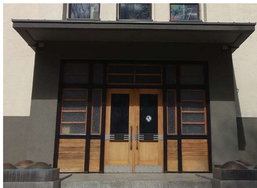
Fig.21-22: Entrance before and after restoration.
