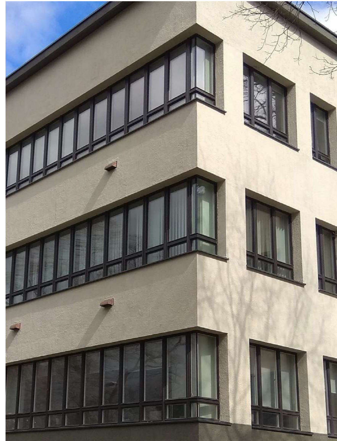
Fig.9: View of the windows.
