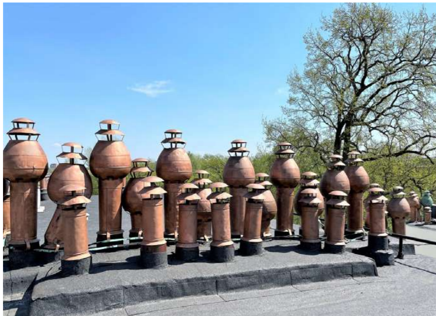
Fig.25: Original ventilation chimneys before and after renovation.
