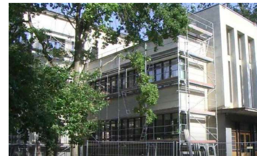
Fig.23: Renovation of the building's façade.
