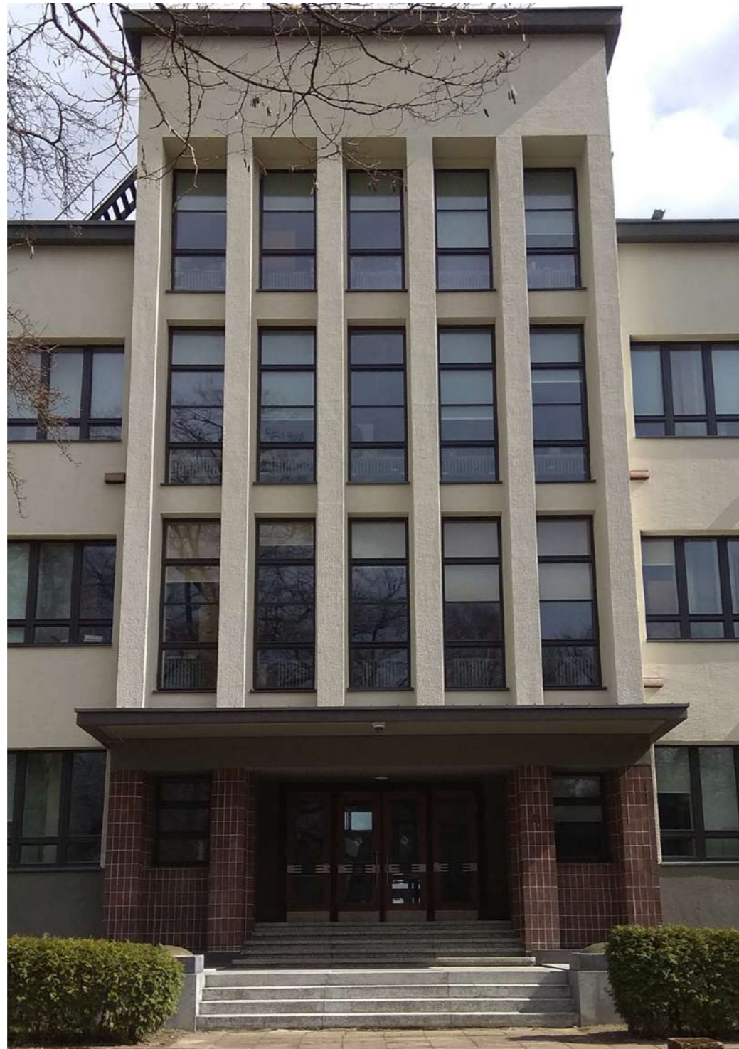
Fig.8: Central part of the west façade.
