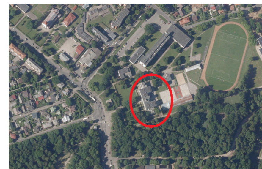
Fig.3: Satellite image of the building.
