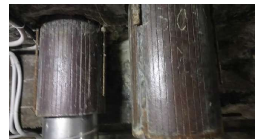
Fig.24: Old ventilation pipes used in conjunction with new details.
