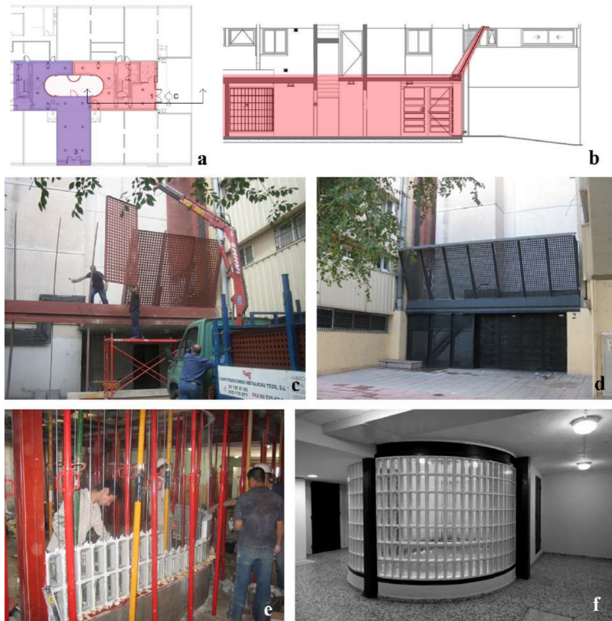
Fig.8: Design and execution of the refurbishment of the first floors at Mina Nueva.
