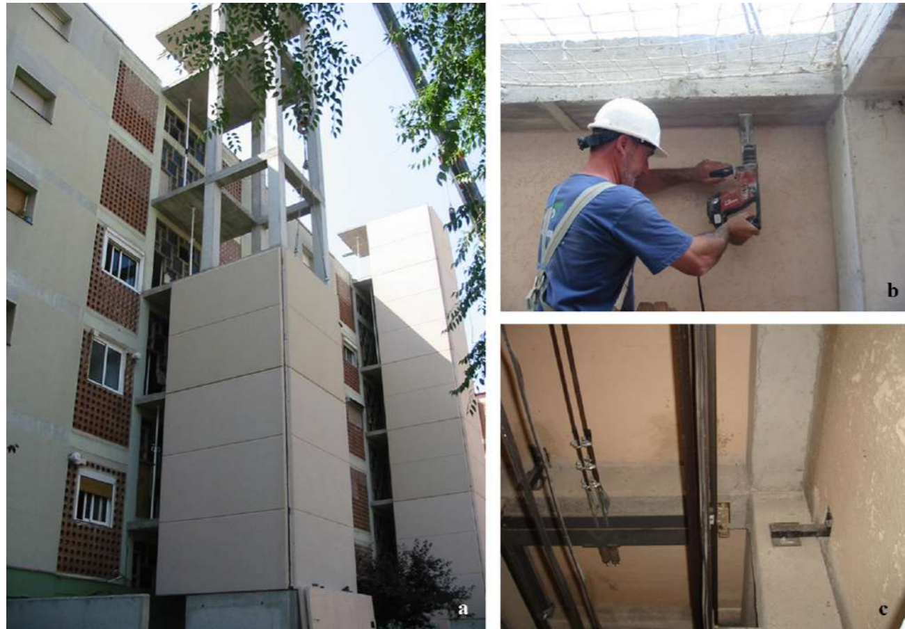
Fig.12: Installation of the external enclosure of the elevators.
