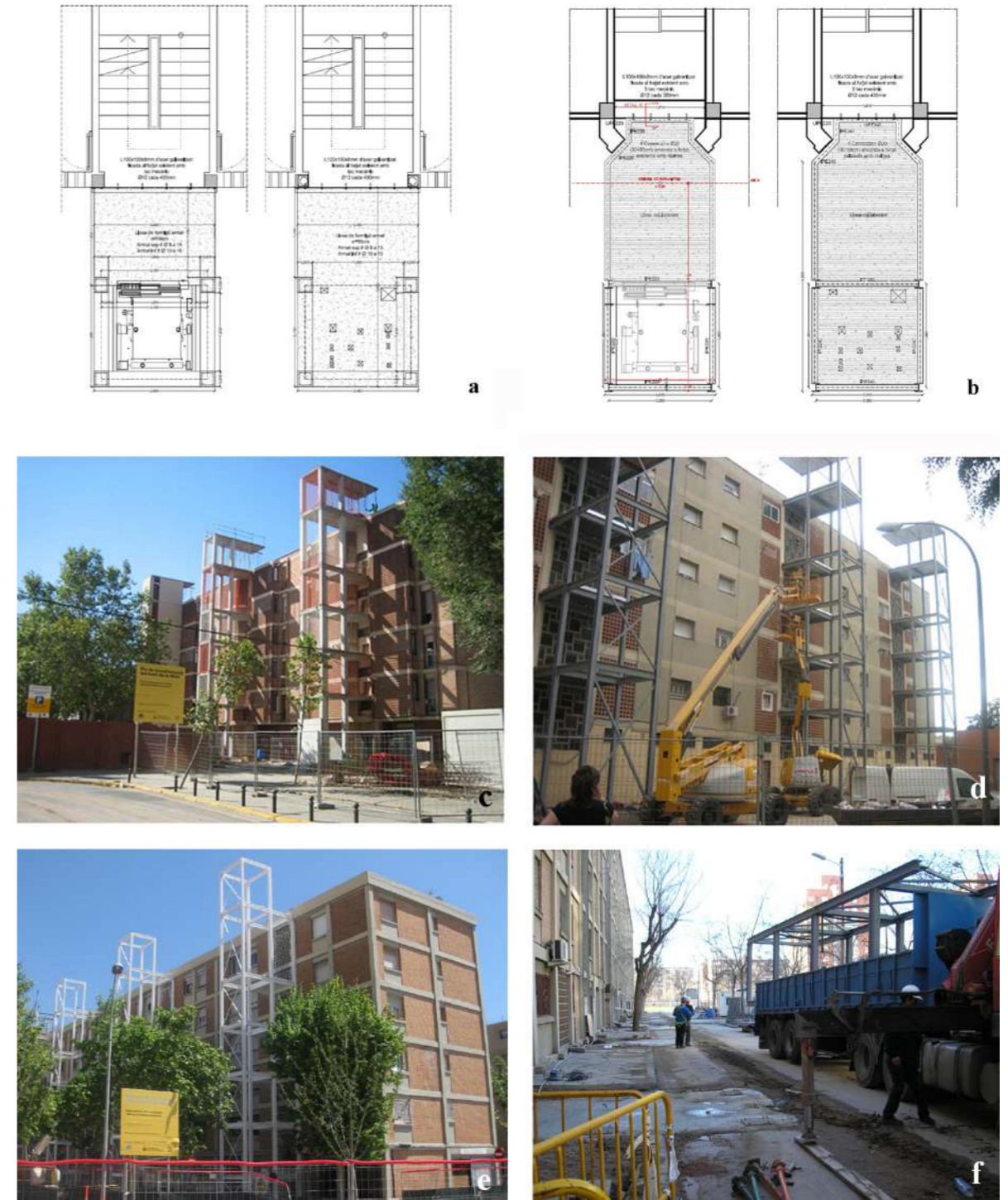
Fig.11: Addition of the exterior structure containing the elevators.
