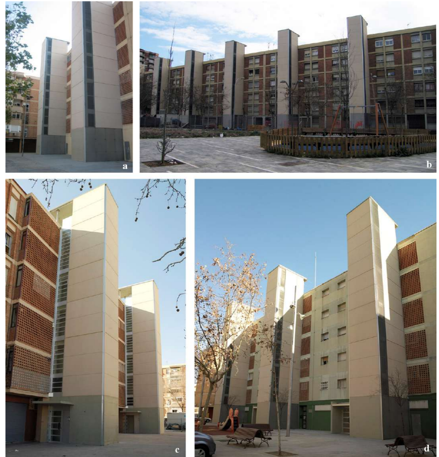
Fig.14: Exterior image of the elevator modules.
