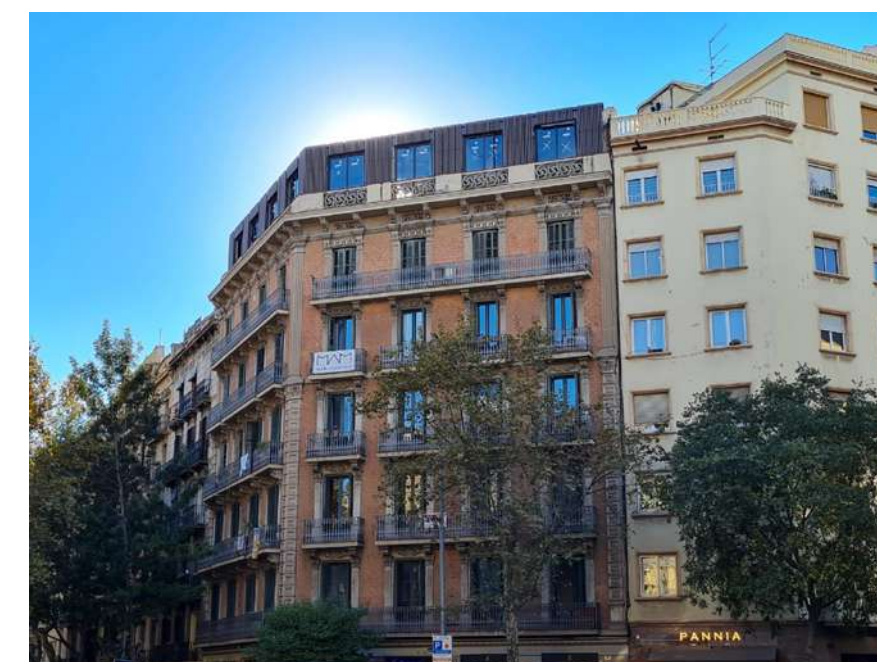
Fig.7: Main façade with all the modules already in place.
