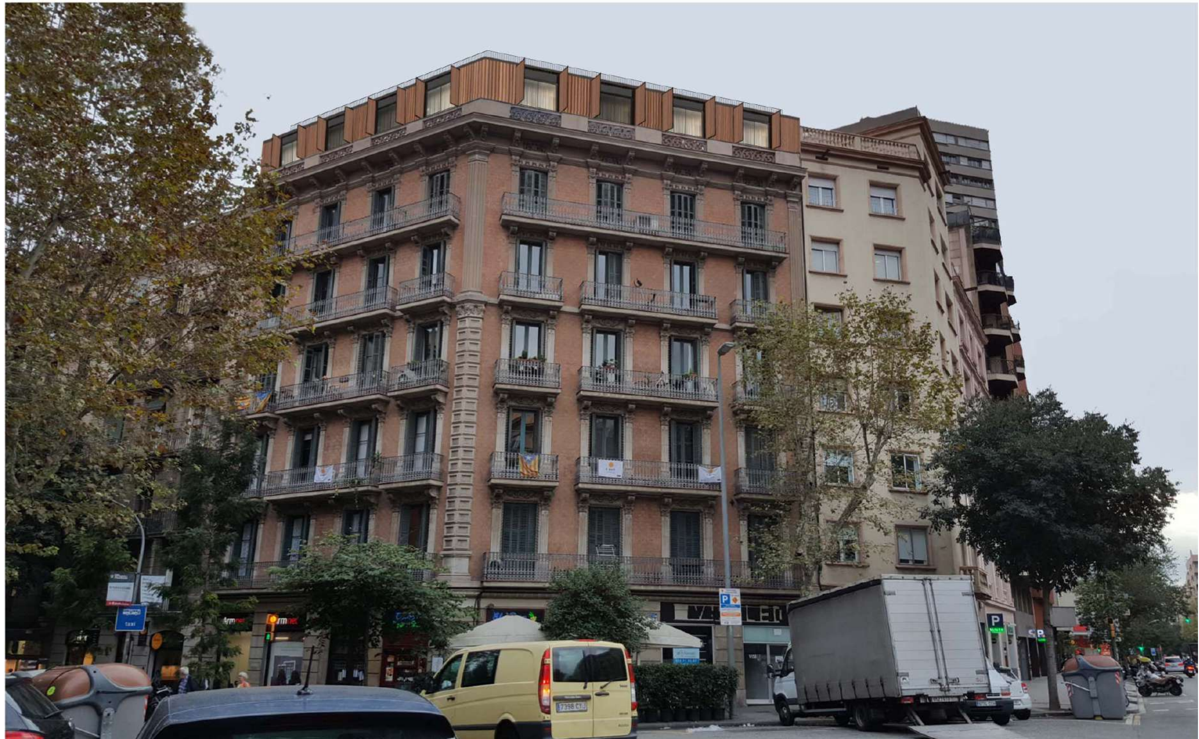
Fig.10: Perspective of the main façade with the proposed intervention (with windows opened).
