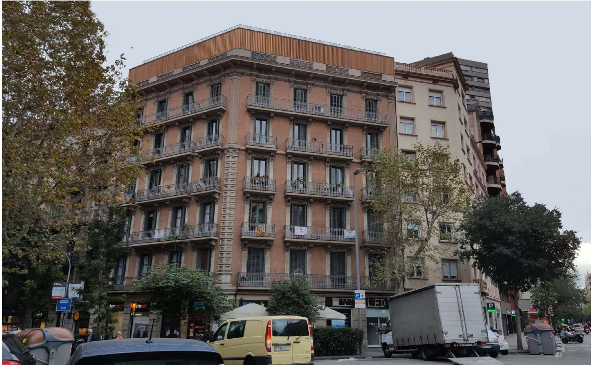
Fig.9: Perspective of the main façade with the proposed intervention (with windows closed).
