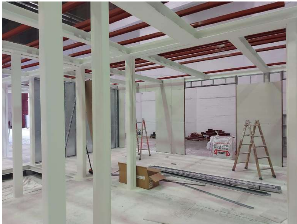
Fig.11: View of the pre-fabrication process of the modules (interiors).
