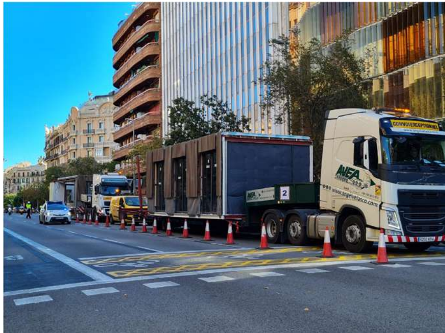
Fig.8: Transporting the pre-fabricated modules to the construction site.
