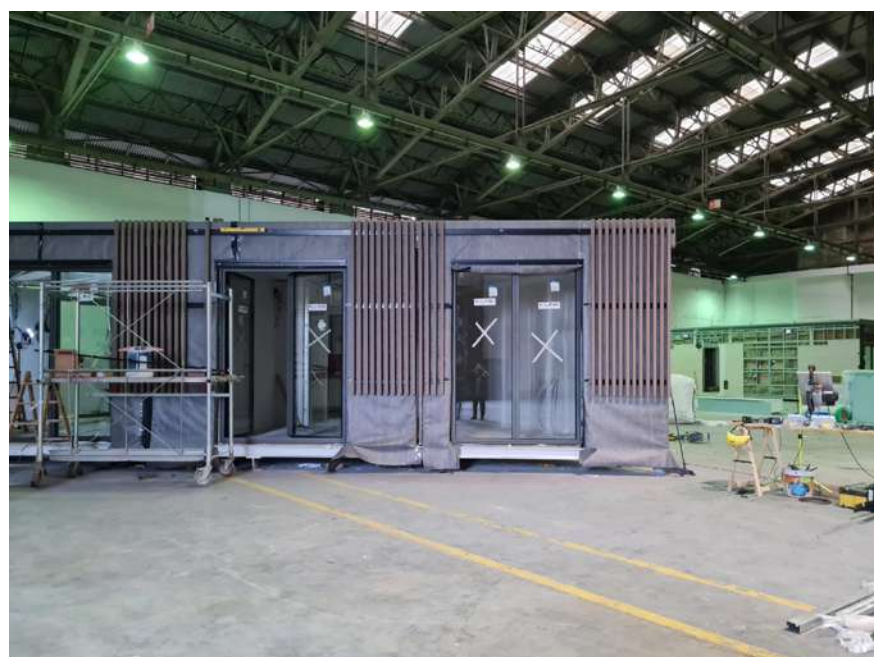
Fig.5: View of the pre-fabrication process of the modules (exterior).
