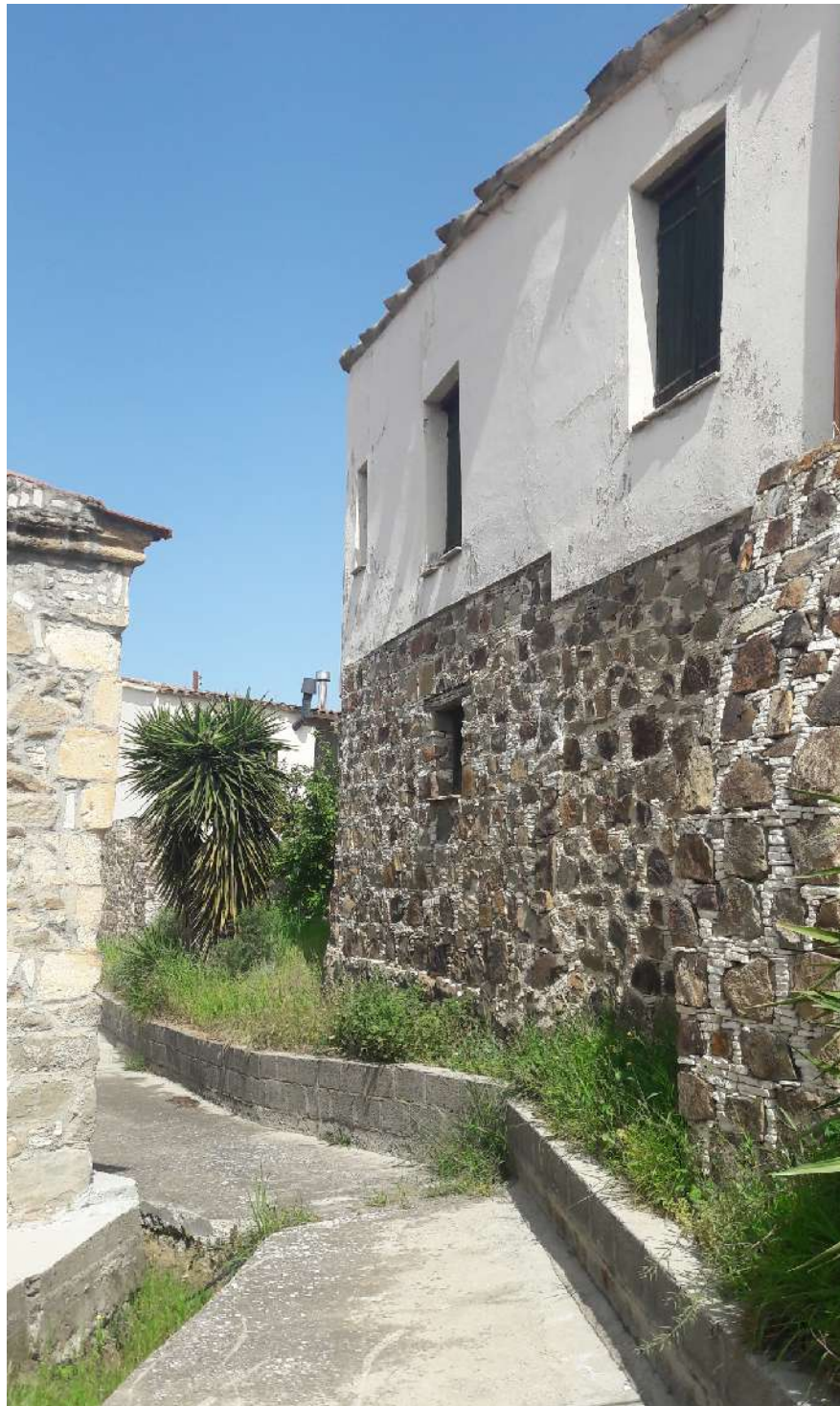
Fig.6: Side elevation of house. © N. Chrysochou
