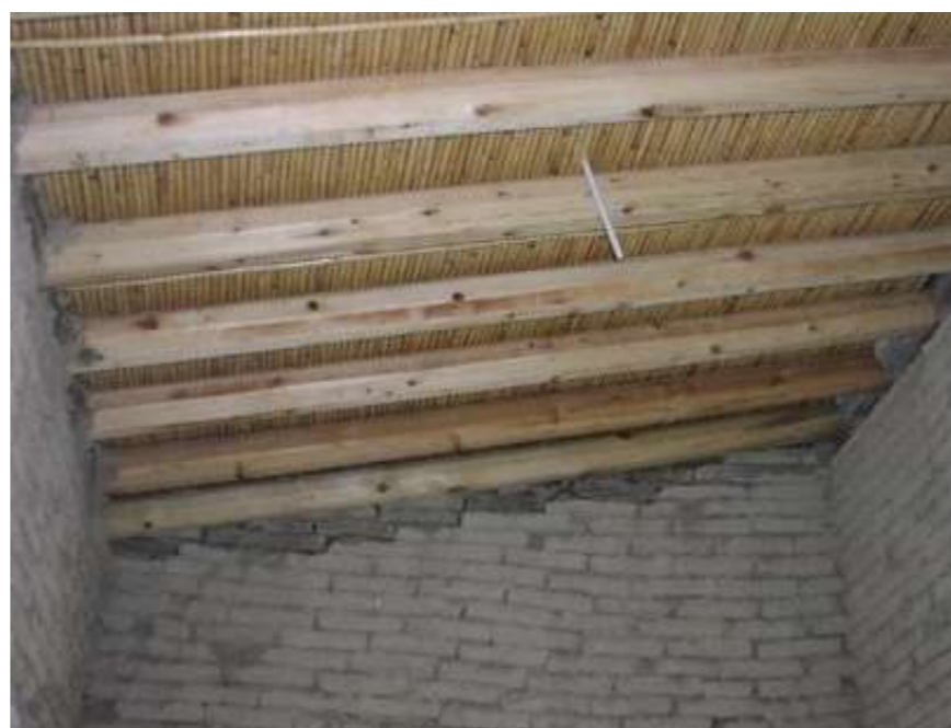
Fig.13-16: Restoration of timber roofs with the use of traditional materials and techniques. © M. Philokyrou
