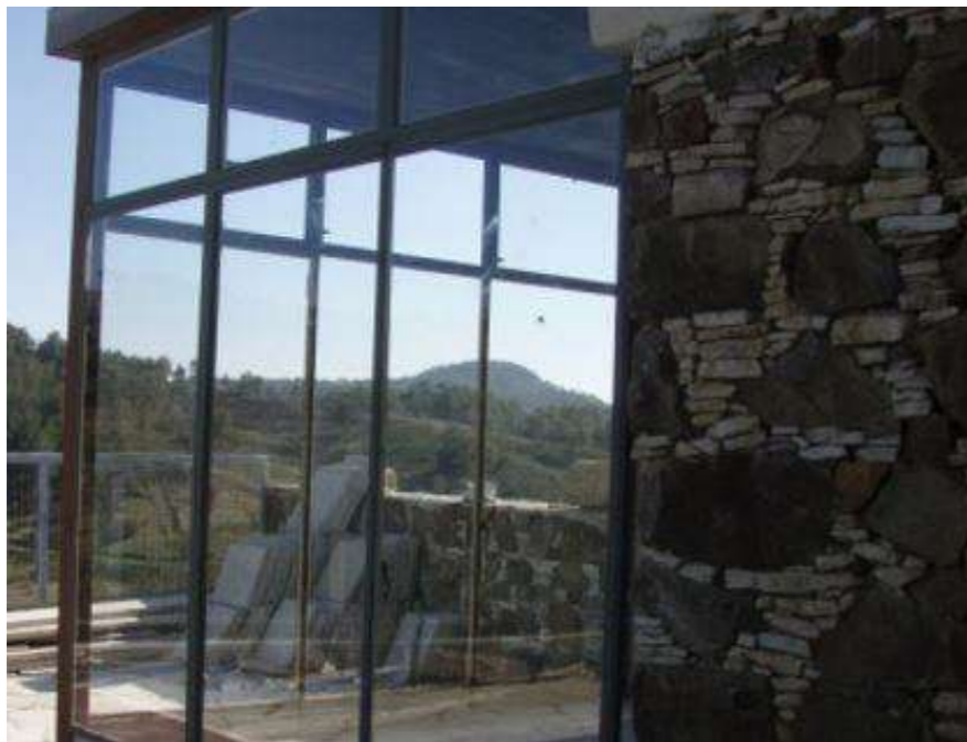
Fig.20-21: Erection of two lightweight contemporary structures with the use of glass surfaces. © M. Philokyprou
