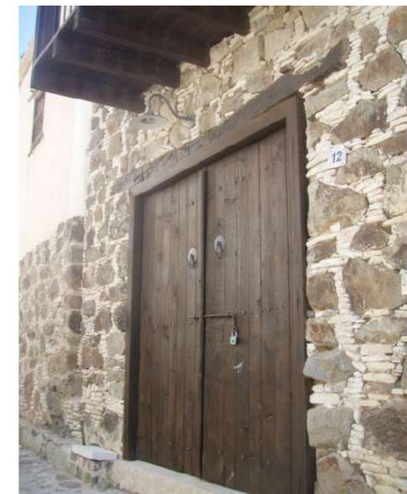
Fig.31: View of the main entrance after restoration. © M. Philokyprou
