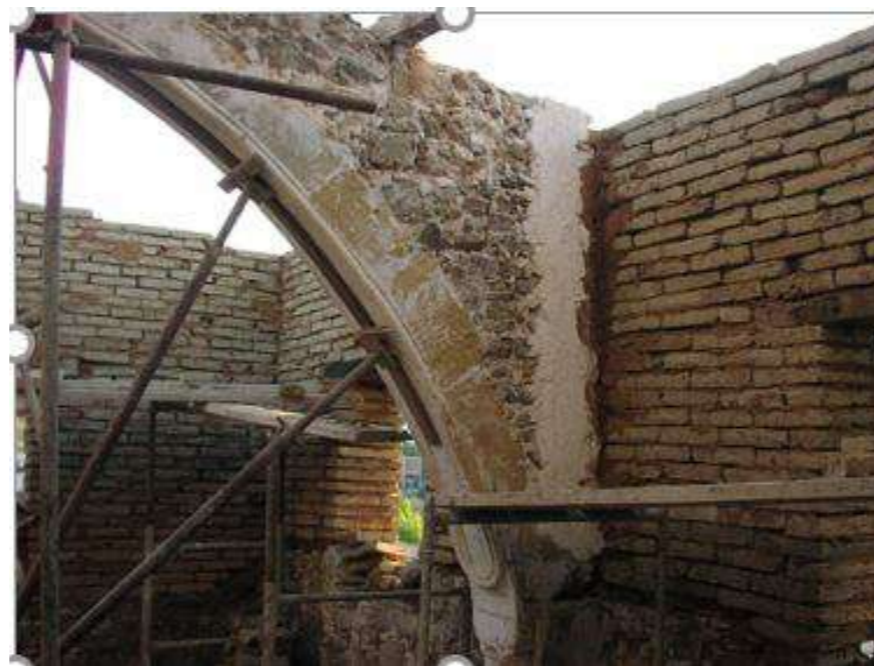
Fig.10: Maintenance of the original traditional materials, and use of a metal structure above the main arch of dichoro. ©M. Philokyprou
