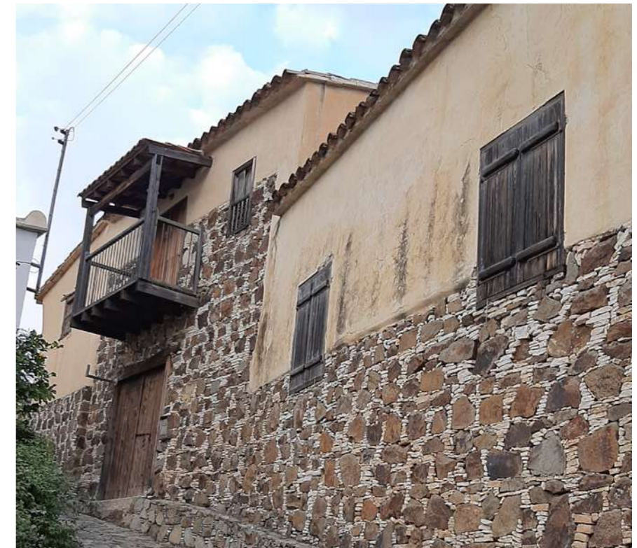
Fig.24-25: Interior and Exterior view of the dwelling after restoration. © M. Philokyprou
