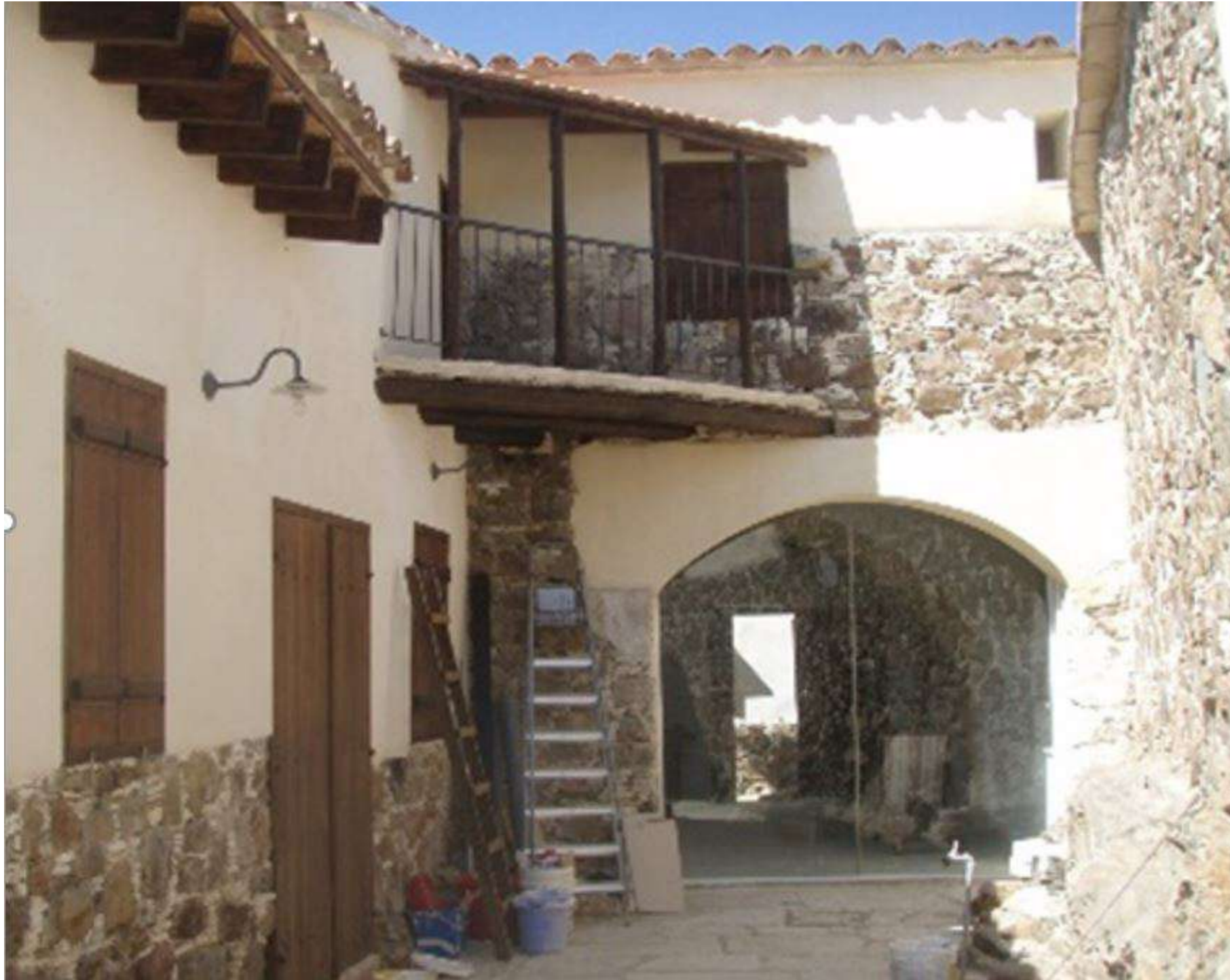
Fig.26: Views of the vernacular dwelling from the central yard after the restoration, showing the triangular balcony and the closing of the arch of the iliakos with frameless glass. © M. Philokyprou
