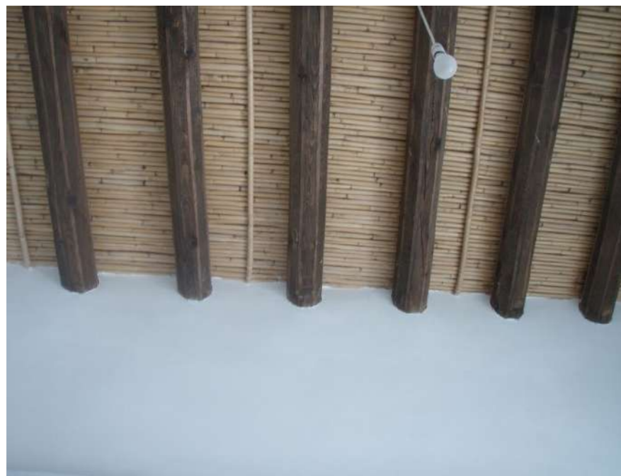
Fig.9: Maintenance of the original traditional materials. © M. Philokyprou
