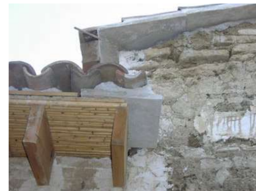
Fig.17-18: Timber roof details. © M. Philokyrou
