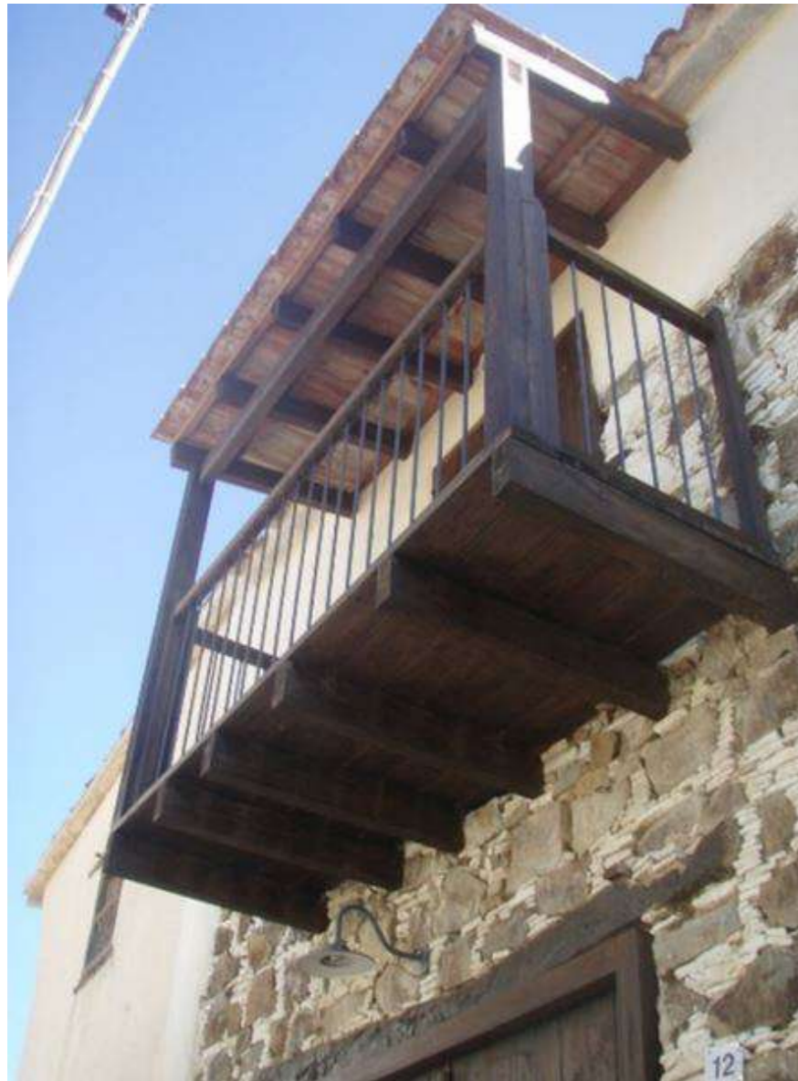
Fig.32: View of the balcony towards the street after restoration. © M. Philokyprou
