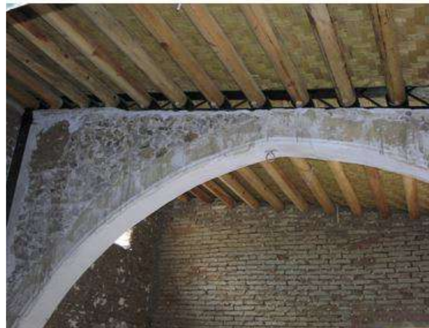
Fig.10: Maintenance of the original traditional materials, and use of a metal structure above the main arch of dichoro. ©M. Philokyprou
