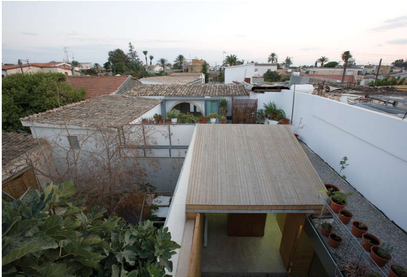
Fig.12: Roof View of the completed intervention. © Y. Hadjichristou
