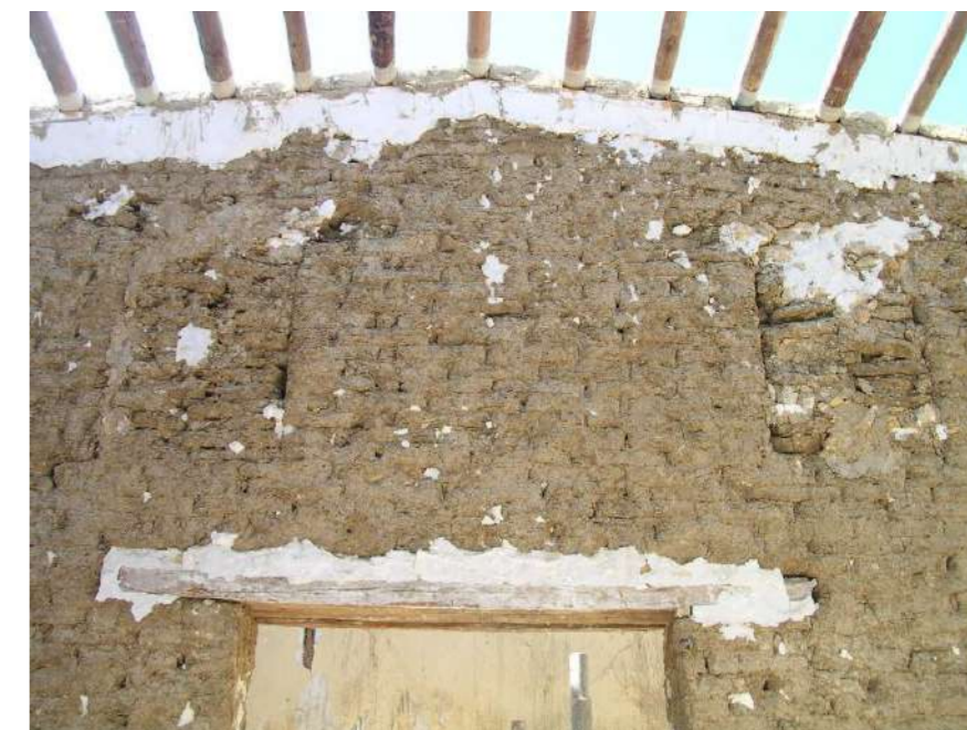
Fig.11: Finding the traces of the arseras, the upper windows for cross ventilation. © Y. Hadjichristou
