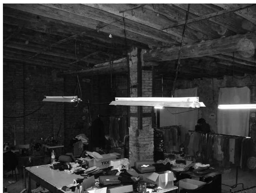
Fig.3: View of the existing conditions in the interiors of the buildings. © Taller 9s Arquitectes
