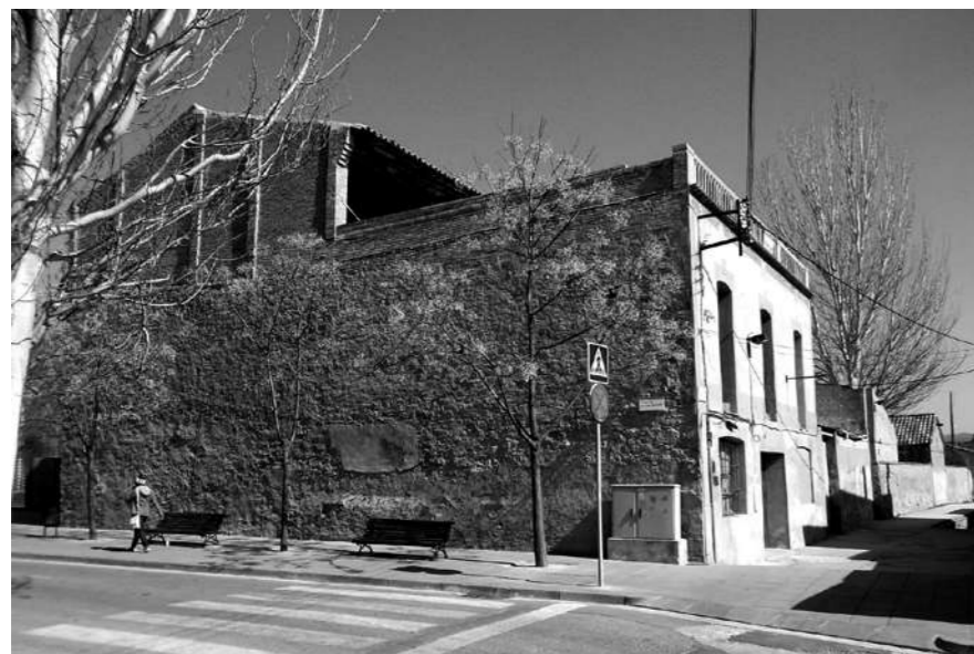
Fig.2: View of the existing conditions of the buildings' exteriors from the main street. © Taller 9s Arquitectes
