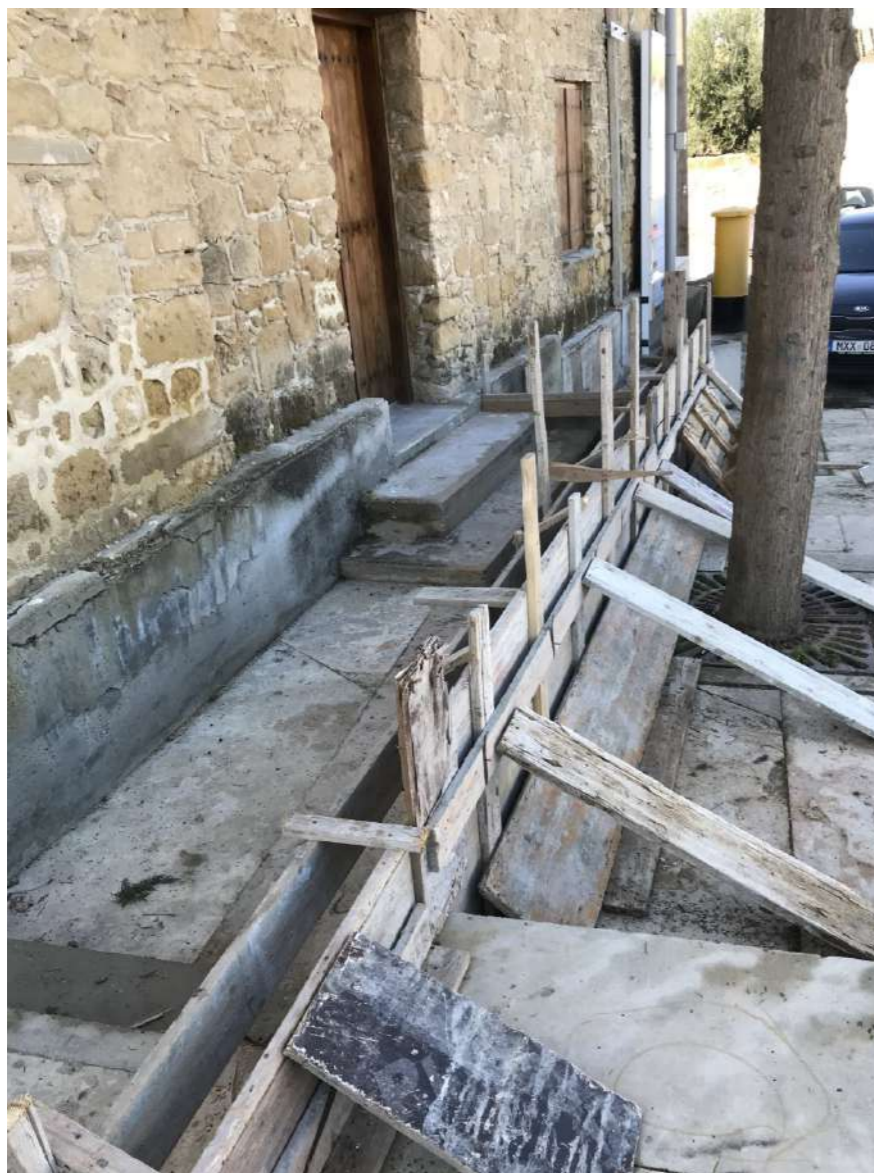
Fig.28-29: Construction of accessible routes for the building. © FOSS Research Centre for Sustainable Energy / University of Cyprus
