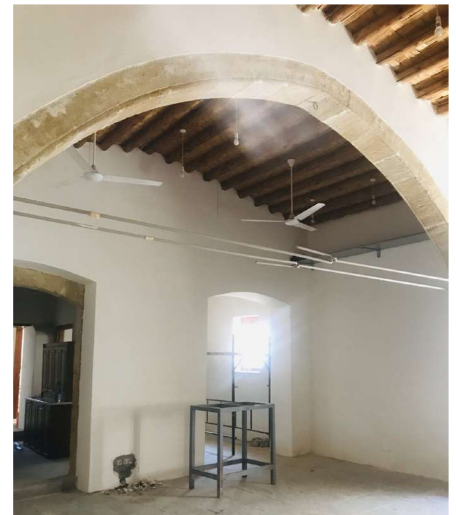
Fig.8: Interior view of the central space – double space room (dichoro). © FOSS Research Centre for Sustainable Energy / University of Cyprus
