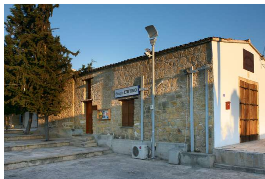
Fig.1: Exterior views of the building before conservation. © FOSS Research Centre for Sustainable Energy / University of Cyprus
