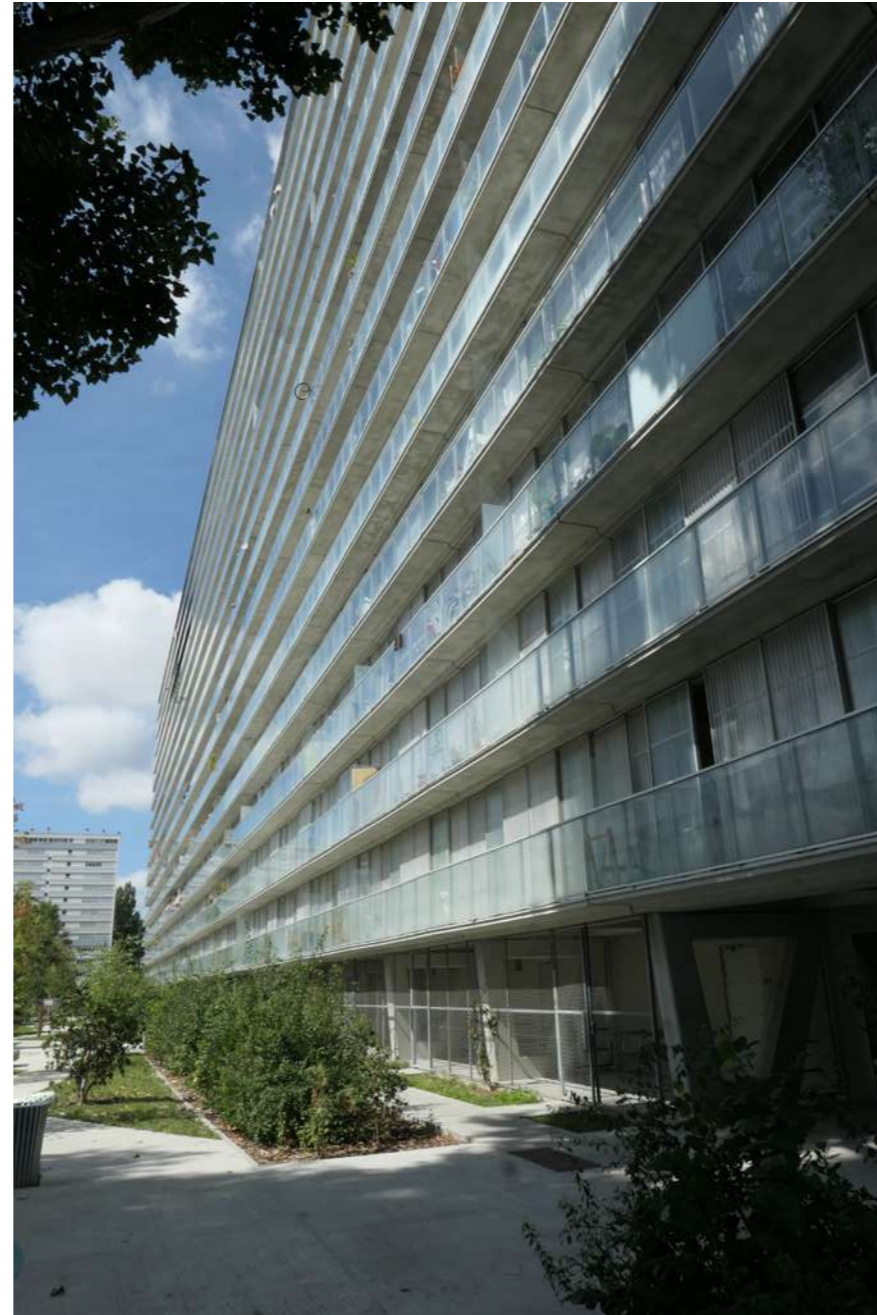
Fig.24: View of transformed façade and renovated exterior landscape.
