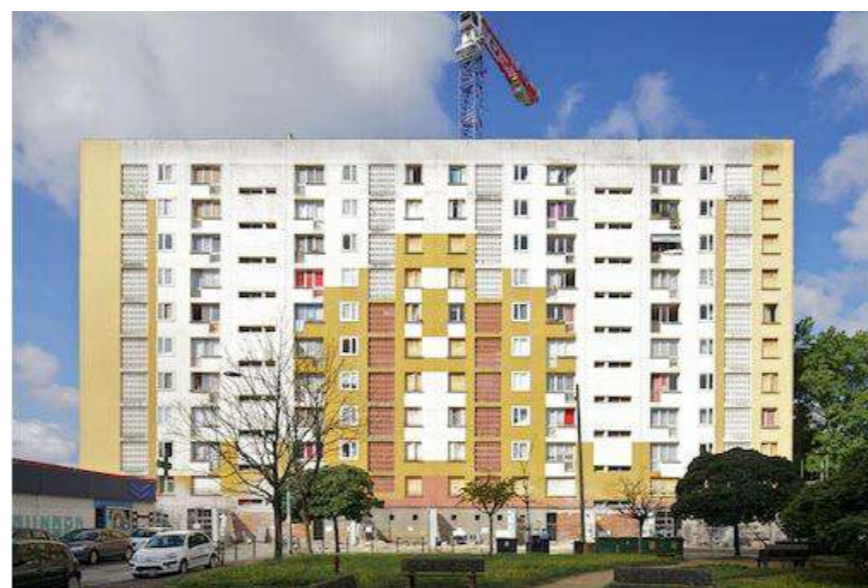
Fig.1: Building G before the renovation. © Philippe Ruault.
