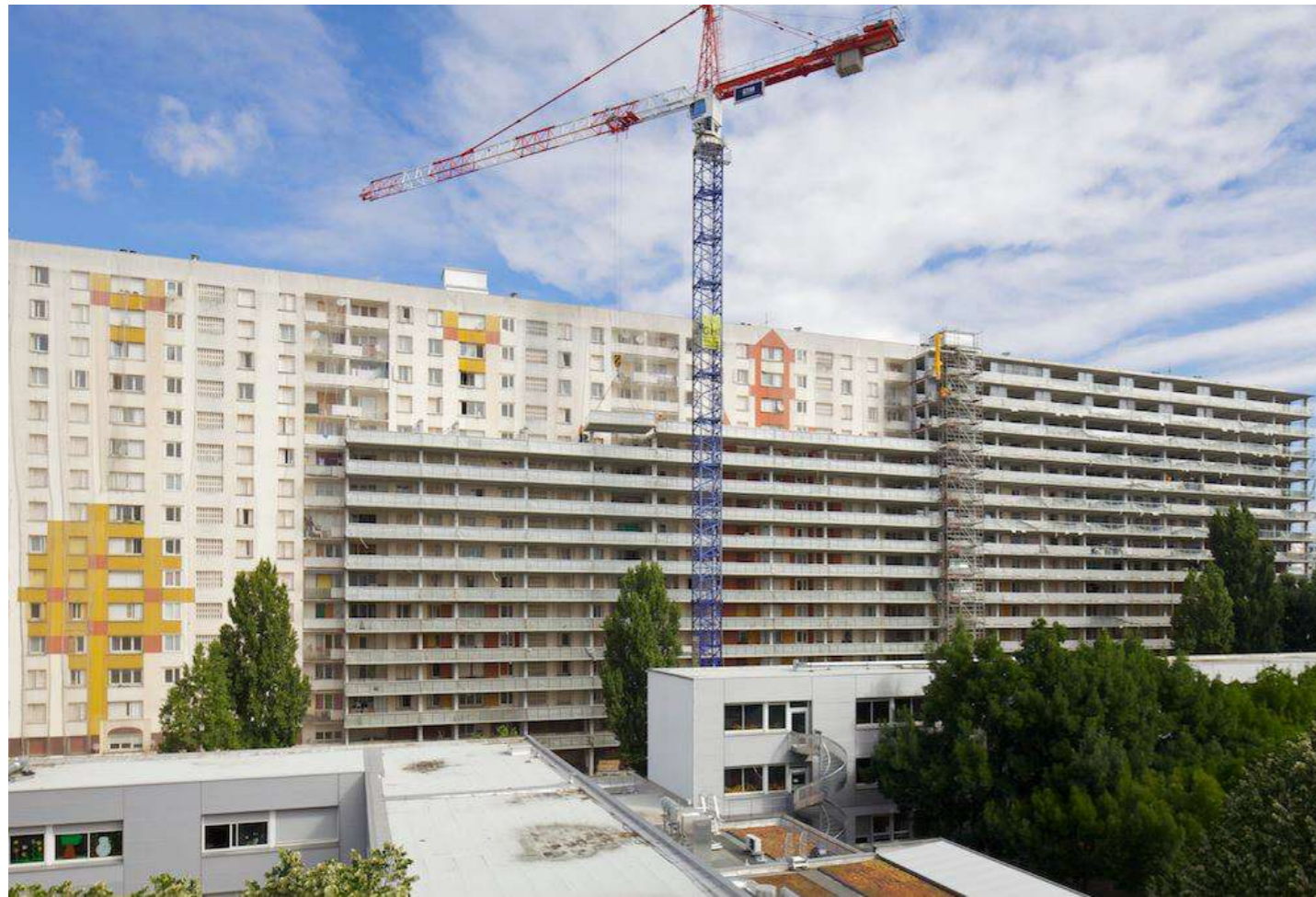
Fig.19-20: Construction process, installation of pre-fabricated elements over the existing buildings.. © Philippe Ruault.
