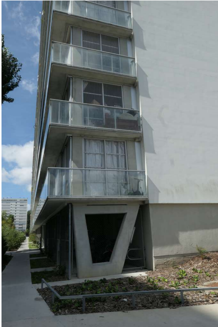
Fig.23: Detailed view of the extension's base structure.
