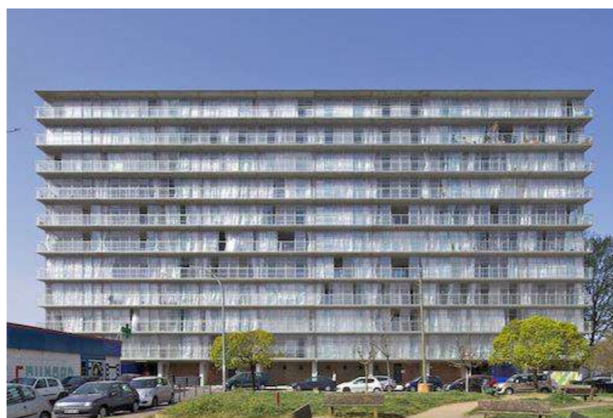
Fig.2: Building G after the renovation. © Philippe Ruault.
