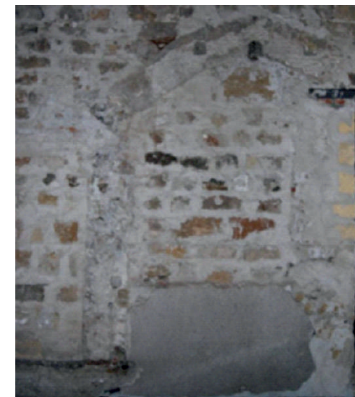
Fig.20: Crowning's examples of openings embedded in masonry at different levels. © Arch. Francesco Miceli
