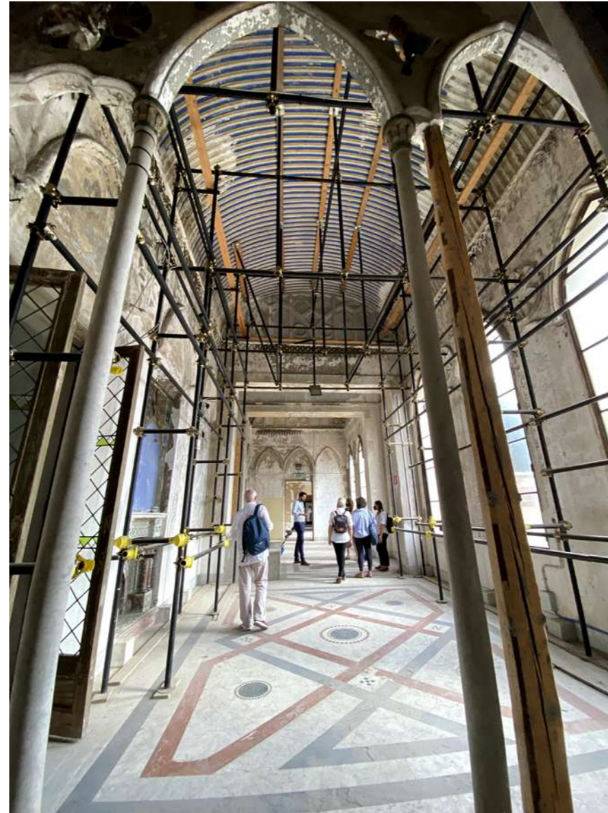
Fig.30: Interior space, waiting for restoration. © Luisa Lombardo
