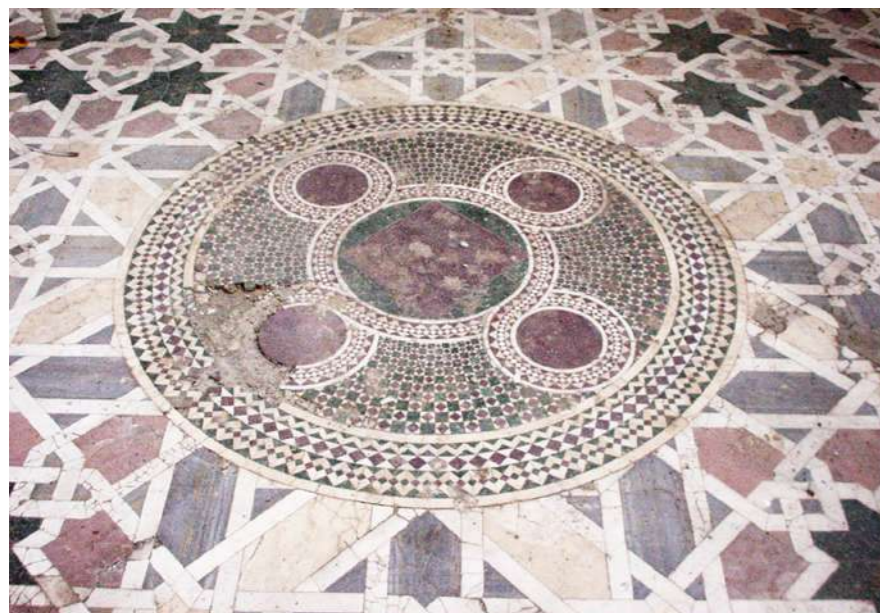
Fig.6: Detail of the paving of same Representative hall, today © Project Designersigliano, and ANCE Palermo Staff; Detail of internal wall decoration. © Francesco Renda
