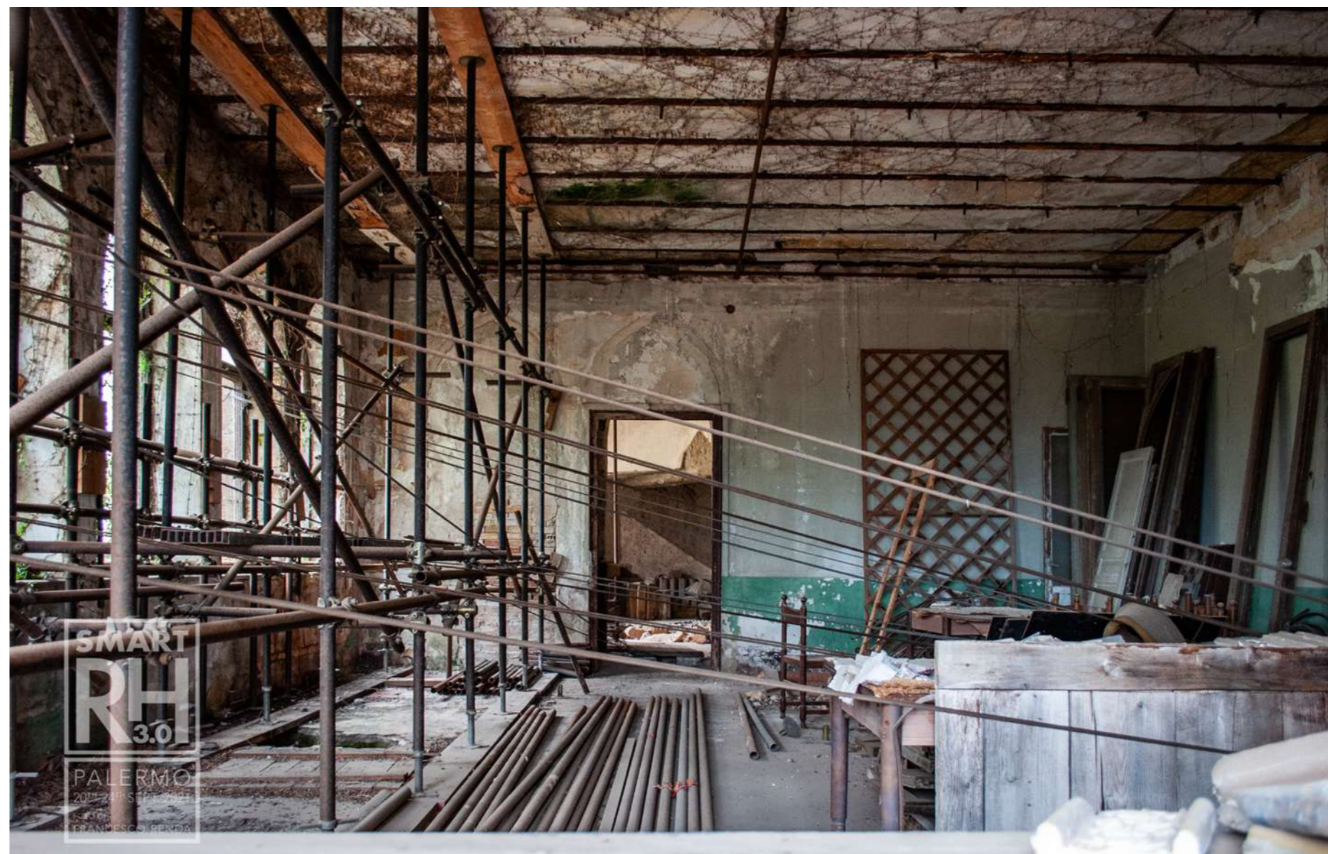
Fig.25: Interior space, waiting for restoration. © Francesco Renda
