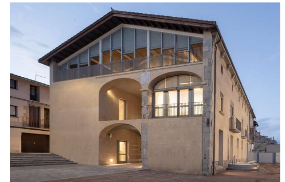
Fig.5: Rehabilitated south façade.
