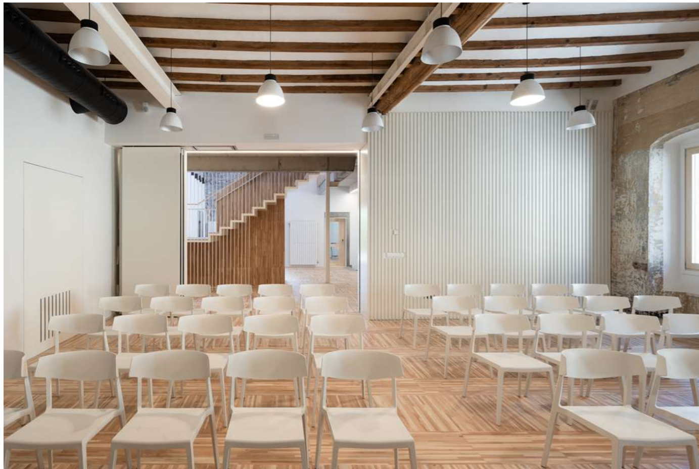
Fig.14-15: Multipurpose room: Noble room on the first floor with preserved and reinforced slab of wooden joists and interior facing of the original facade.
