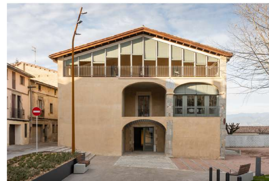
Fig.3: Before and after of the main façade.
