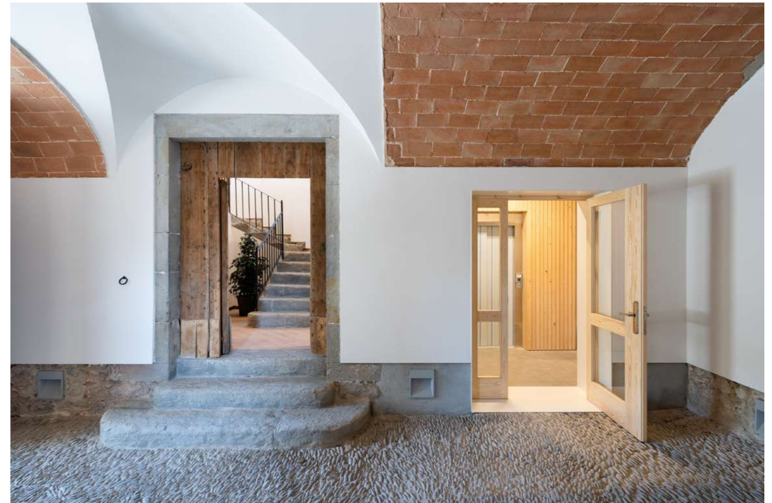
Fig.12: Interior entrance: Lobby closed on the ground floor, with double access and restored original construction elements (round pebble paving and ceramic vault).
