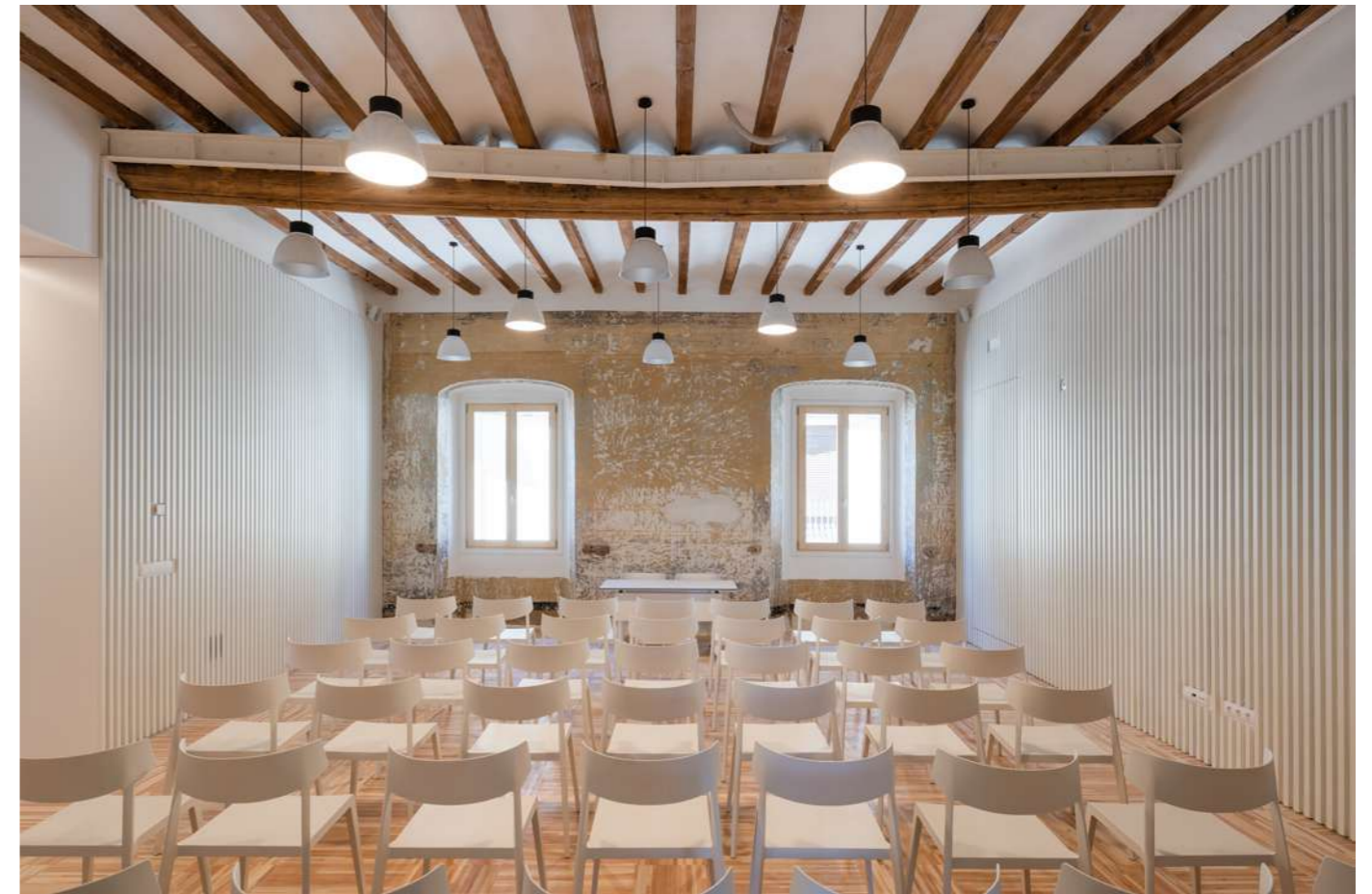
Fig.14-15: Multipurpose room: Noble room on the first floor with preserved and reinforced slab of wooden joists and interior facing of the original facade.
