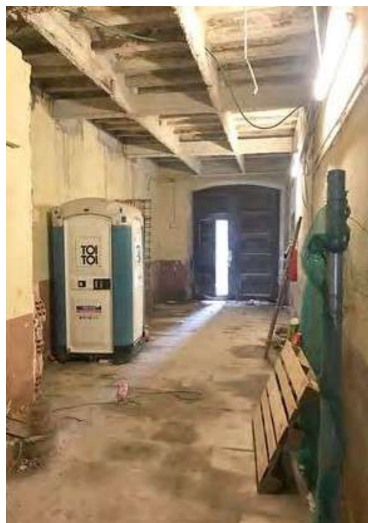
Fig.4: View of the existing entrance hall. © Juli Pérez-Catalá Arquitectura
