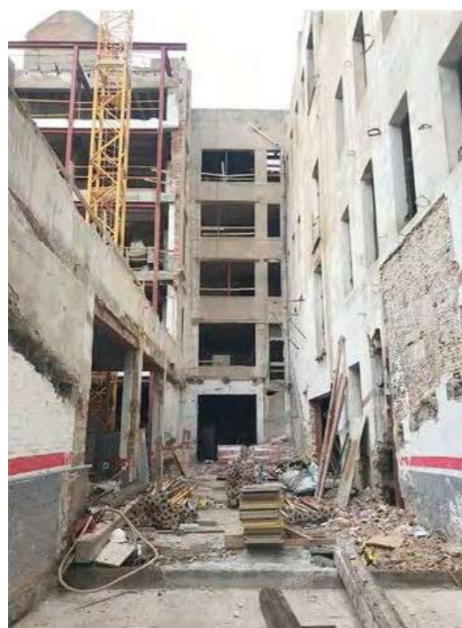
Fig.9-10: Views of the existing conditions in the courtyards. © Juli Pérez-Catalá Arquitectura
