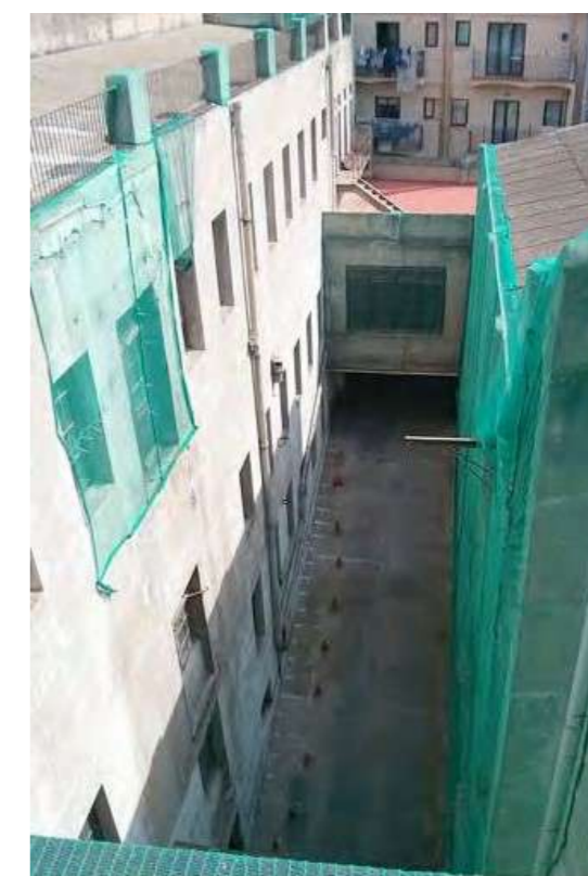
Fig.7-8: Views of the existing conditions in the courtyards. © Juli Pérez-Catalá Arquitectura
