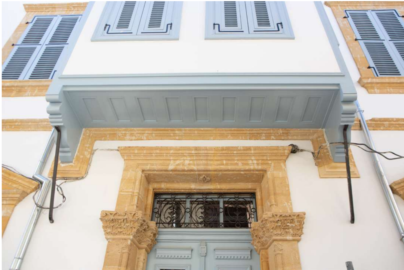
Fig.20: Exterior view of the building after restoration. © Simos Drousiotis/A. M. Andronicou Ltd
