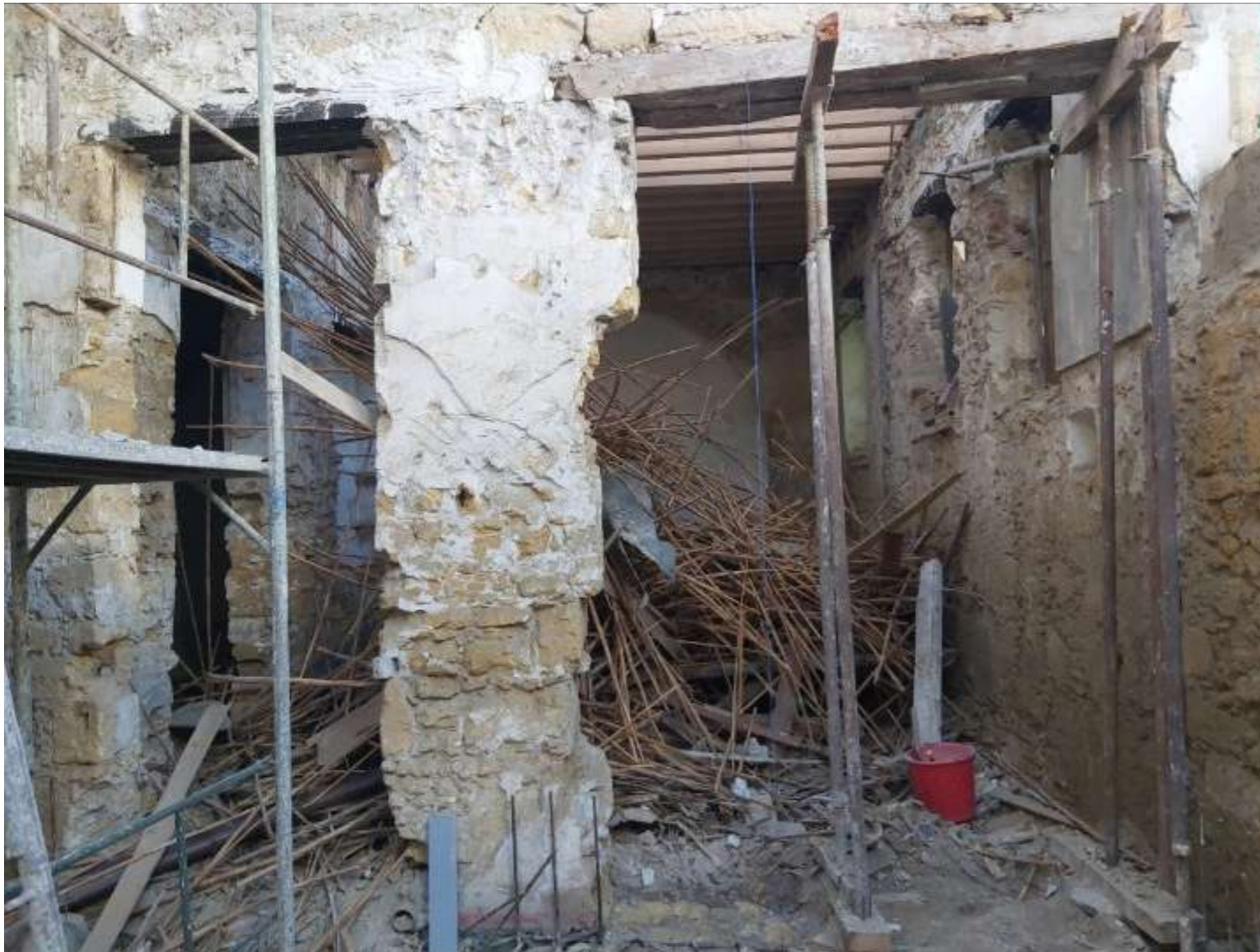
Fig.16: Views of the building during conservation. © Simos Drousiotis/A. M. Andronicou Ltd
