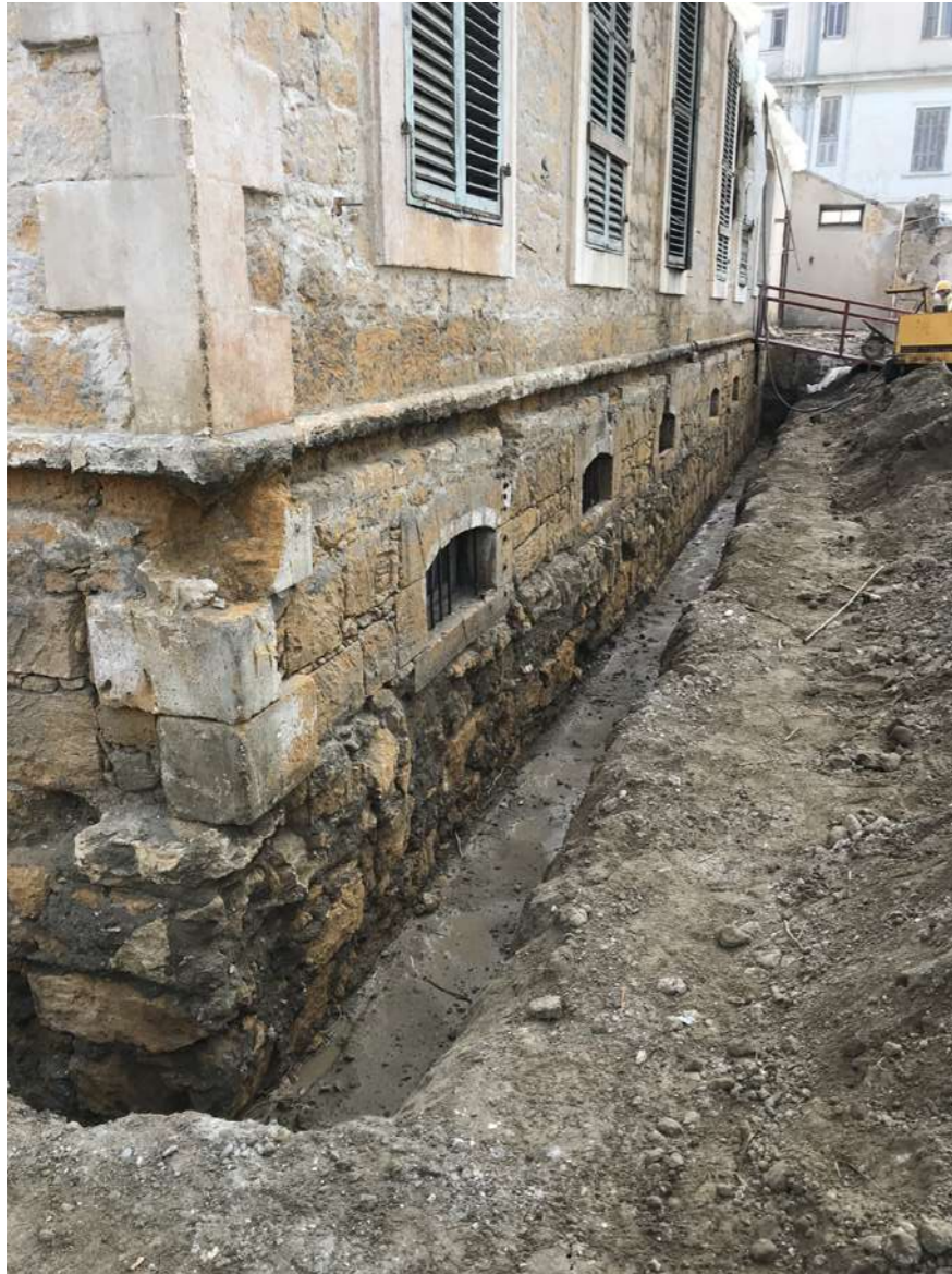
Fig.30-32: Construction phase pictures and details – Drainage system and insulation installation. © C. Marathovouniotis
