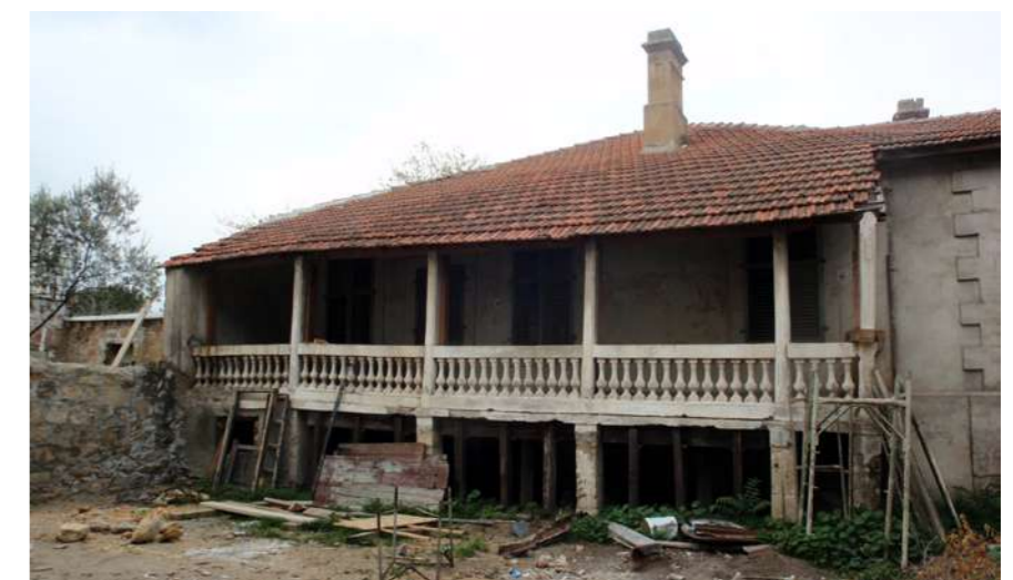
Fig.6-7: General view of the building. © C. Marathovouniotis
