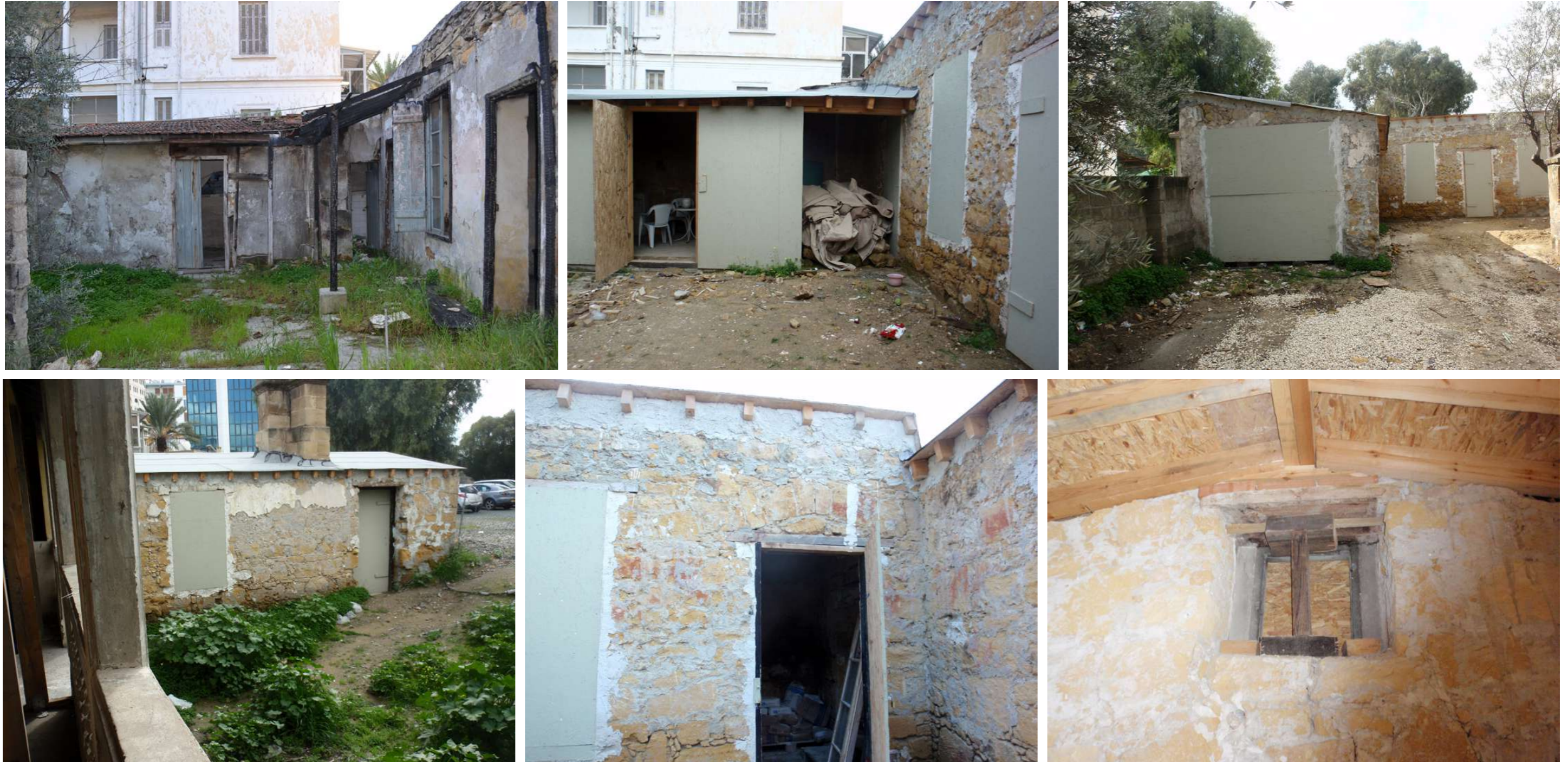
Fig.58-63: Construction phase pictures – Auxiliary buildings restoration and renovation. © C. Marathovouniotis
