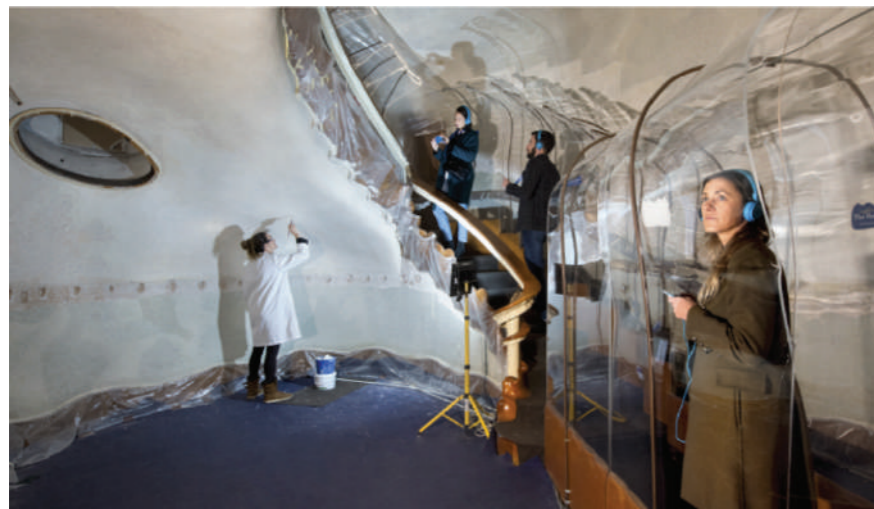
Fig 10.1. Screen adapted for spaces to protect but also allow the visitor to see during the restoration process. Oscar Criado - Archivo Casa Batlló
