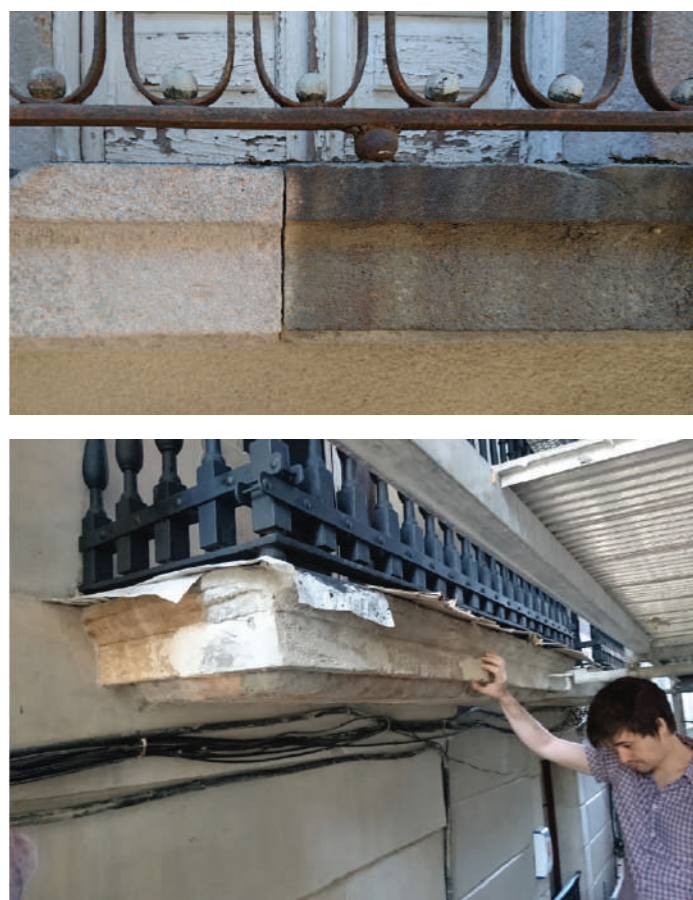
Fig.4-5: Process of the restoration and cleaning of the balconies.
