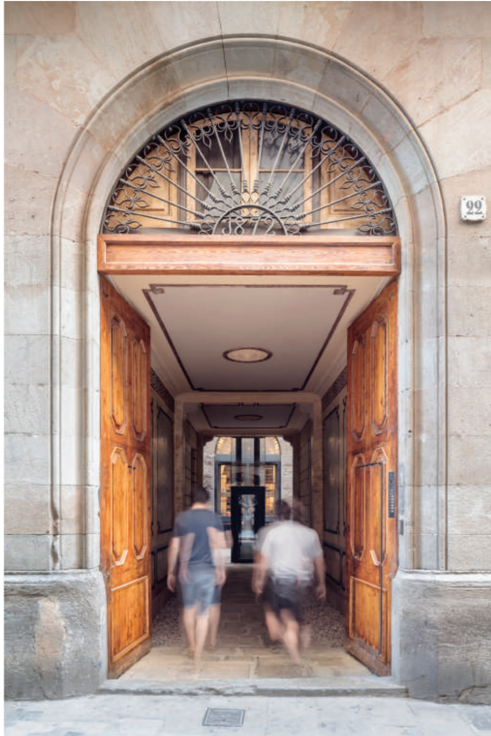
Fig.20: View of the main entrance.
