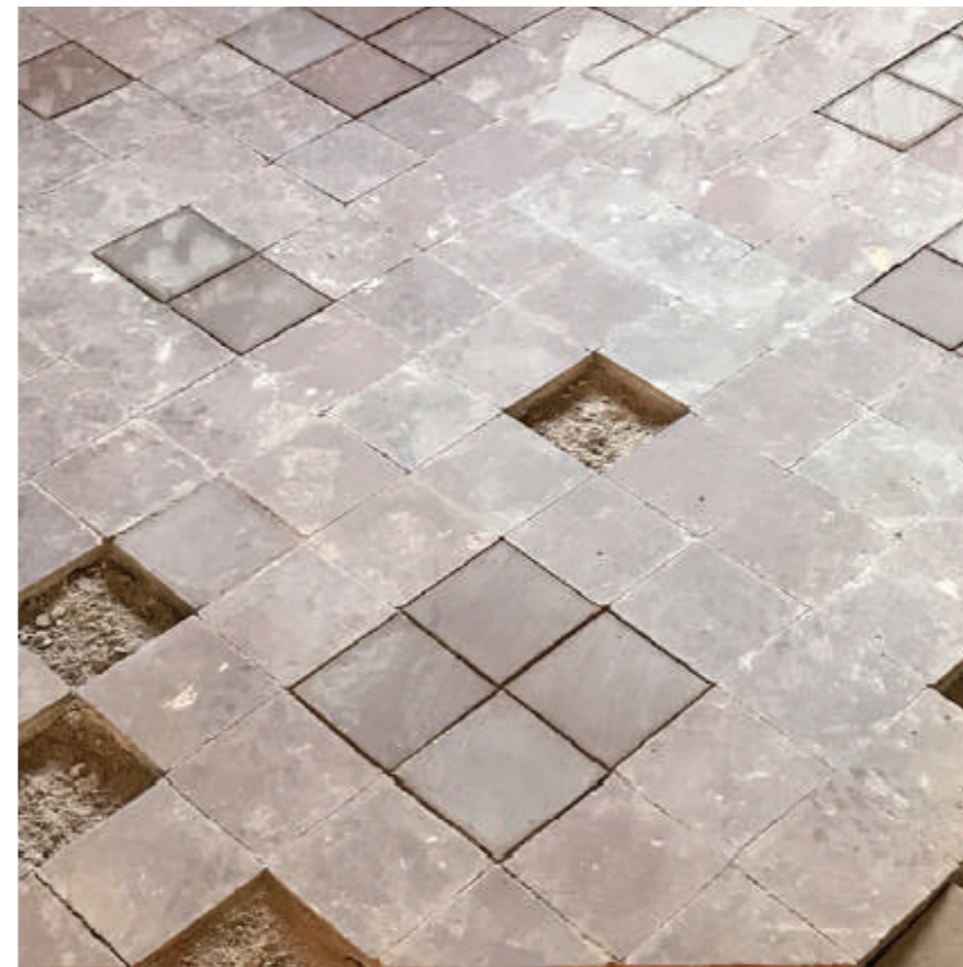
Fig.8: Recovery process of the original interior pavement.
