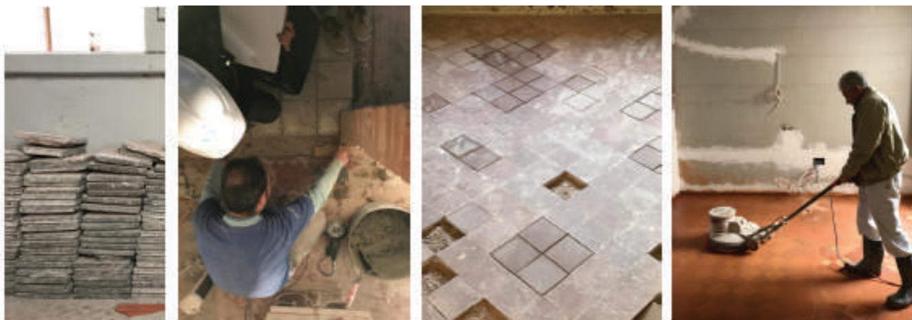
Fig.13: Restoration / recovering of the pavements.
