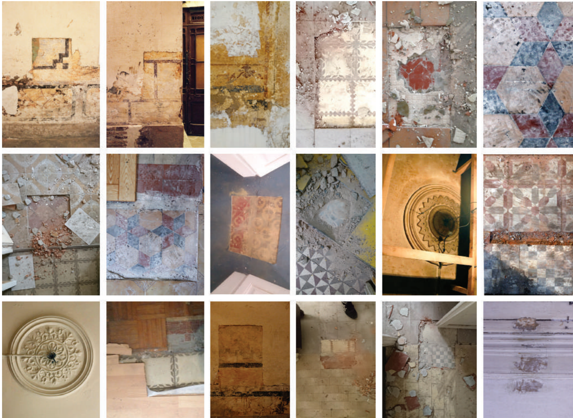
Fig.11: Exploratory test-holes to discover the original elements hidden underneath later interventions.
