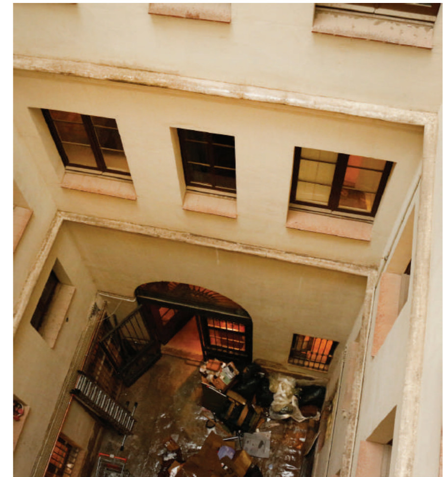
Fig.3: View of courtyard, before the intervention.
