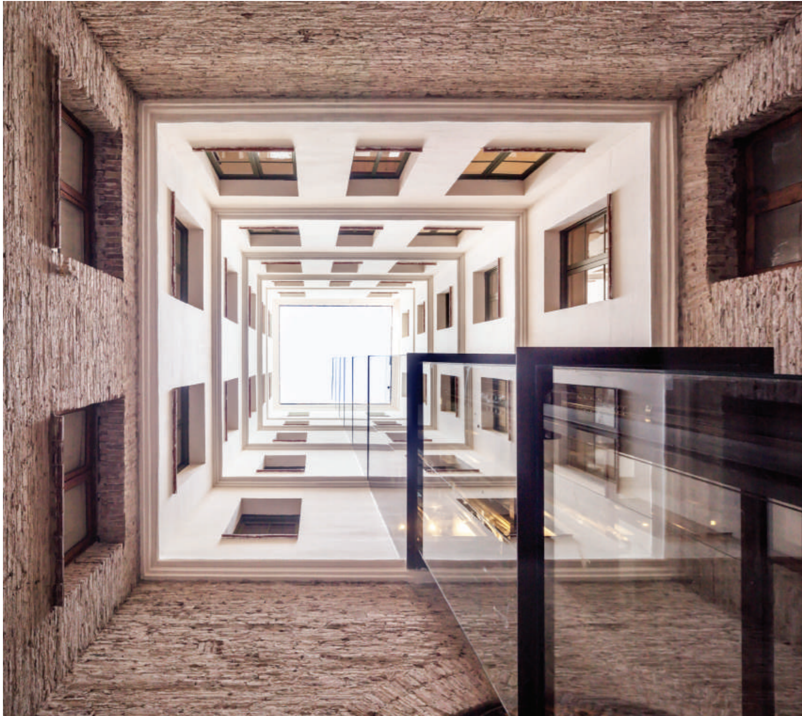
Fig.24: View of the new elevator as it “vanishes” through its surroundings.
