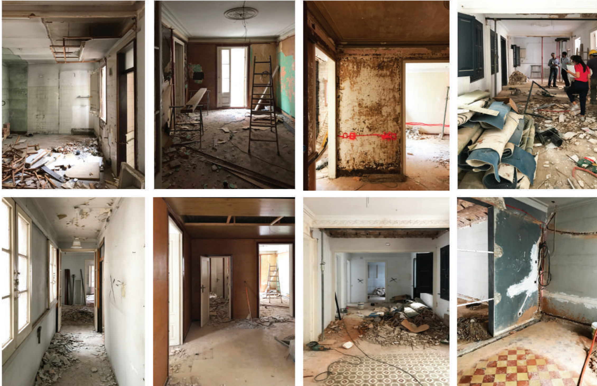
Fig.12: Removal of the modern interventions that cover the historical elements.
