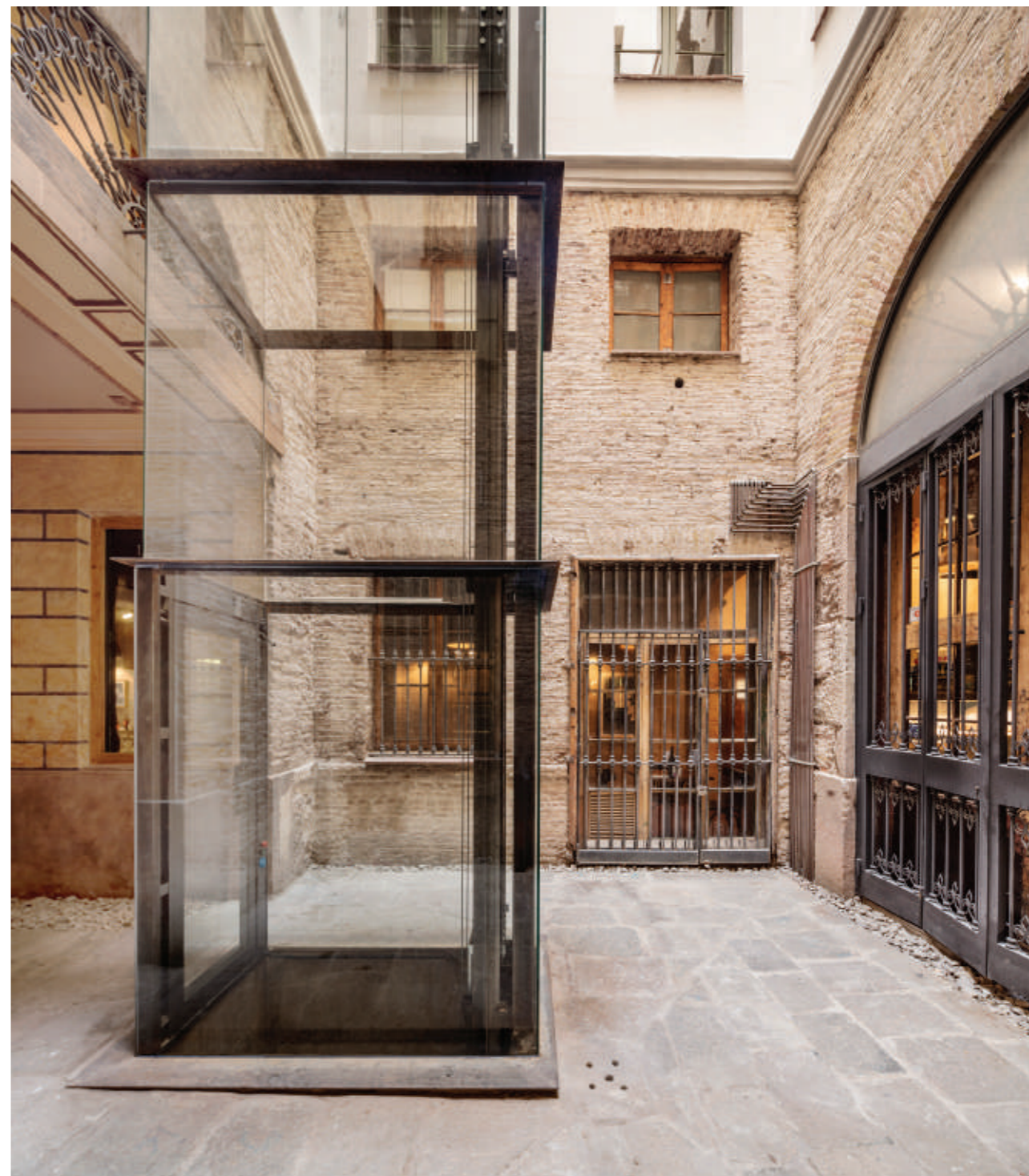
Fig.23: View of the courtyard and new elevator structure.
