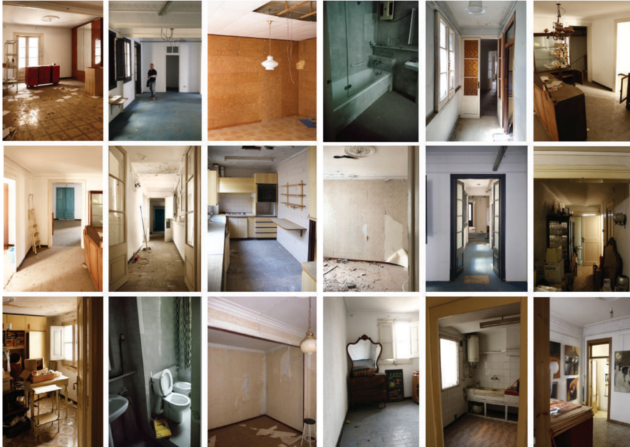
Fig.10: Existing conditions of the dwellings.
