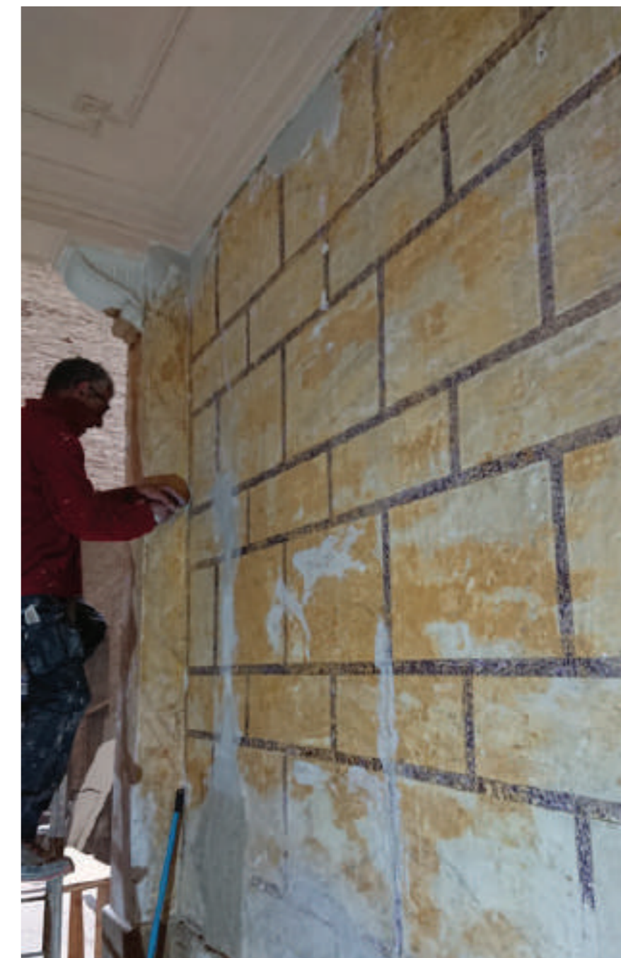
Fig.6: Restoration of the stuccoes of the interior passage.
