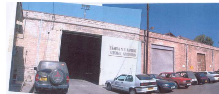
Fig.36: Original condition with traffic access. © Kristian Christou Architects, A. J. Brooks, Architect.
