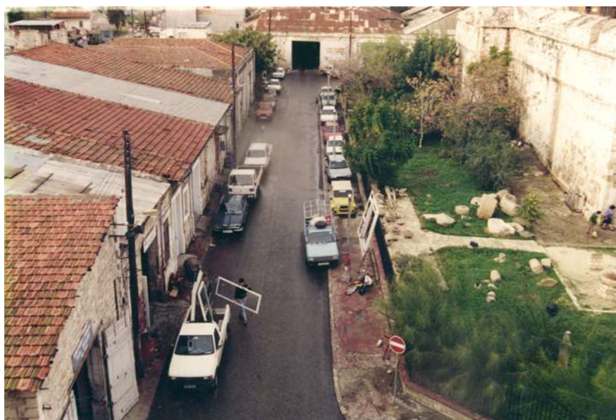
Fig.33: Approach road to Carob Mill before. © Kristian Christou Architects, A. J. Brooks, Architect.
