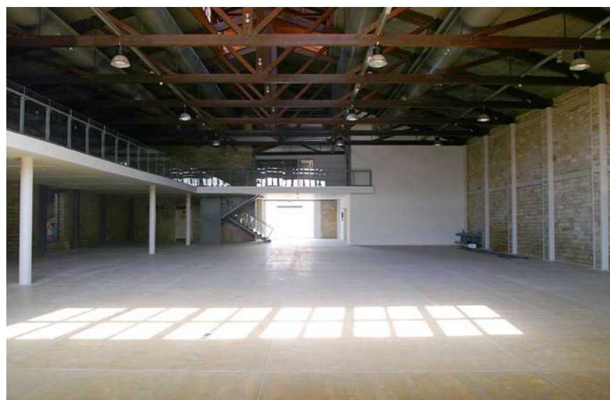
Fig.2: In the North hall, central, free-standing concrete columns and metal trusses were removed and replaced with single span timber laminated trusses with no intermediate support. © Kristian Christou Architects, A. J. Brooks, Architect.
