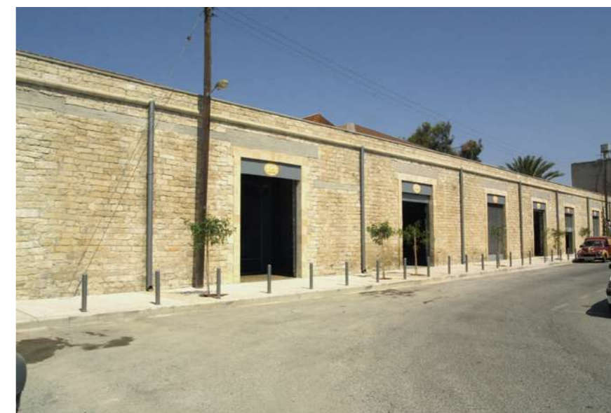
Fig.37: After restoration with traffic access. © Kristian Christou Architects, A. J. Brooks, Architect.
