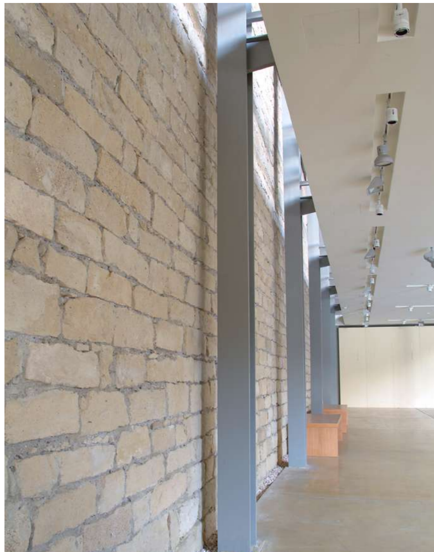
Fig.5: View of the rehabilitated interior with new interventions. © Kristian Christou Architects, A. J. Brooks, Architect.
