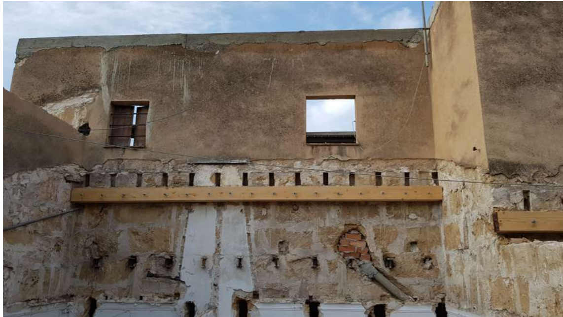
Fig.34: Works on roofs.
