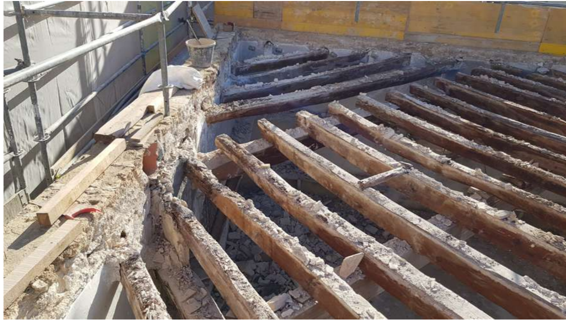
Fig.26: Wooden Floor Slabs.
