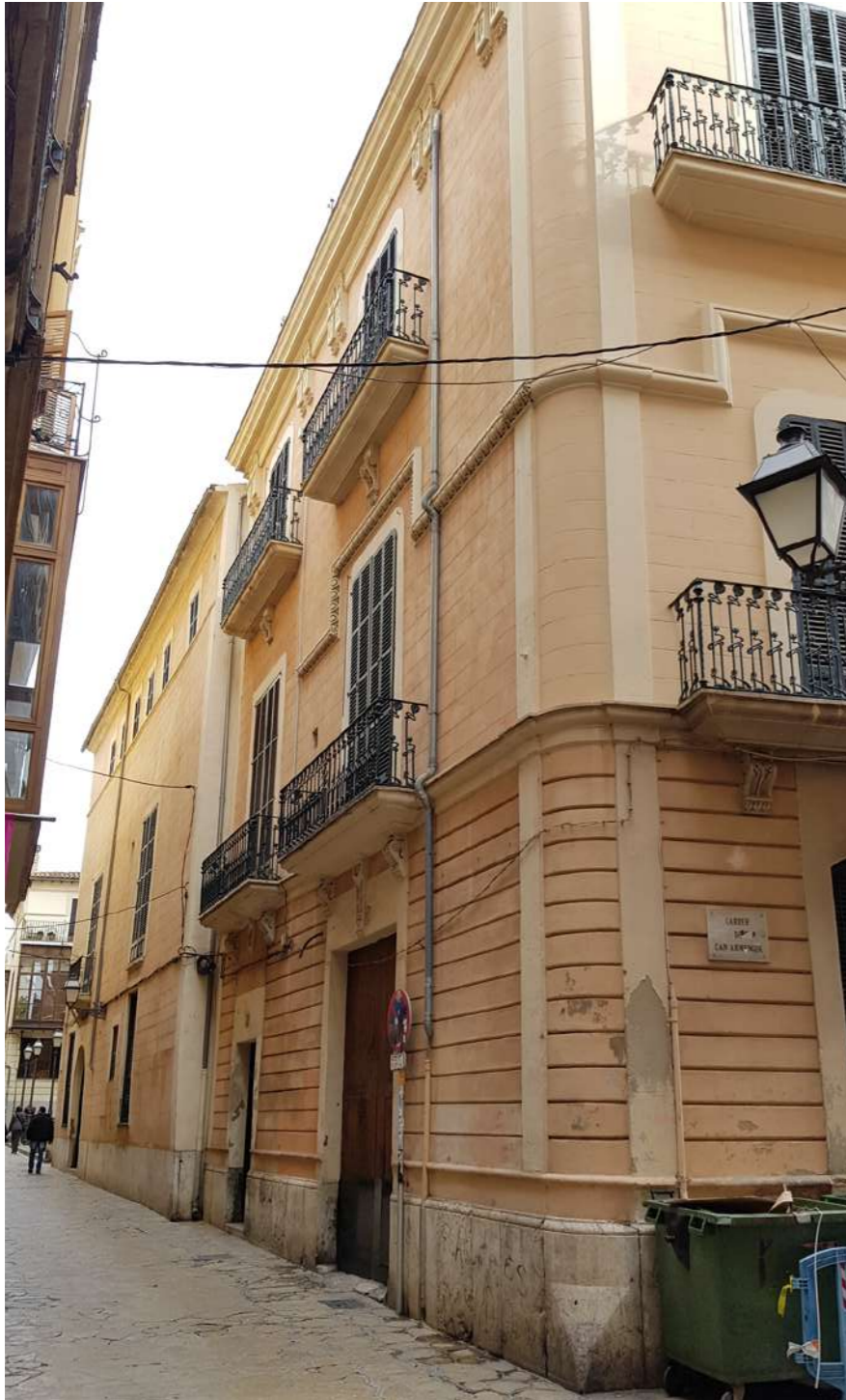
Fig.12: Initial state Main façade
