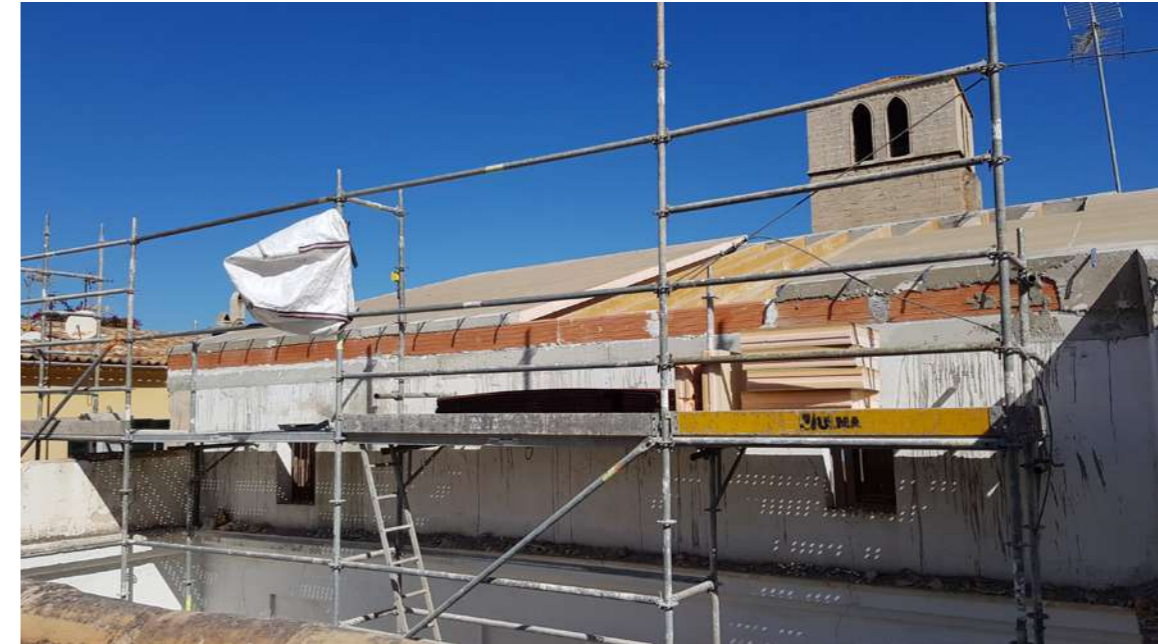
Fig.36: New roofs' thermal insulation.
