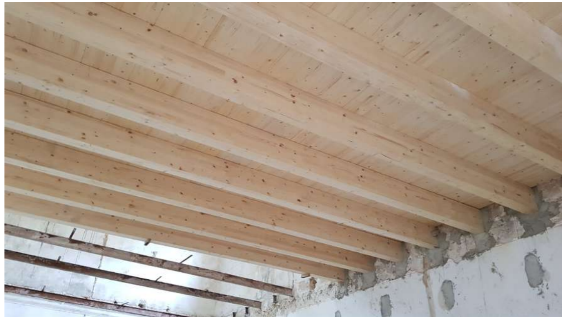
Fig.42: New laminated wooden floor slab.
