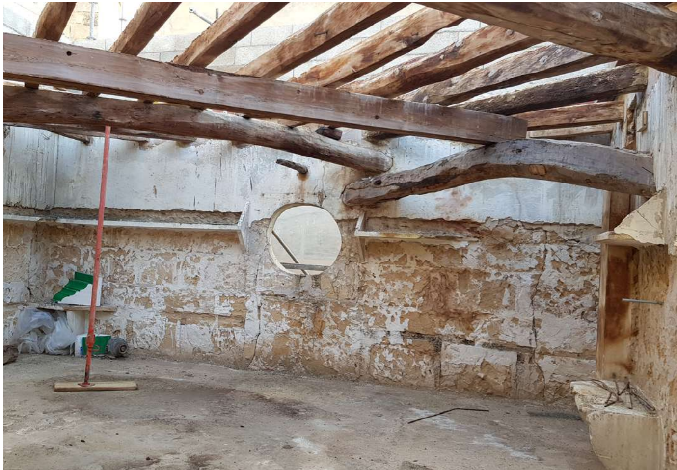
Fig.15: Marés stone load-bearing walls and wooden beams. Initial state.
