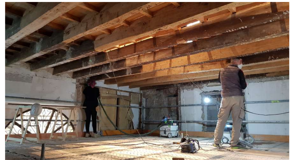
Fig.41: Existing wooden floor slab under restoration.
