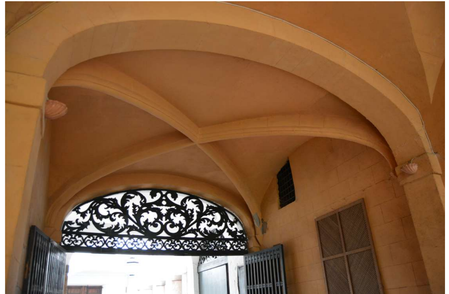
Fig.16: Marés stone vault, arches, and walls. Initial state.
