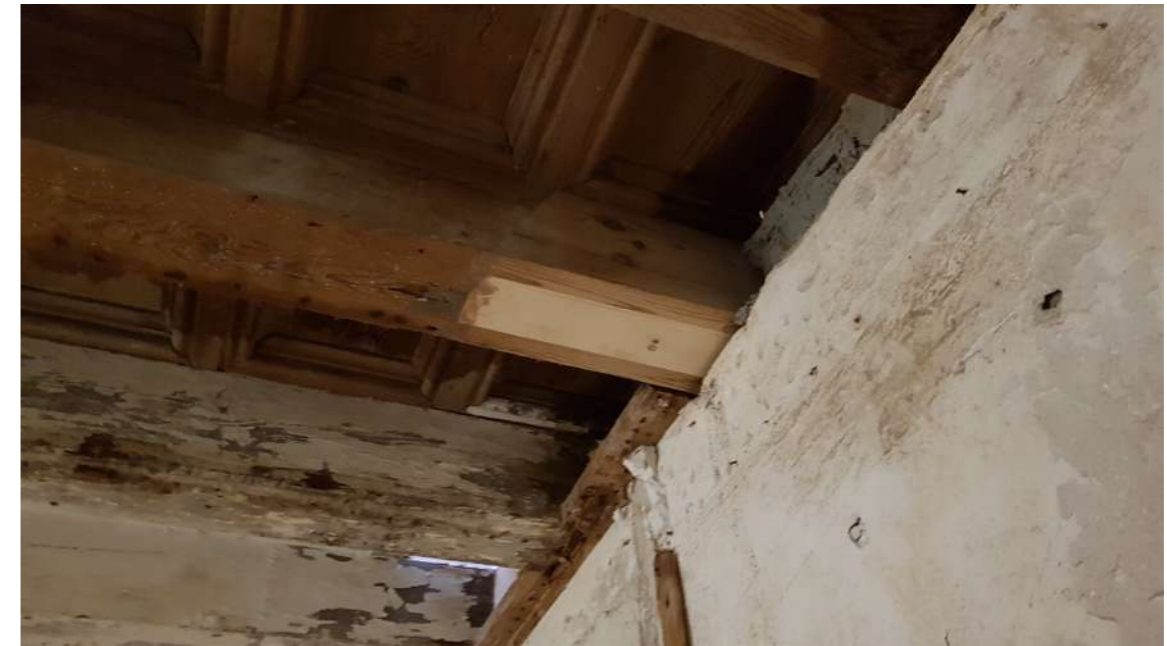
Fig.40: Reinforcement of ancient wooden beam.
