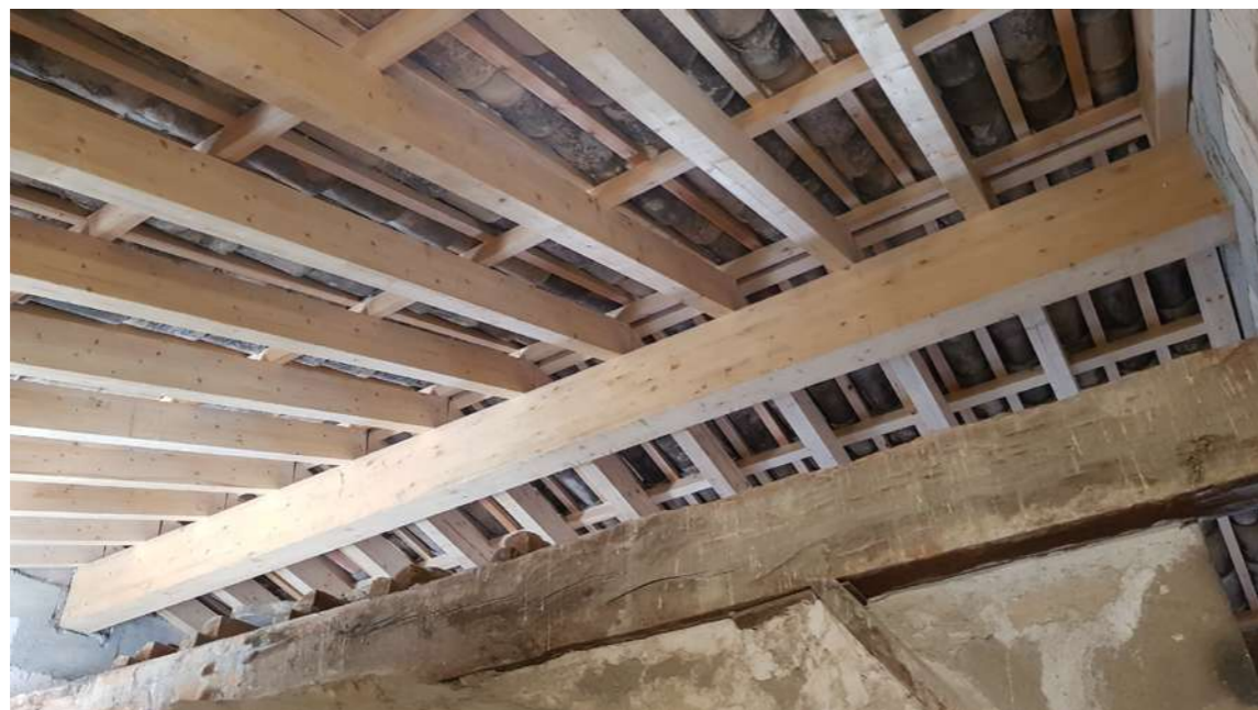
Fig.39: New laminated wood structure covered with ancient ceramic roof tiles.
