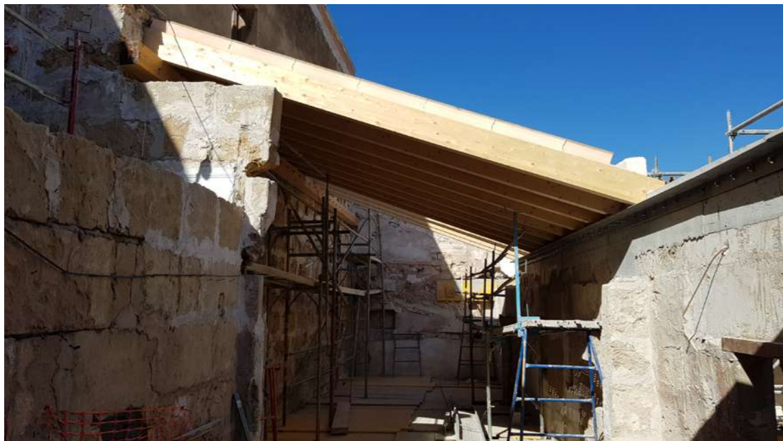
Fig.35: New laminated wood beams.
