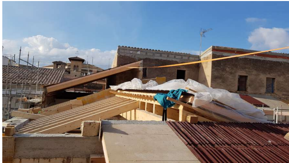
Fig.38: Works on different roofs.
