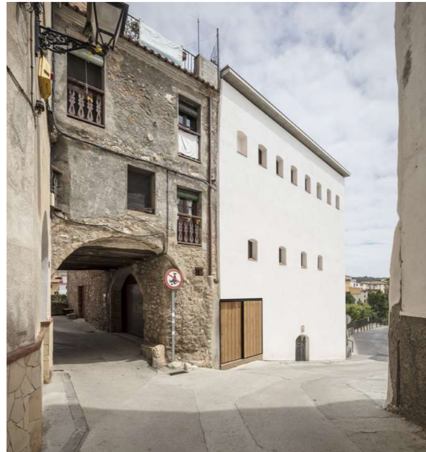
Fig.4: View of one of the side façades, and neighboring buildings.
