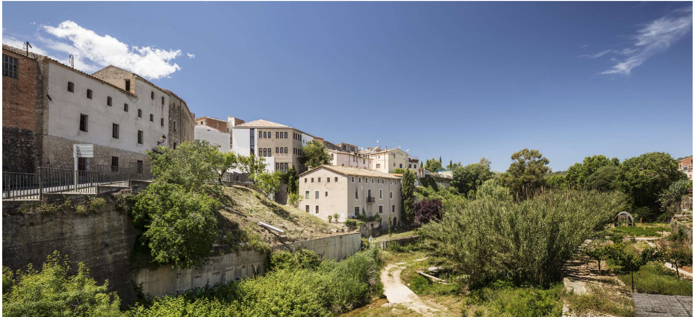
Fig.8: View of the the rehabilitated complex blending with the historical city and landscape.
