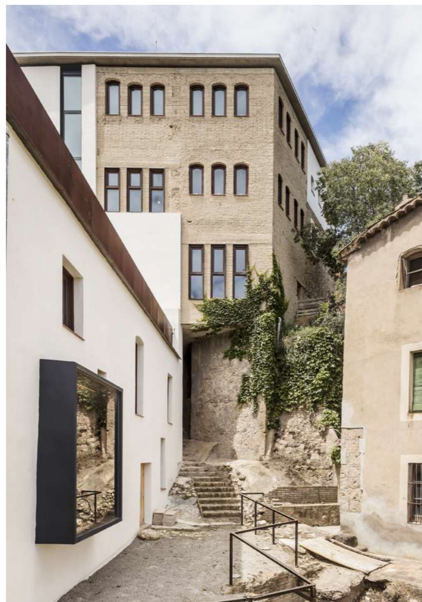
Fig.1: View of the rehabilitated complex.
