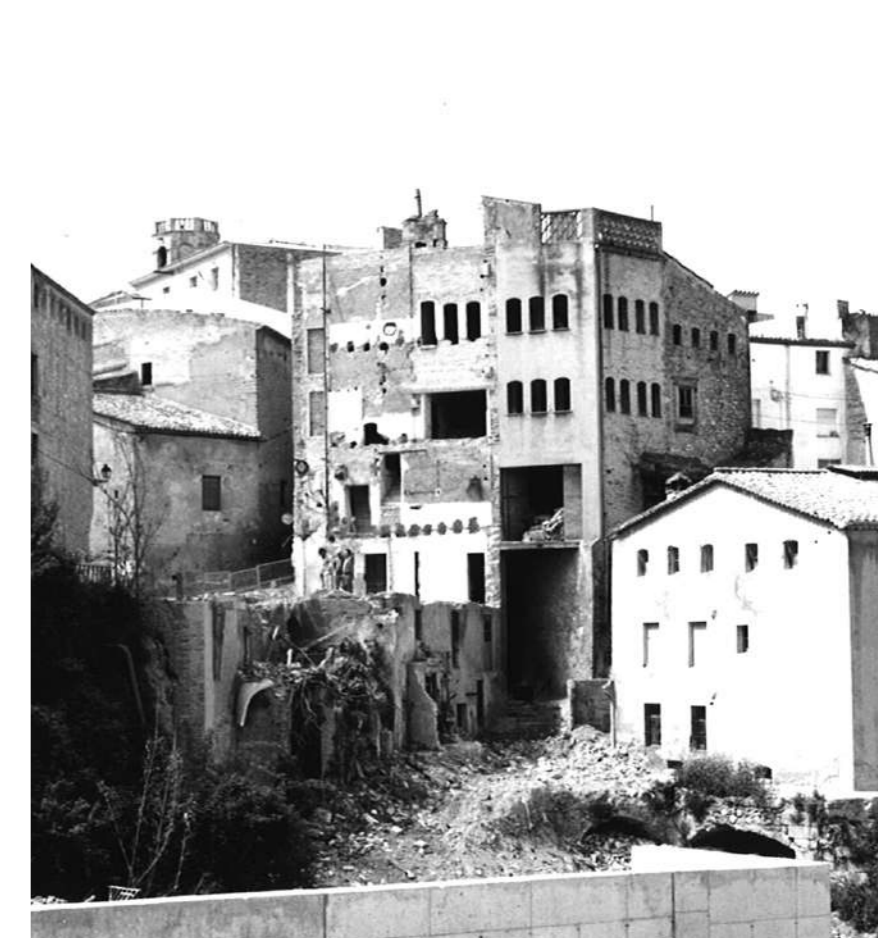
Fig.2: View of the existing conditions prior to the intervention.
