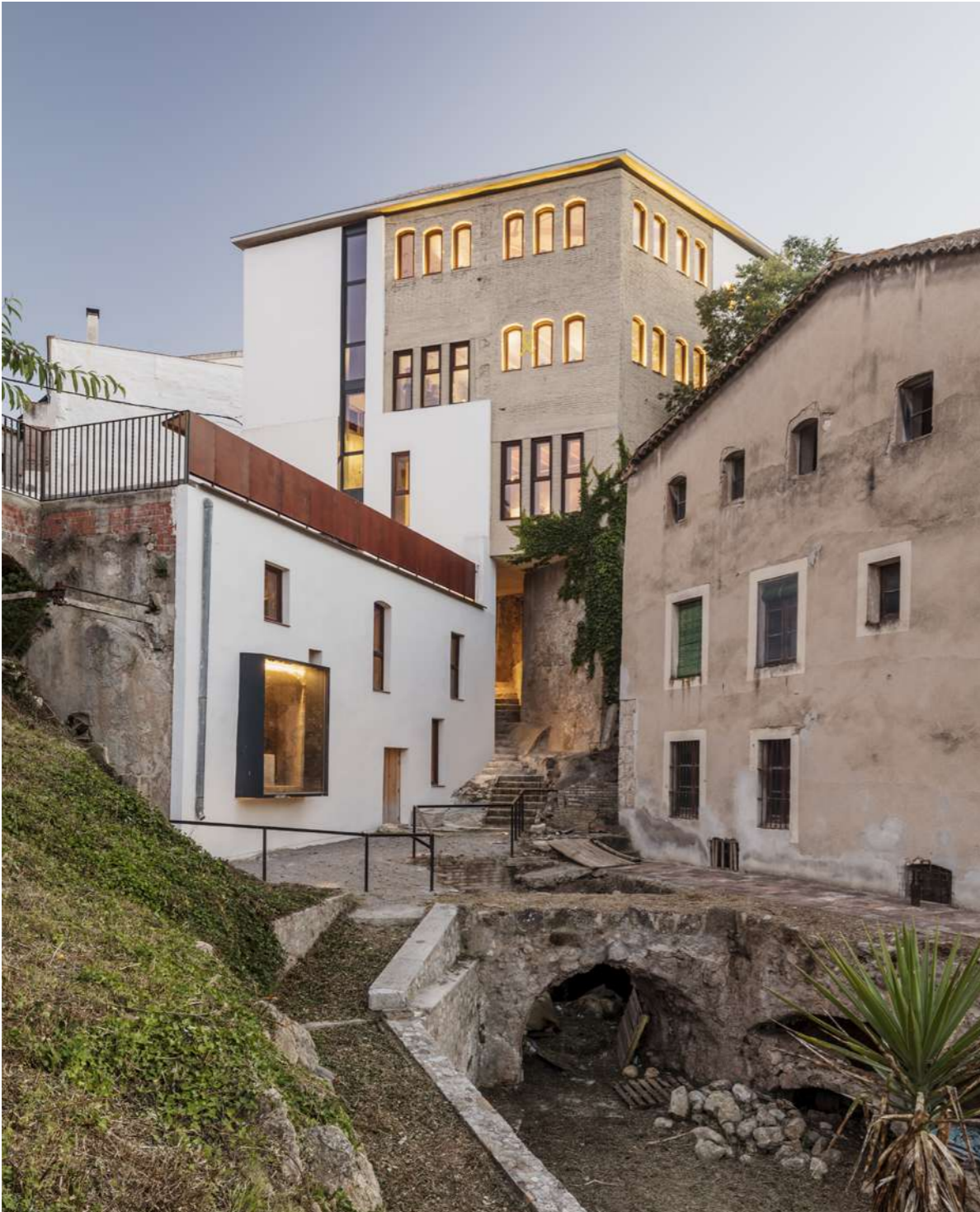
Fig.9: View of the the rehabilitated complex from the lowest part of its site.
