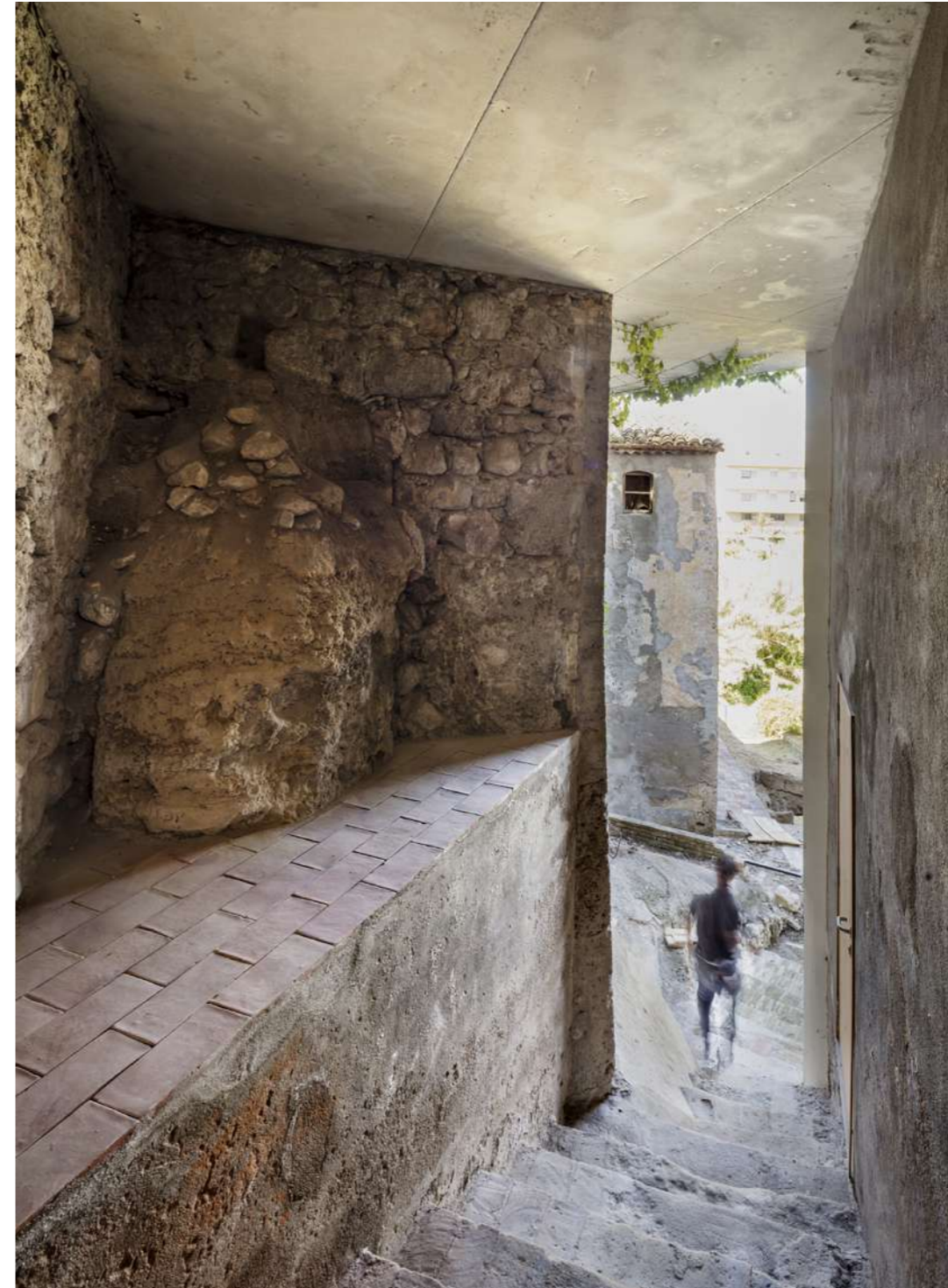
Fig.10: View of a passage that runs through the rehabilitated building.
