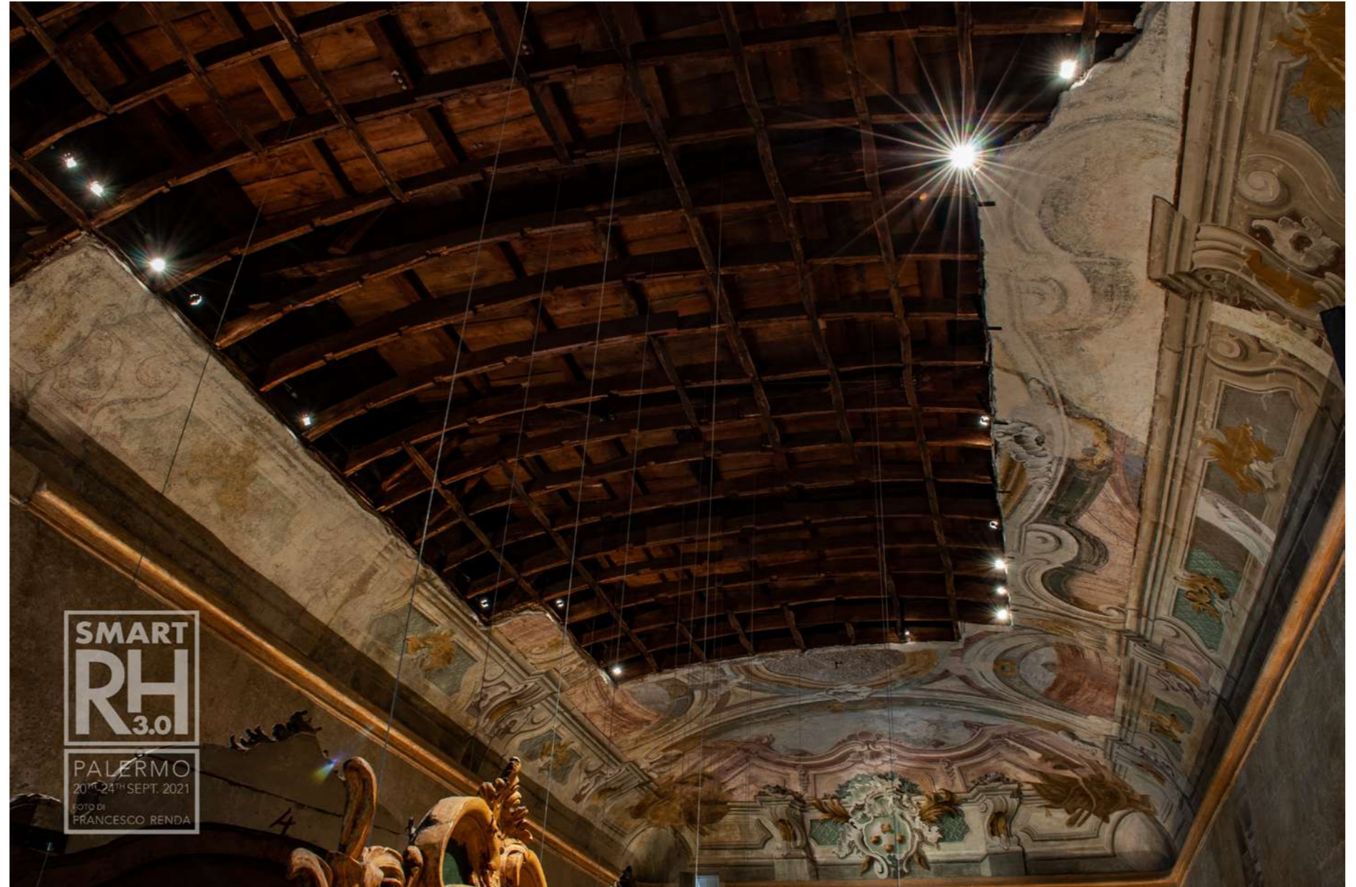
Fig.24: Restoration of a great wooden vaulted ceiling, without completing intrados plaster finishing, but with the centering and listel structure left on sight. © Francesco Renda
