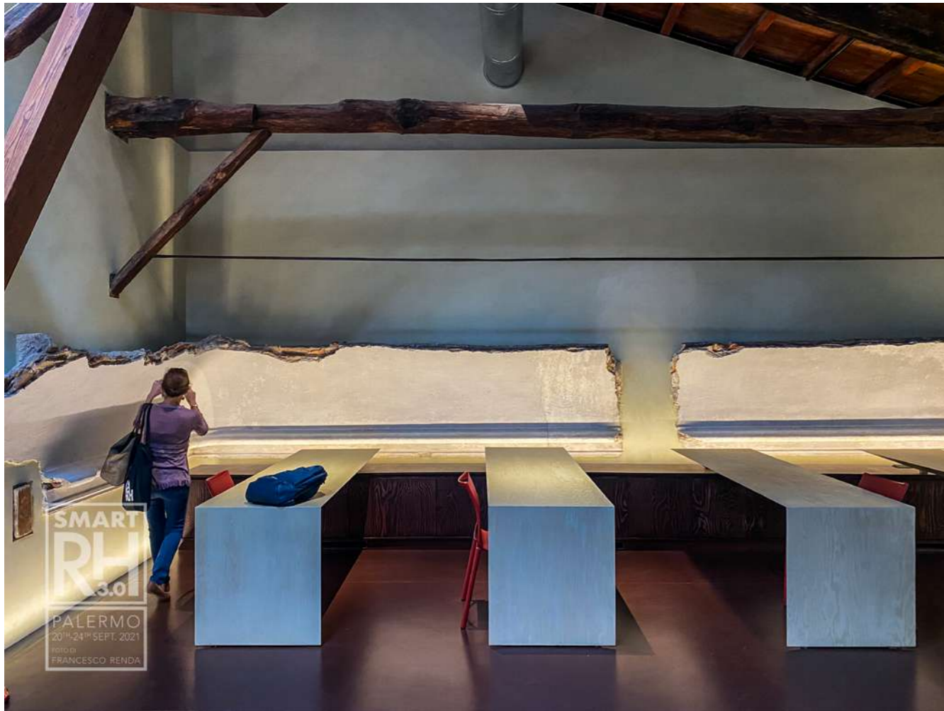
Fig.26: Restoration concept of not rebuild some timber vault's ceilings while leaving on sight the superior timbered roof. © Francesco Renda
