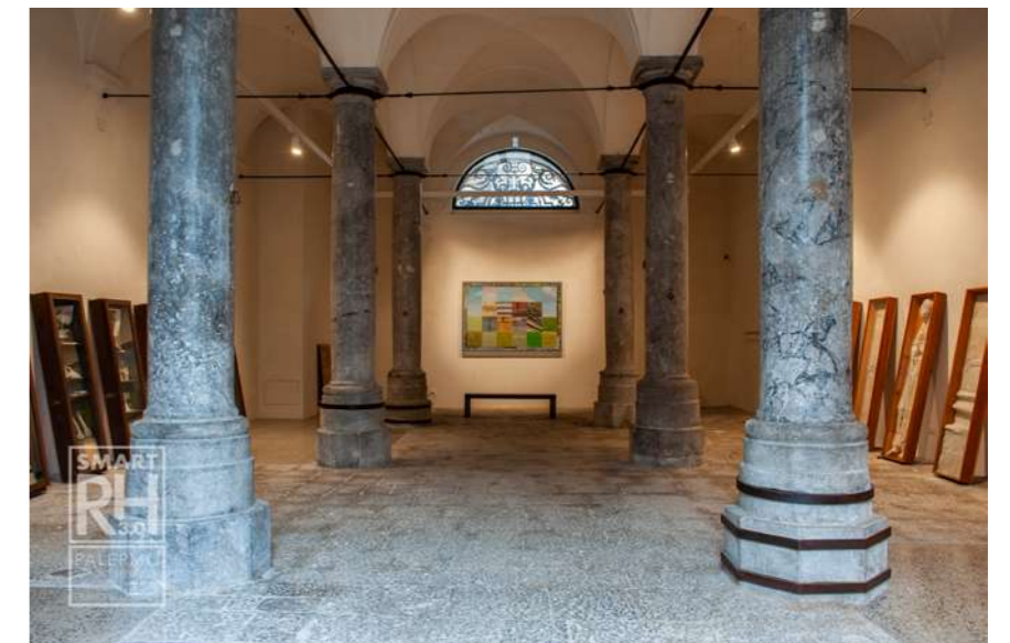
Fig.19a-b: The original stable, before and after restoration. © Project Designers & Francesco Renda
