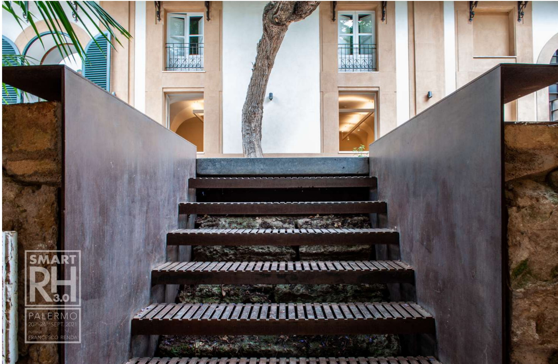
Fig.28a-b: New steel stairs and hoops in correspondence of openings. © Francesco Renda
