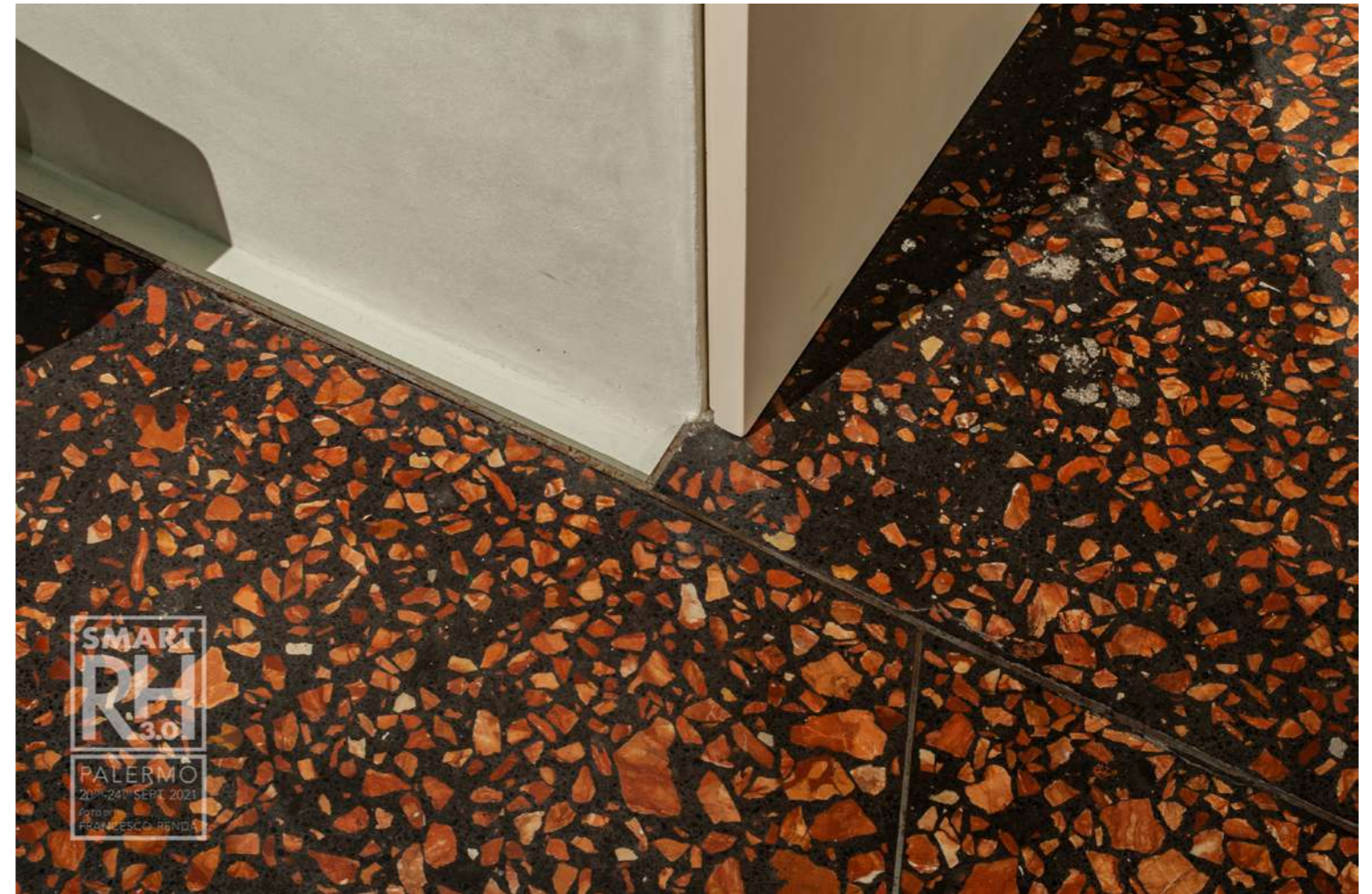
Fig.27: New paving in Venetian concrete and red marble splinters. © Francesco Renda
