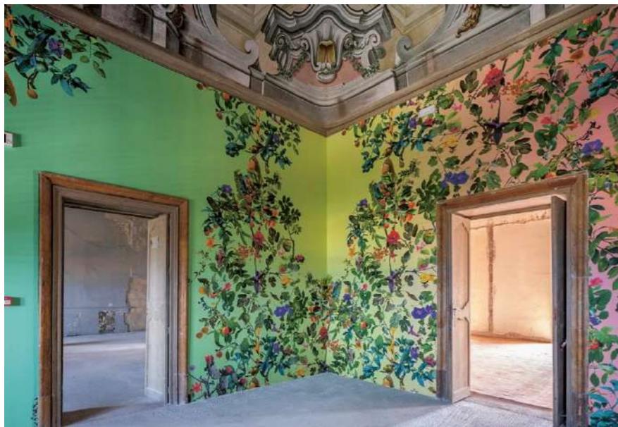
Fig.23: Manifesta 12 painting installation on walls, during the restoration works. © Project Designers
