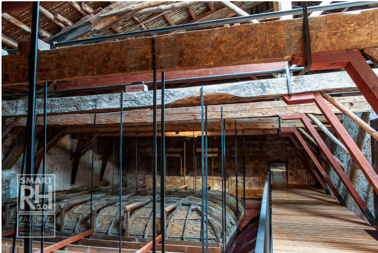
Fig.25: Restoration of wooden ceiling and trusses; structural restorations, adding new steel reinforcements. © Francesco Renda
