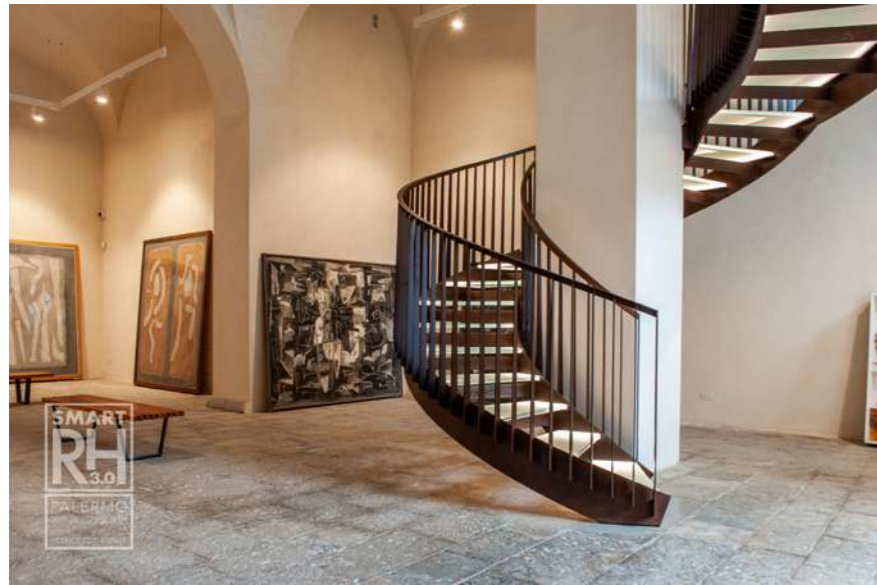
Fig.16a-b: The rooms at ground floor, hosting art collection and with the introduction of a new steel and structural glass staircase after the restoration, during the visit of Smart Rehabilitation 3.0 Erasmus+ project , Staff Training Course, happening in Palermo, September 2021. © Francesco Renda
