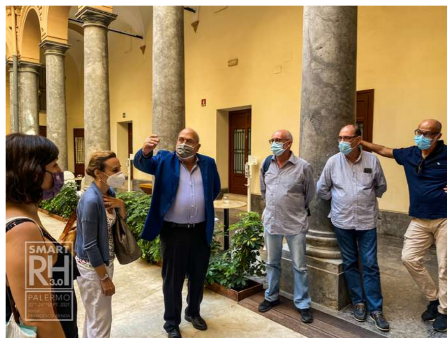
Fig.26: One of the owners, dott. Giovanni Di Giovanni, explains the general decay condition of the complex, before the restorations to the Partners and during the Staff Training Course (C6) of the EU Smart Rehabilitation 3.0 project, Palermo September 2021. ©Francesco Renda
