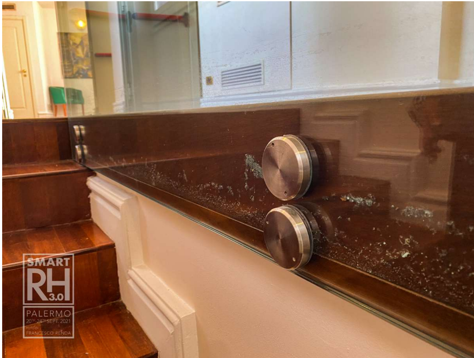
Fig.38: Tradition vs Technological Innovation details of one of the structural glass and steel parapets. ©Francesco Renda
