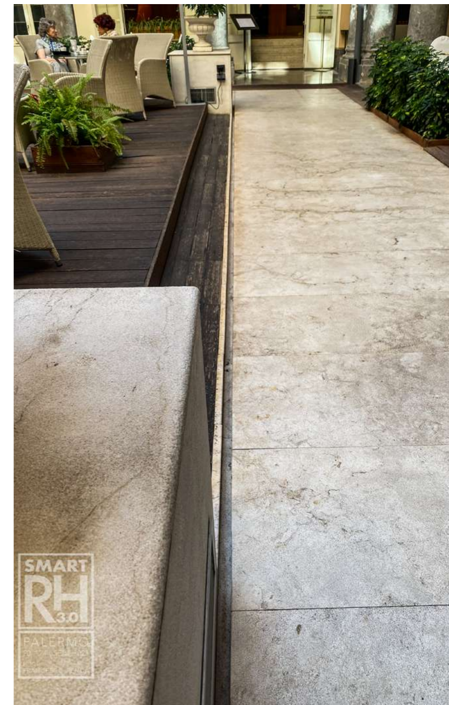
Fig.17: Permanence of compact limestone pavements enhanced by the skilful restoration project; on the left, the wooden flooring of the ancient cloister, which houses the living room at the entrance of the hotel and a conversation room. © Francesco Renda
