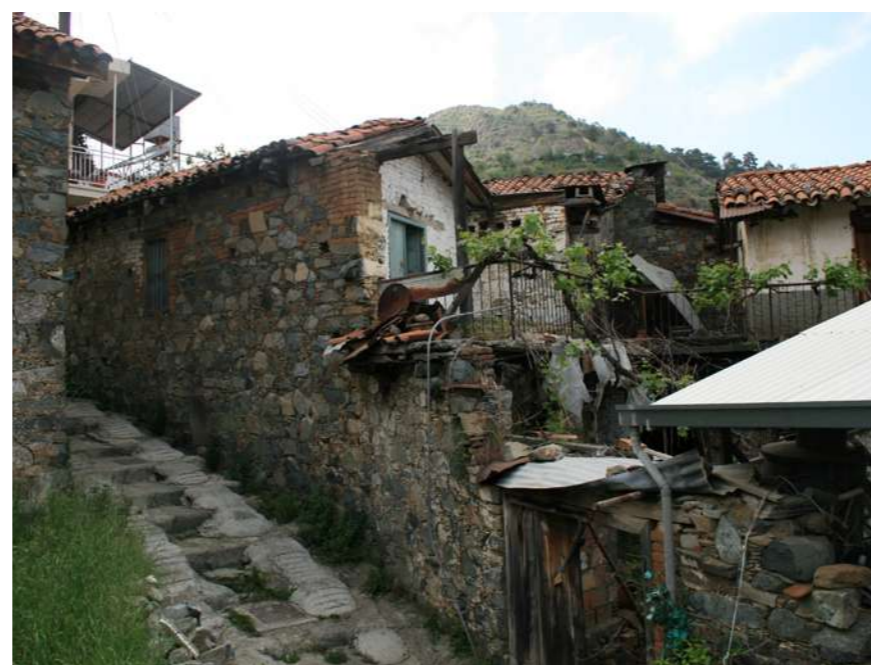
Fig.2: The house from the SE before the renovation works. © Agisilaou & Kalavas
