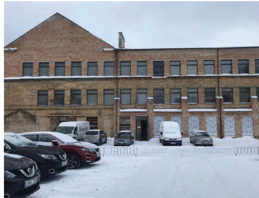
Fig.5: Yard facade before renovation.
