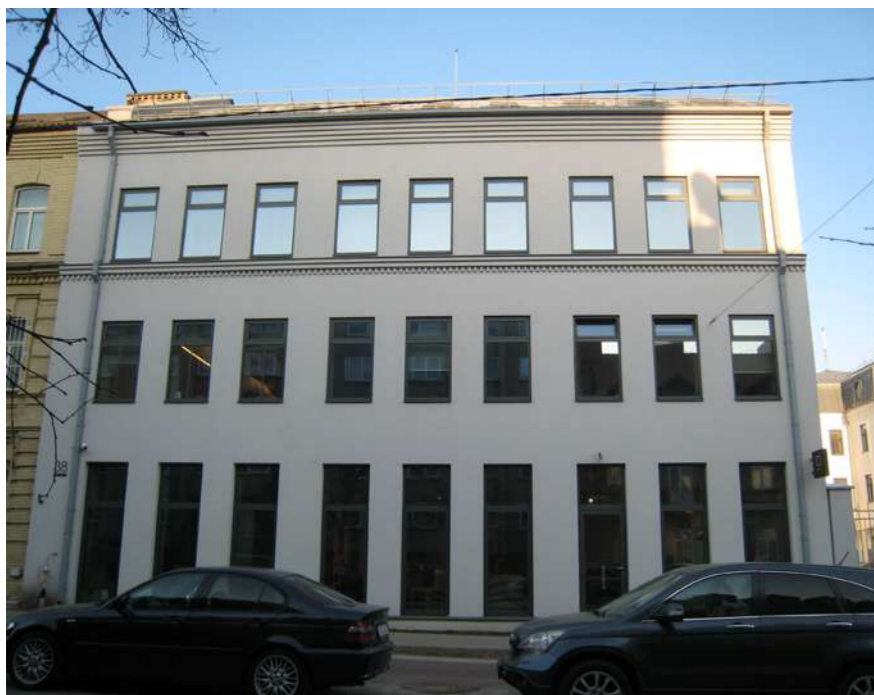
Fig.4: Street facade after renovation.
