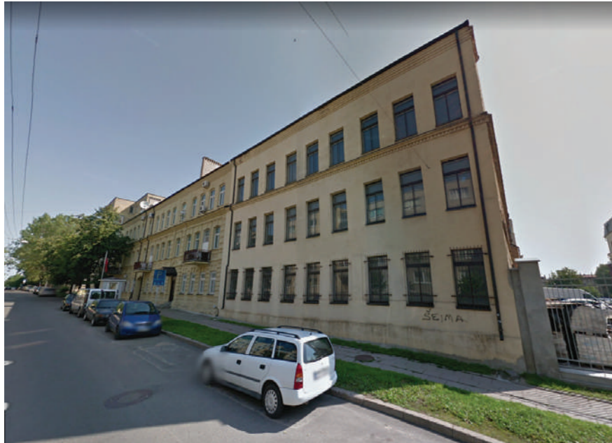
Fig.3: Street facade before renovation.
