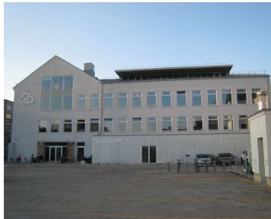
Fig.6: Yard facade after renovation.
