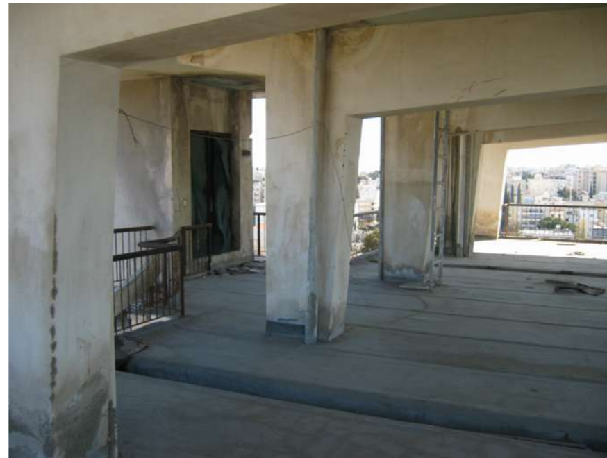
Fig.10-11: Photographs of the building before the intervention. © A. Michael's archive.
