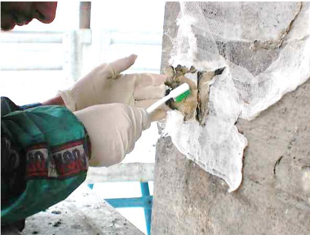
Fig.2: Restoration of the Trento Cathedral (Italy) - Consolidation of stone using compress method with very long application times. © https://www.impresedilnews.it/metodologia-bagnato-su-bagnato-per-il-restauro-delle-superfici-del-duomo-di-trento/
