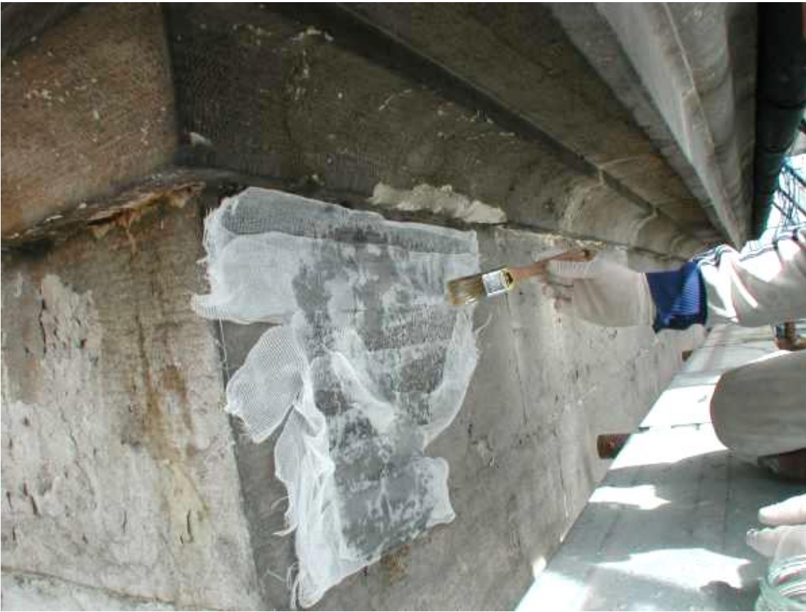
Fig.3: Restoration of the Trento Cathedral (Italy) - Consolidation Intervention of a stony cornice - the product was used to fix small and medium sized flakes and powdery parts. First, the stone was treated with acetone given by brush, in order to facilitate the penetration of the adhesive to be applied later.
