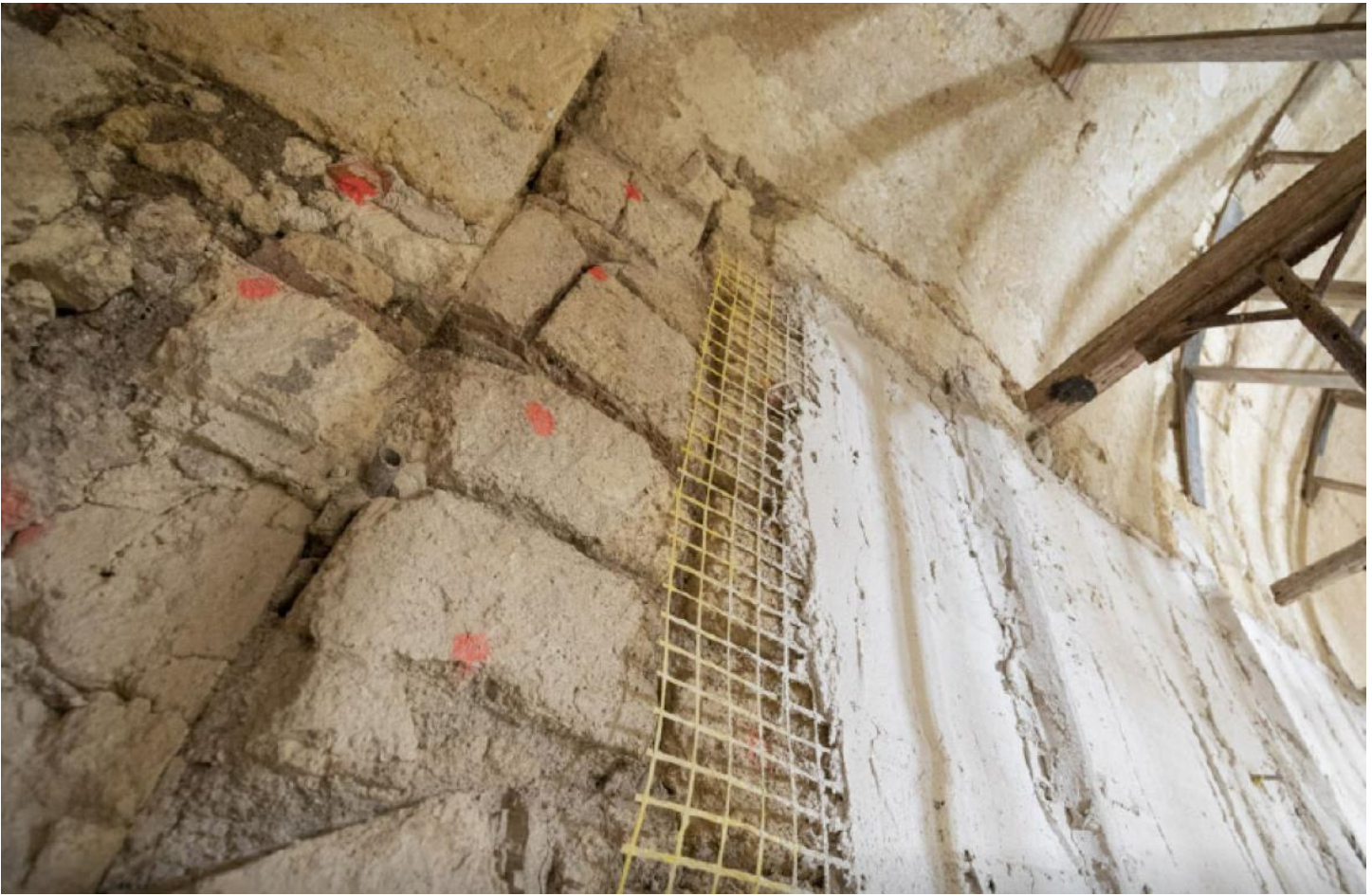
Fig.3: Application of structural concrete over fibreglass mesh. © WWW.IT.WEBER
