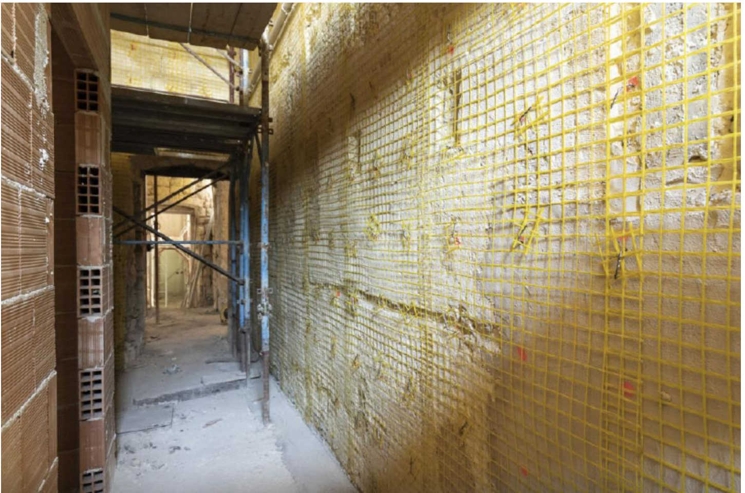
Fig.2: Saint-Gobain Weber solutions used: consolidation of the existing masonry with a thick diffusion system using webertec BTcalce F structural concrete, webertec rete250A fibreglass mesh and webertec elicafix steel bars for reinforced plaster. Restoration of the structural continuity of the masonry by injections of superfluid mortar webertec iniezione 15. New internal plasters webercalce into F finished with webercalce rasatura, both products based on hydraulic lime NHL5. © WWW.IT.WEBER
