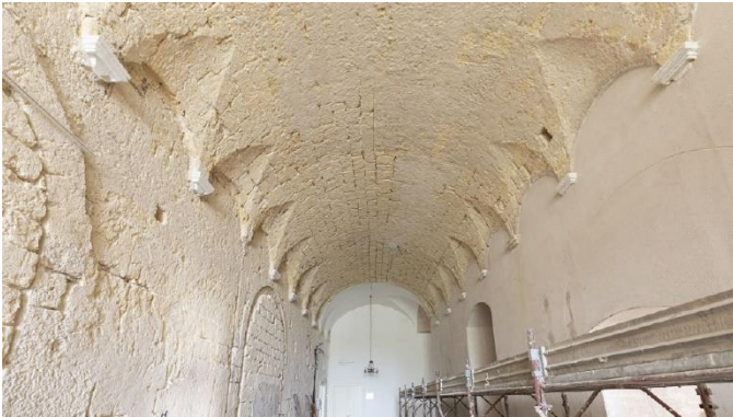
View of an interior hall with vaulted ceiling.
