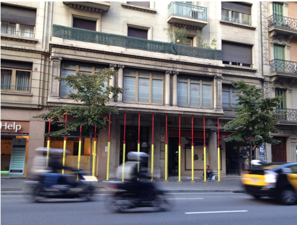
Fig.2: The shored-up gallery, prior to the start of the works. ©Xavier Falguera
