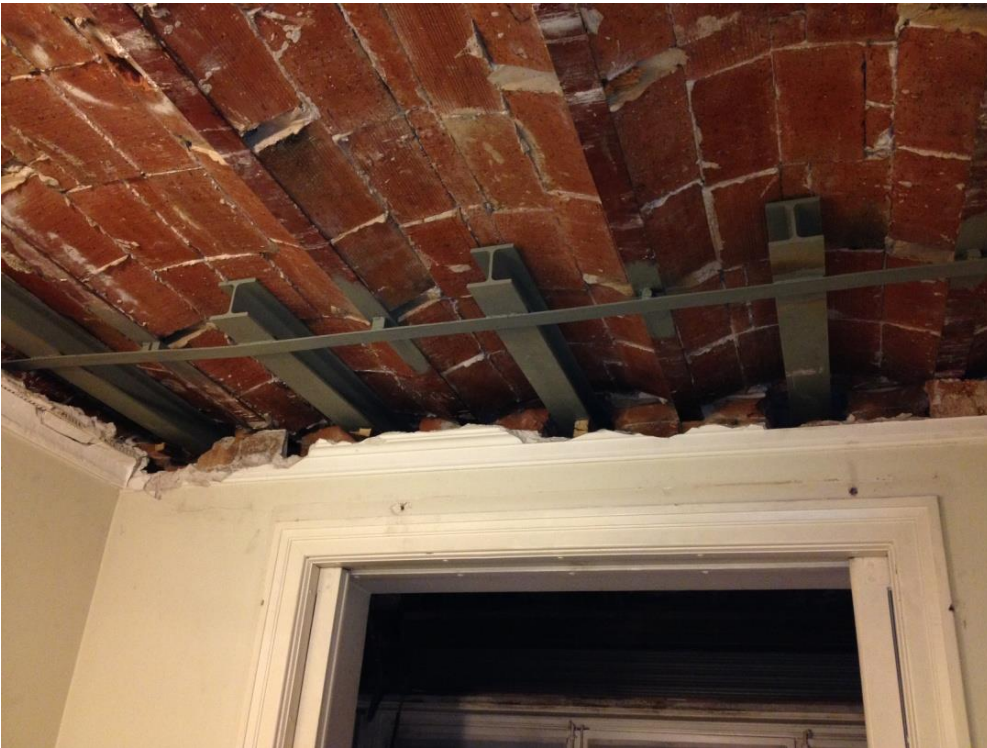
Fig.3: The new profiles, from the inside of the building, prior to the repointing of the profiles. ©Xavier Falguera
