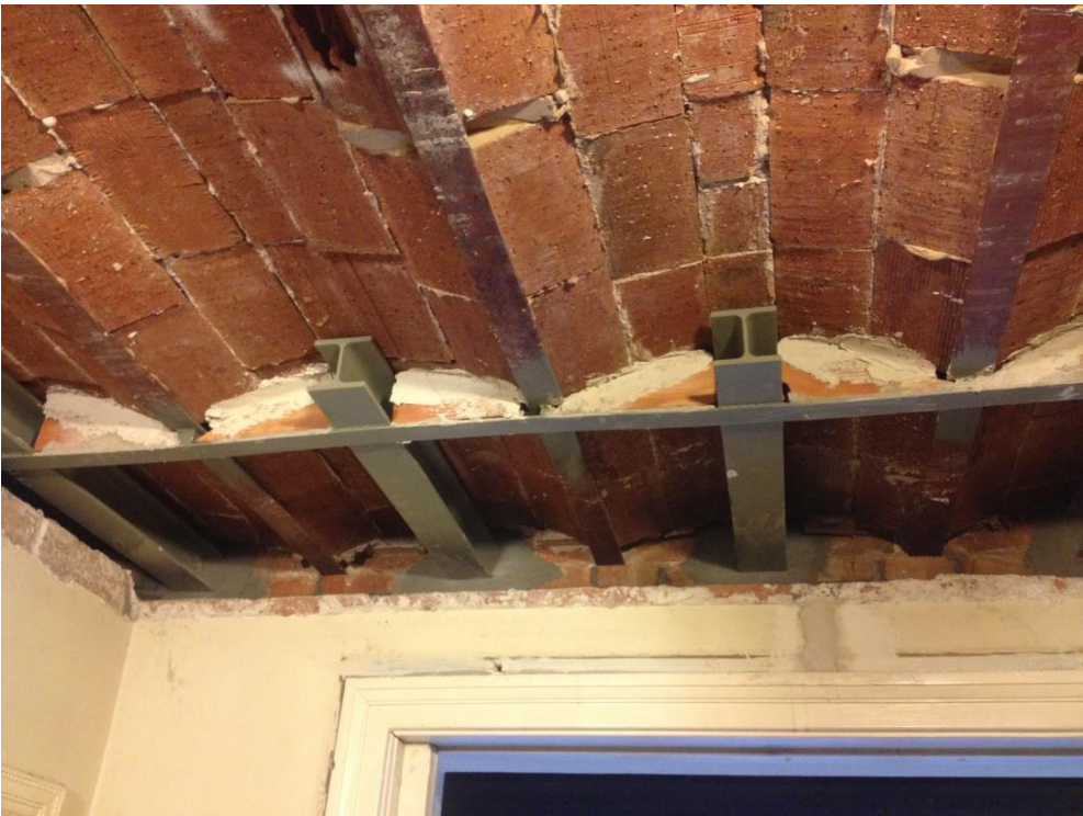
Fig.4: The new profiles, from the inside of the building, after being rejointed. ©Xavier Falguera
