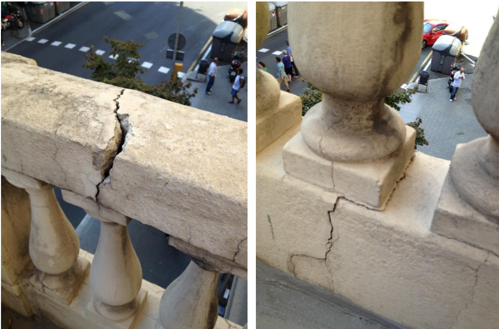
Fig.1: Damages on the railing prior to the intervention. ©Xavier Falguera
