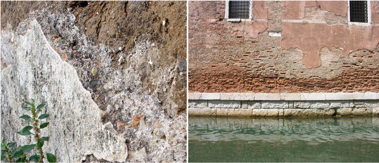
Fig.13-14: Ancient plaster based on aerial lime and cocciopesto finished in “marmorino” (fig.13). Plaster based on aerial lime and cocciopesto , walls of the Arsenale in Venice (fig.14). © https://www.quaderniquarneti.it/quaderno-4/il-cocciopesto-materia-amica.html ; https://www.quaderniquarneti.it/quaderno-4/il-cocciopesto-materia-amica.html
