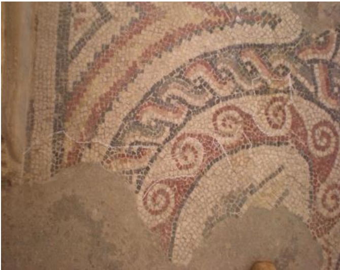
Fig.10: Mortar based on aerial lime and cocciopesto to integrate gaps in the mosaic paving (new intervention). ©Private Archive
