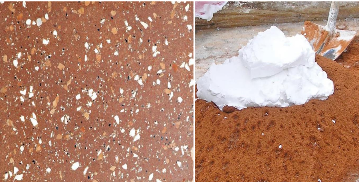
Fig.19-20: Paving realized using beaten cocciopesto with stone inserts (fig.19). Preparation on site of the mortar based on aerial lime and cocciopesto (fig.20).
