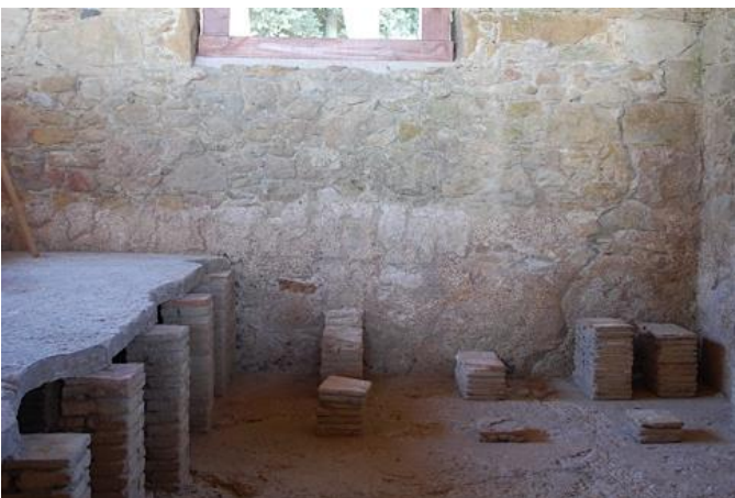
Fig.6: Mortar based on aerial lime and cocciopesto as screed for the ventilated crawl space in the Frigidarium area. ©Private Archive
