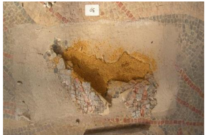
Fig.9: Fragments of cocciopesto as a transpiring filler (new intervention). ©Private Archive
