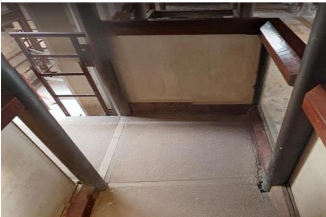
Fig.11: Mortar based on aerial lime and cocciopesto as flooring for internal paths (new intervention). ©Private Archive
