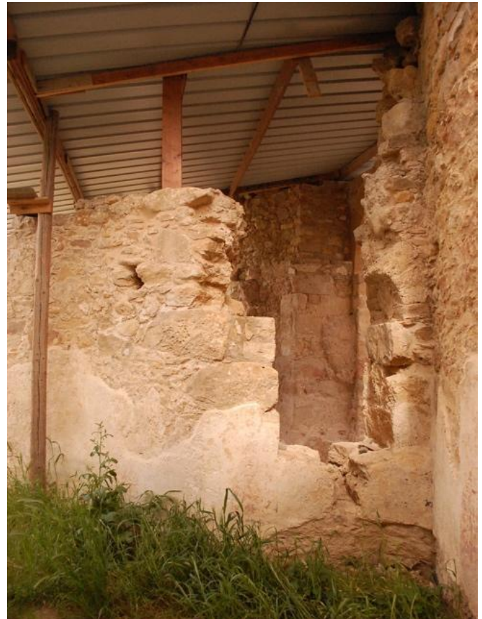
Fig.3: Mortar based on aerial lime and cocciopesto as external plaster. ©Private Archive
