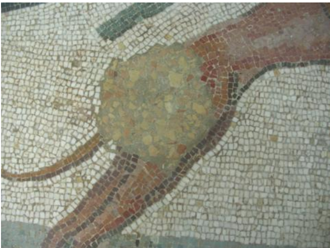
Fig.1: Mortar based on aerial lime and cocciopesto as filling a gap in the mosaic floor (previous recovery intervention). ©Private Archive
