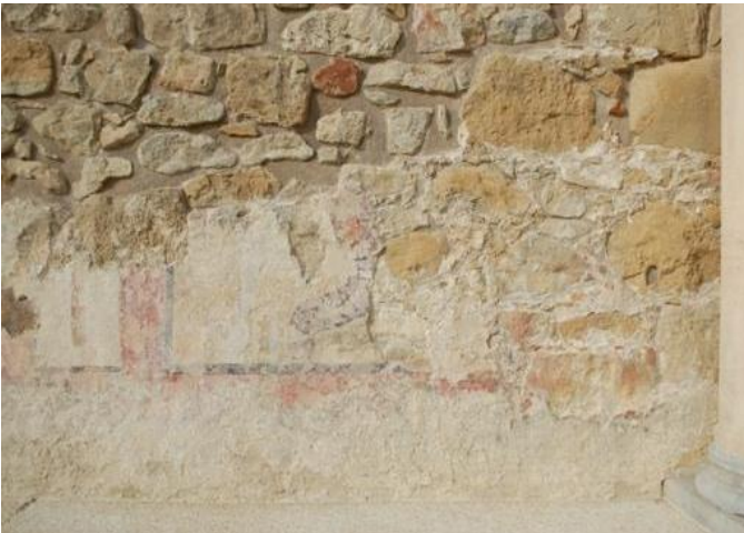
Fig.4: Mortar based on aerial lime and cocciopesto as internal plaster and support of the wall painting.
