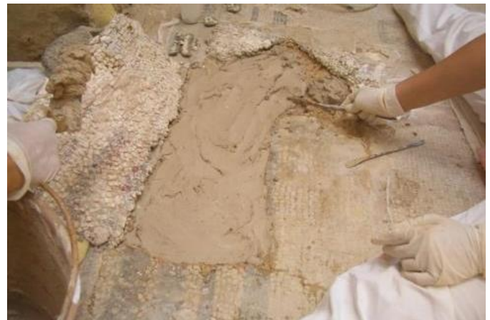
Fig.8: Laying of mortar based on aerial lime and fine-grained cocciopesto as a sediment of the mosaic floor to be relocated. ©Private Archive
