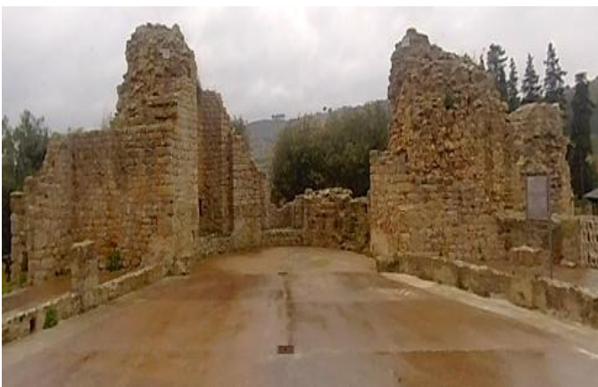
Fig.12: Mortar based on aerial lime and cocciopesto as external flooring (new intervention). ©Private Archive
