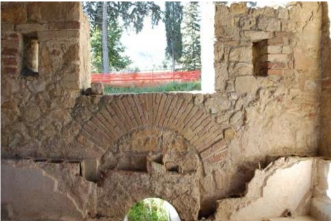
Fig.5: Mortar based on aerial lime and cocciopesto as internal plaster of the Frigidarium area. ©Private Archive
