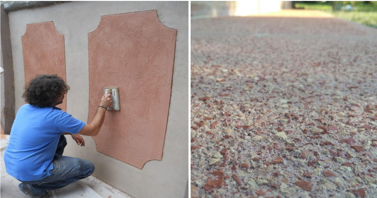
Fig.17-18: Spreading plaster based on aerial lime and cocciopesto using a trowel (fig.17). Background screed with less finely ground cocciopesto (fig.18).
