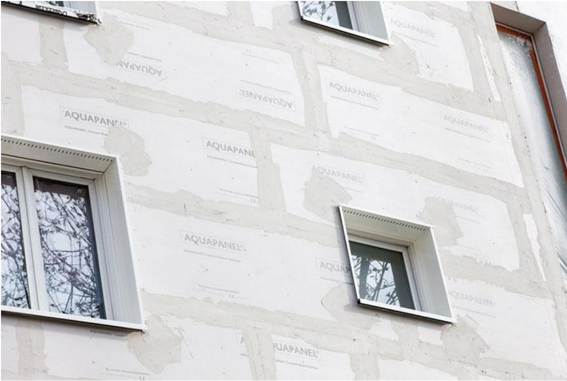
Fig.1: Aqua panel outdoor. © https://www.commercialeisonzo.it/knauf/aquapanel/
