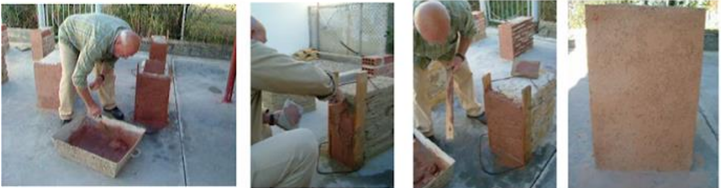
Fig.3: An outline of the process of preparing the hydraulic plaster with the addition of ceramic dust. ©Maria Philokyprou
