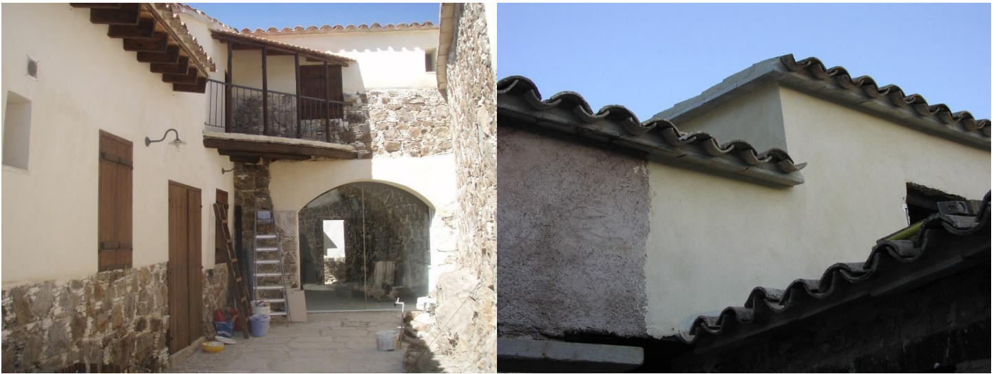
Fig.1-2: Application of hydraulic plaster on a rural dwelling in Kapedes. ©Maria Philokyprou
